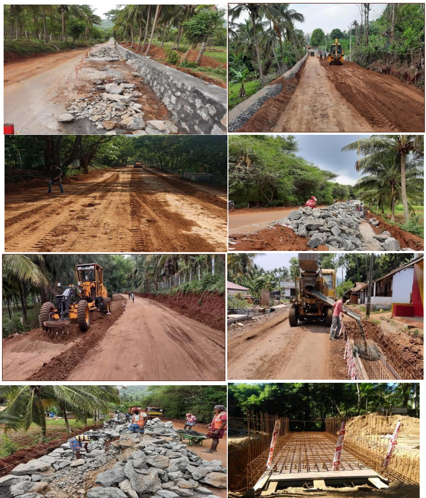
Retaining Wall, Culvert, Side Drain and Road Works are in Progress
