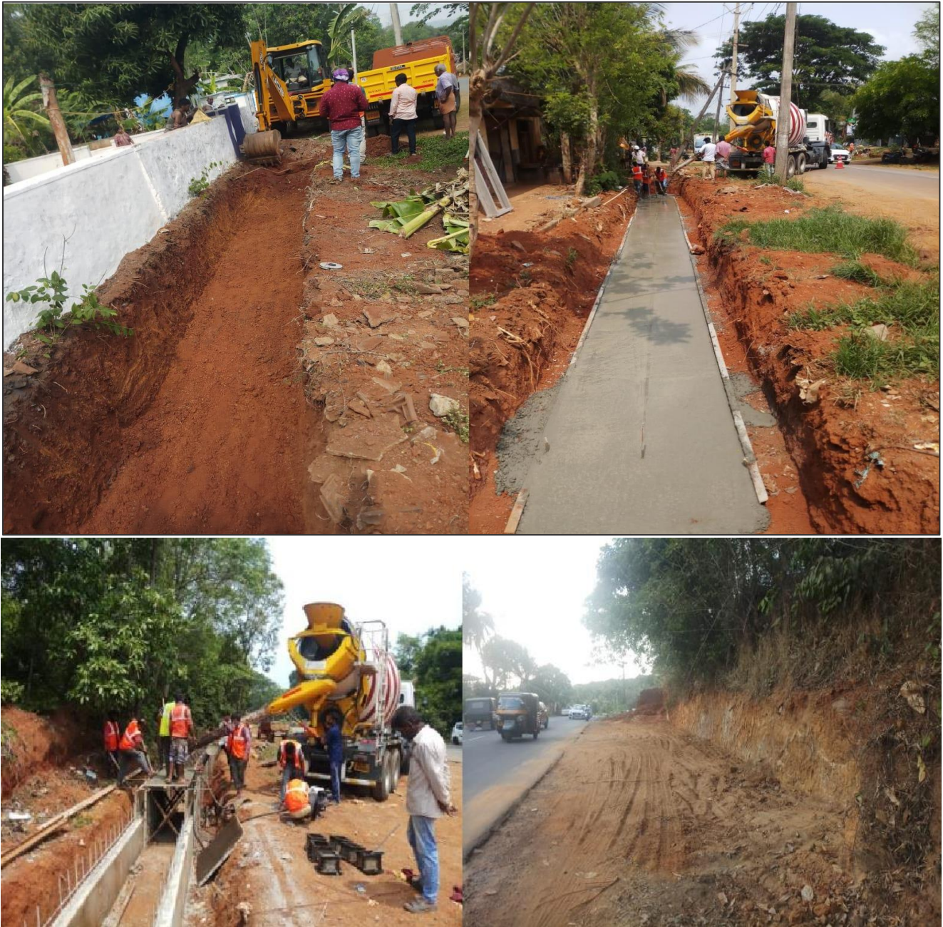
Drain works in progress
