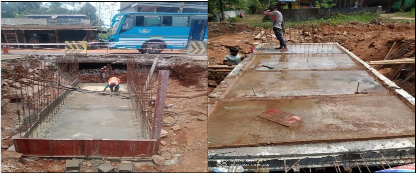
Culvert Work In Progress
