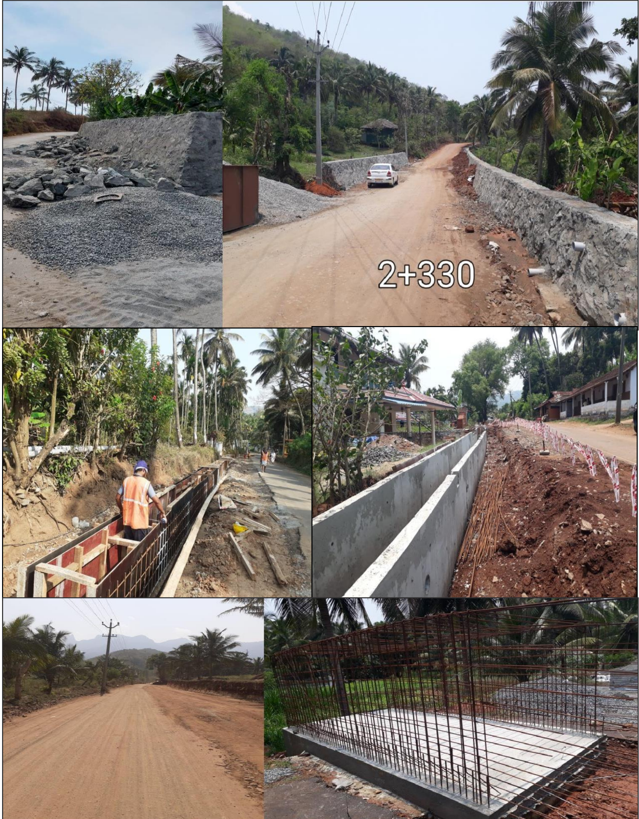
Retaining Wall, Side drain, Culvert and Road Works are in progress
