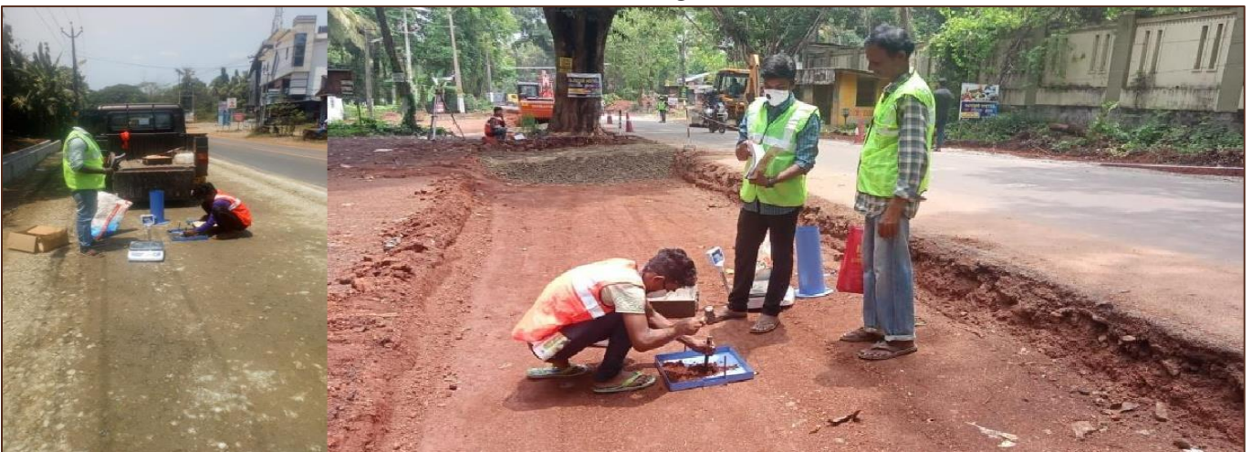
Road Work In Progress
