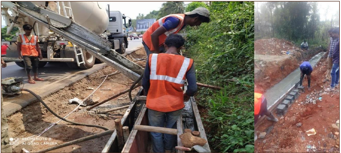
Side Drain Work In Progress
