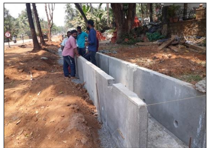
3.8Kms RCC Pre-cast Drain casted and erection in progress
