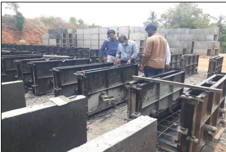
3.8Kms RCC Pre-cast Drain casted and erection in progress
