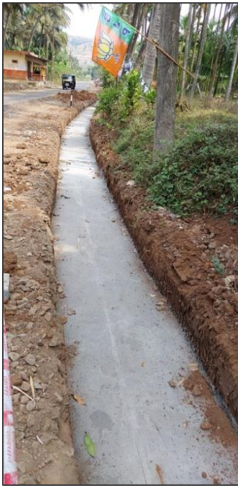
Side Drain Works in Progress
