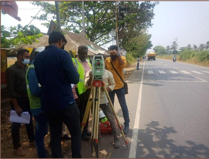
PMC Team visited RKI 09 on 1 st Mar'2021 and conducted Site inventory Survey
