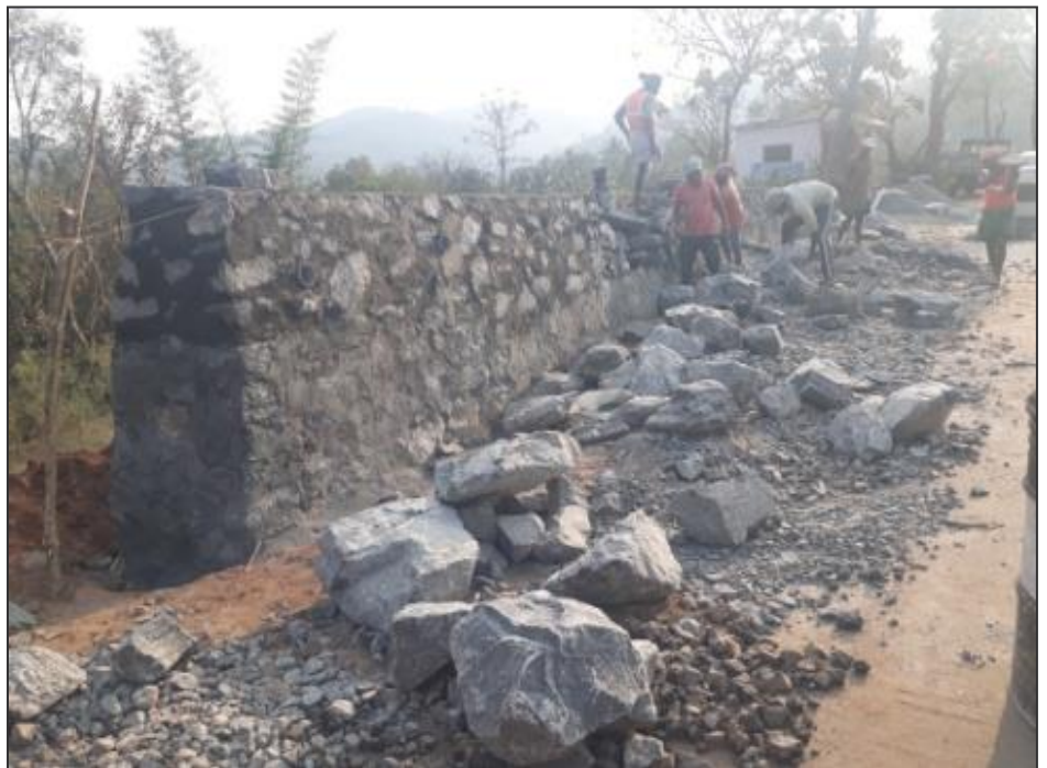
Retaining Wall works in Progress
