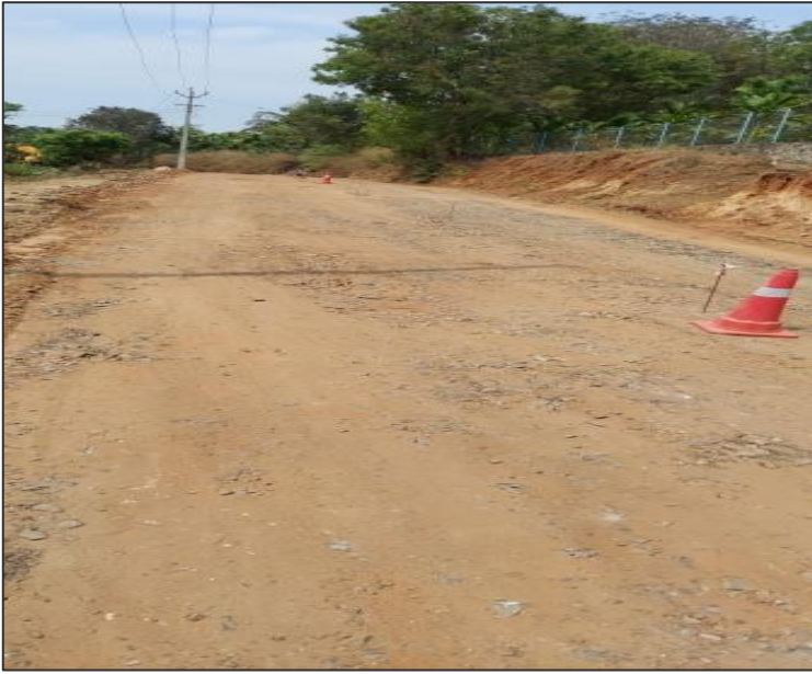
Road Excavation Works in progress
