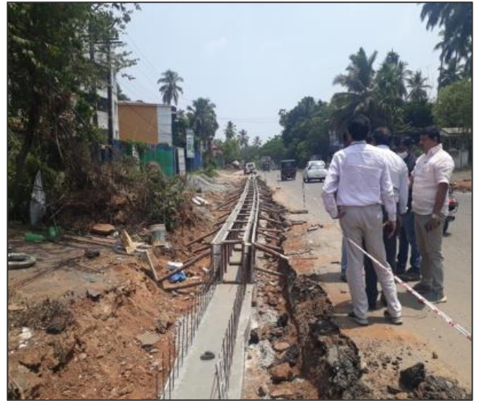
Side Drain Works in Progress
