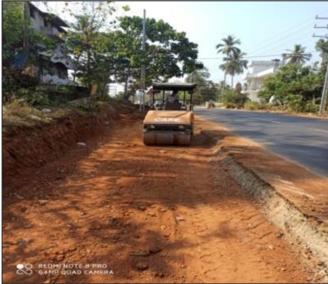
Road Excavation in progress
