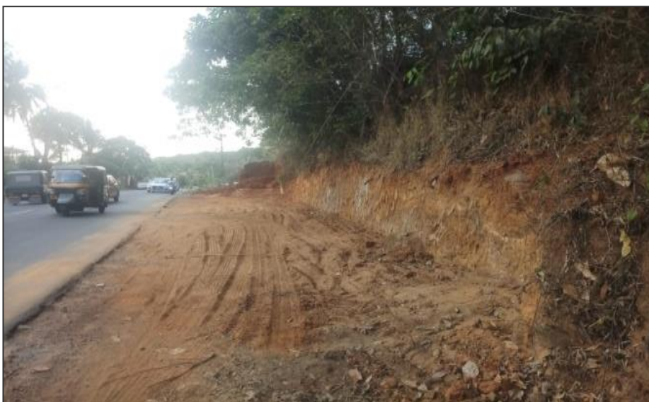
Road excavation Works in progress
