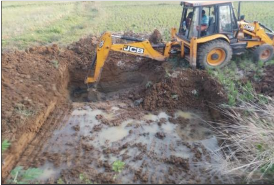
Culvert Widening Works in progress
