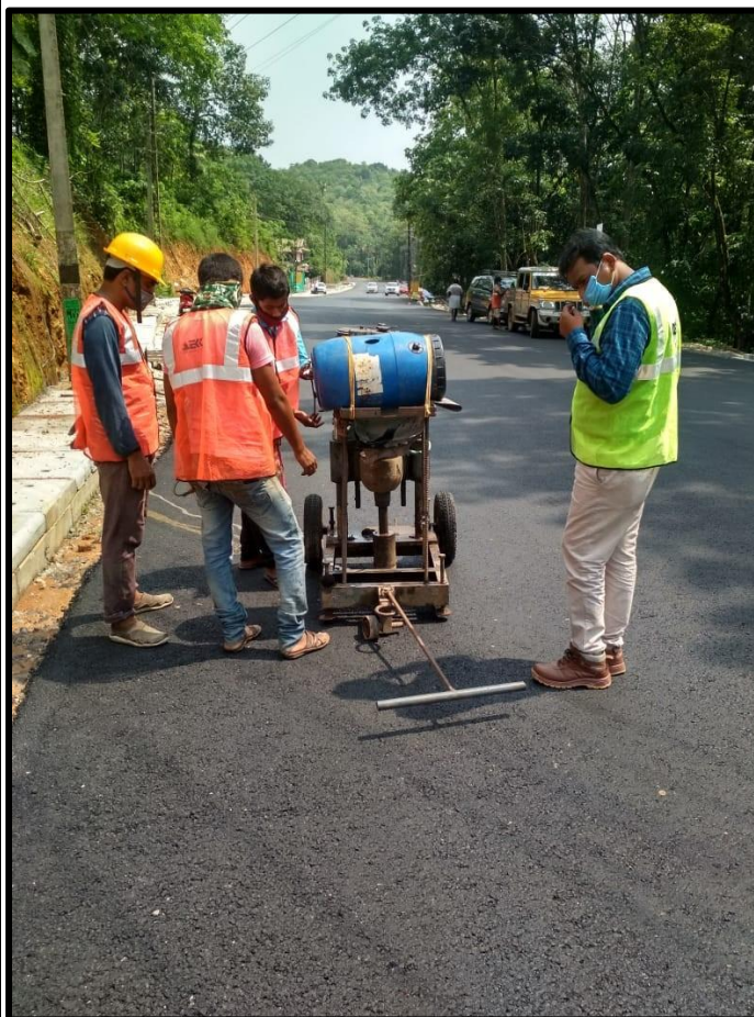
Core cutting work in progress
