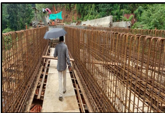
Kootupuzha Bridge Span P2-P3 Girder reinforcement works
