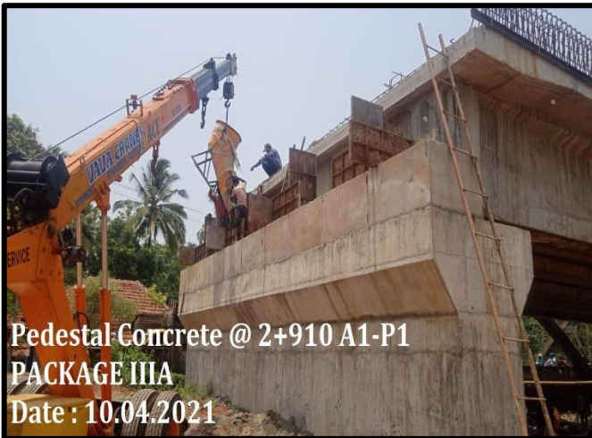
Pedestal Concrete @ 2+910 P1
