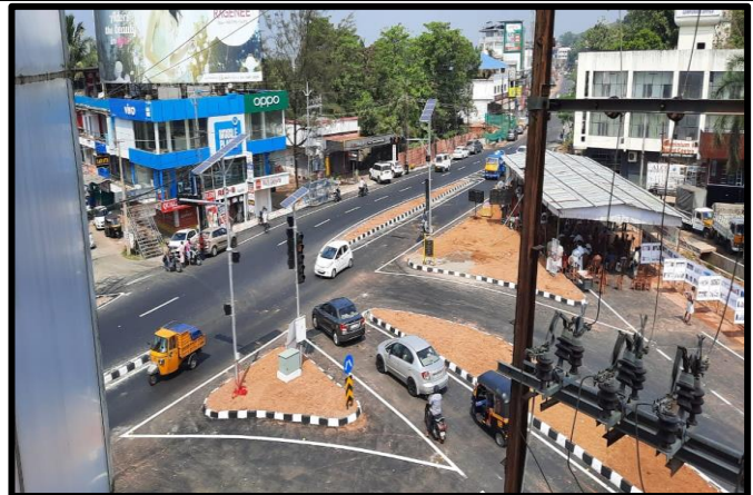
Km:2+300, Ramanchira Junction
