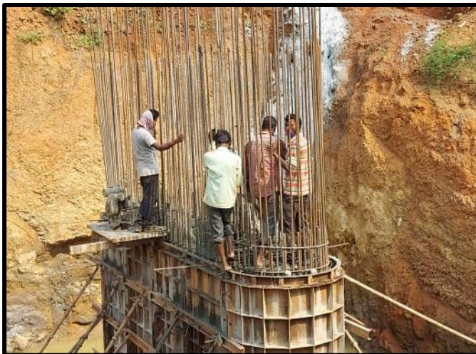
Kootupuzha Bridge Pier P4 01 st lift concreting
