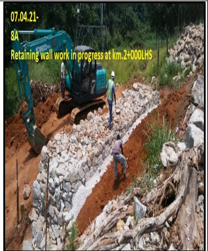
Retaining wall work in progress
