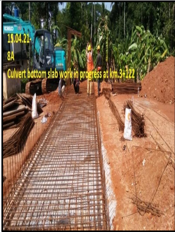
Culvert Bottom slab work in progress
