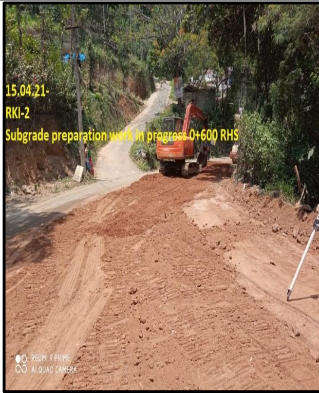
Subgrade work in progress
