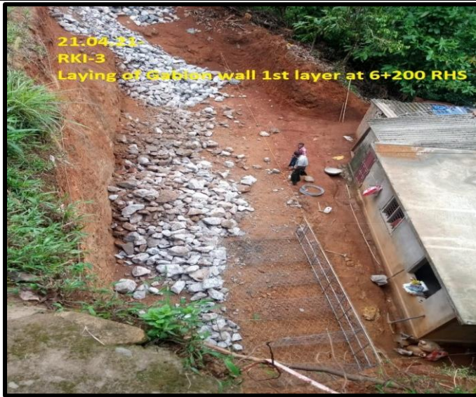
Laying of Gabion wall 1 st layer at 6+200
