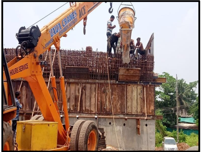
Pedestal Concrete @ 2+910 A1
