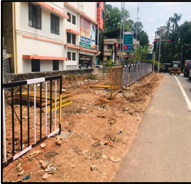
Hand rail work to protect Extra Land at 1+600,RHS
