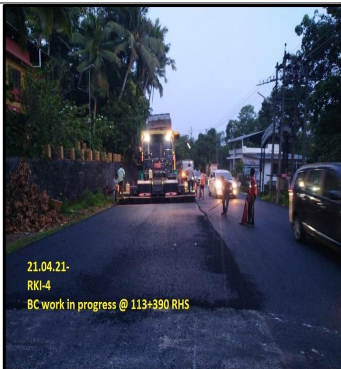
BC work in progress
