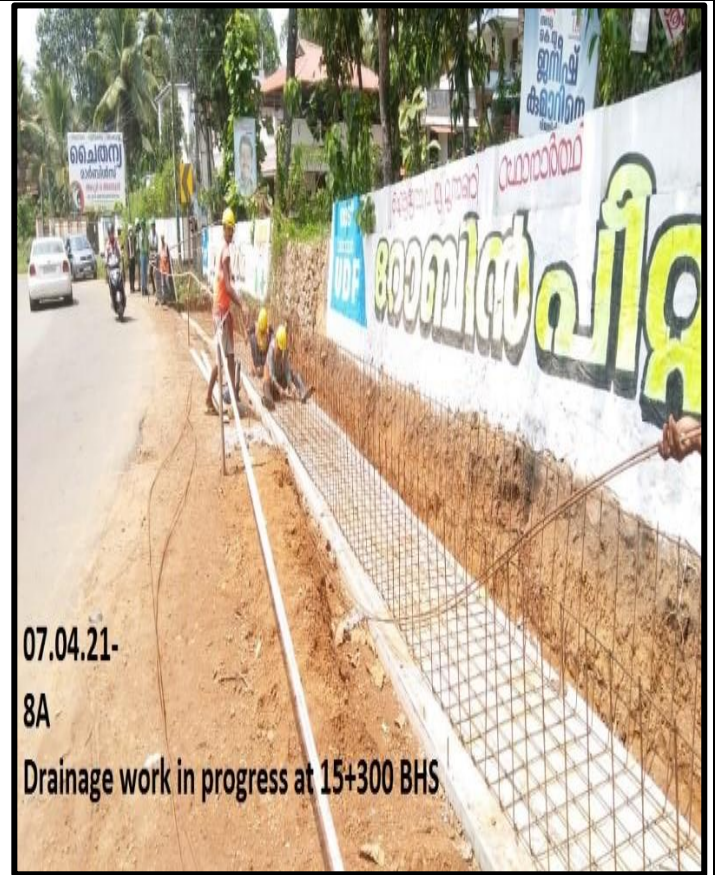
Drain work in progress
