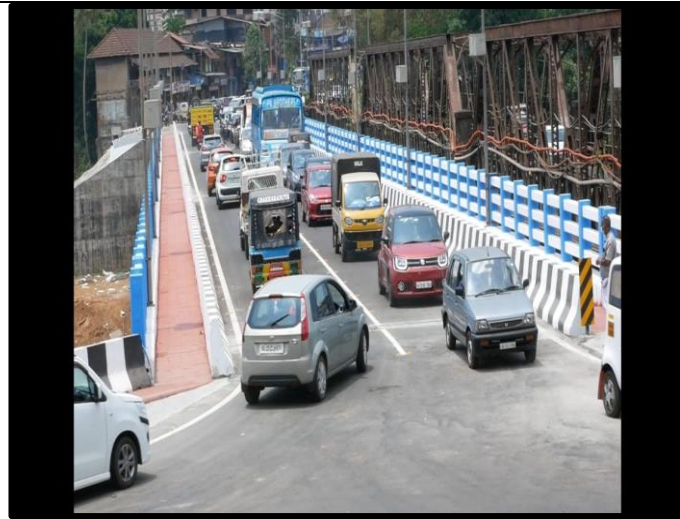
Irritty Bridge at km 42+198 opened for traffic
