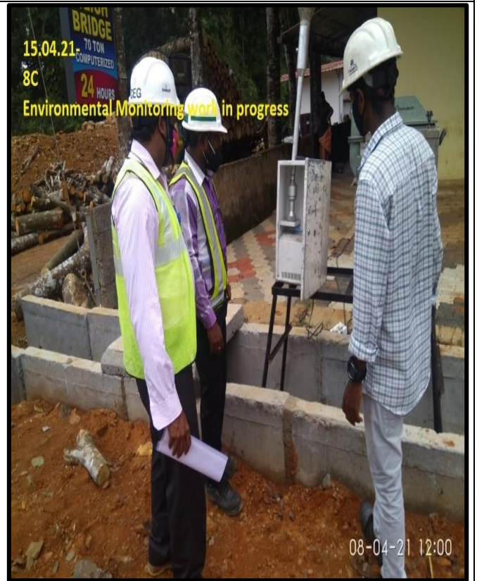
Environmental monitoring work in progress
