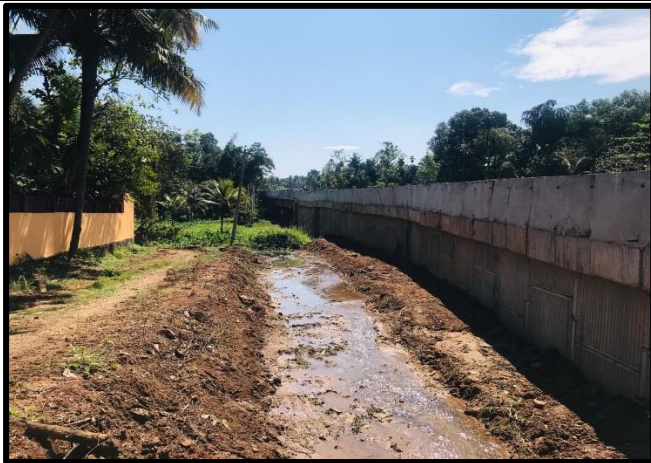
Canal Cleaning work On RHS
