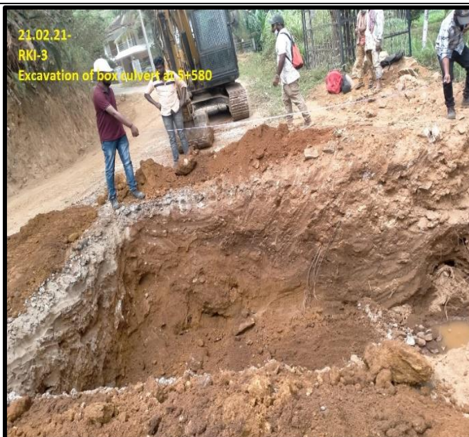
Box culvert Excavation work in progress
