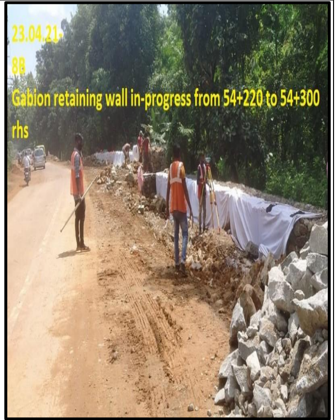
Gabion wall work in progress
