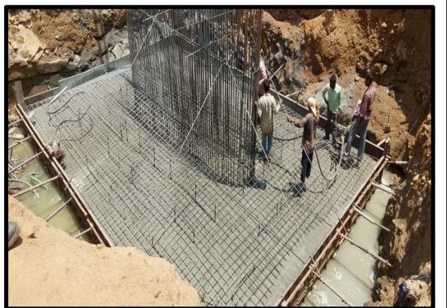
Kootupuzha Bridge Pier P4 Raft concreting
