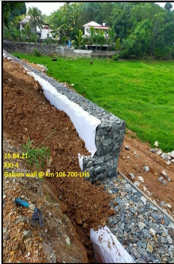
Gabion wall work in progress
