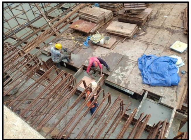
Kootupuzha Bridge Pier P2 (for span P2-P3) pedestal
