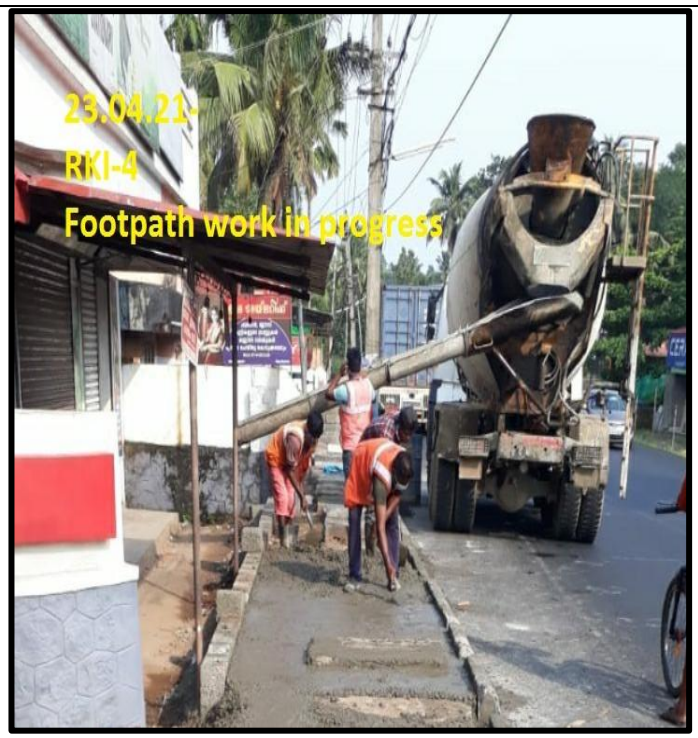
Footpath work in progress
