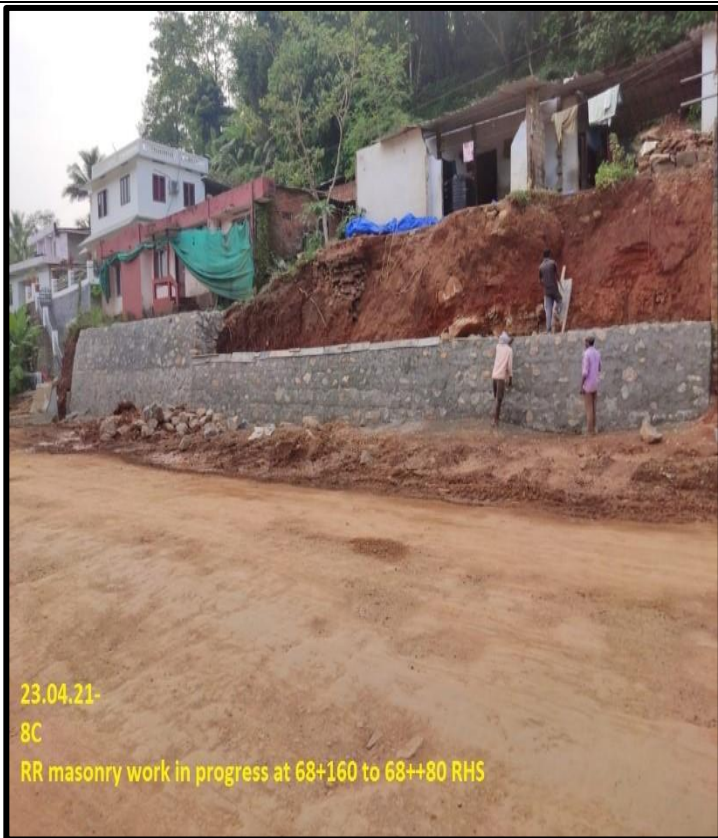
RR Masonry work in progress
