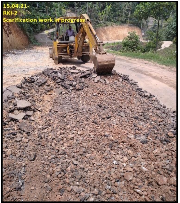
Scarification work in progress
