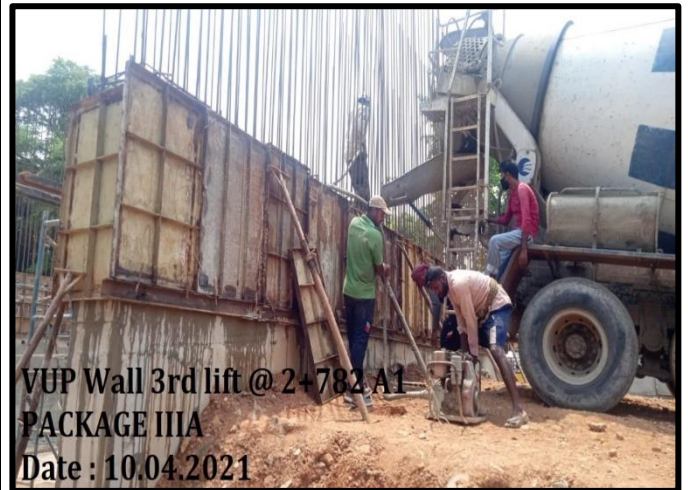
VUP Wall 3 rd lift Concrete @ 2+782 A1 Side
