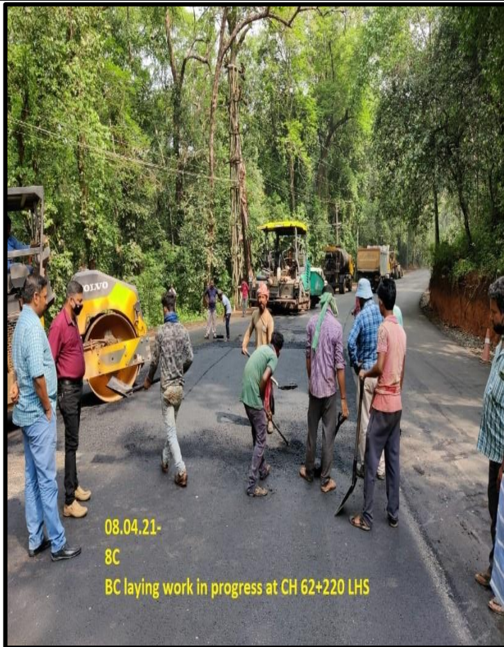
BC Laying work in progress
