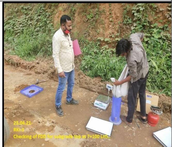
FDD Checking in progress
