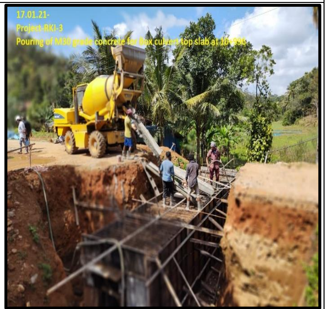
Box culvert concreting work in progress
