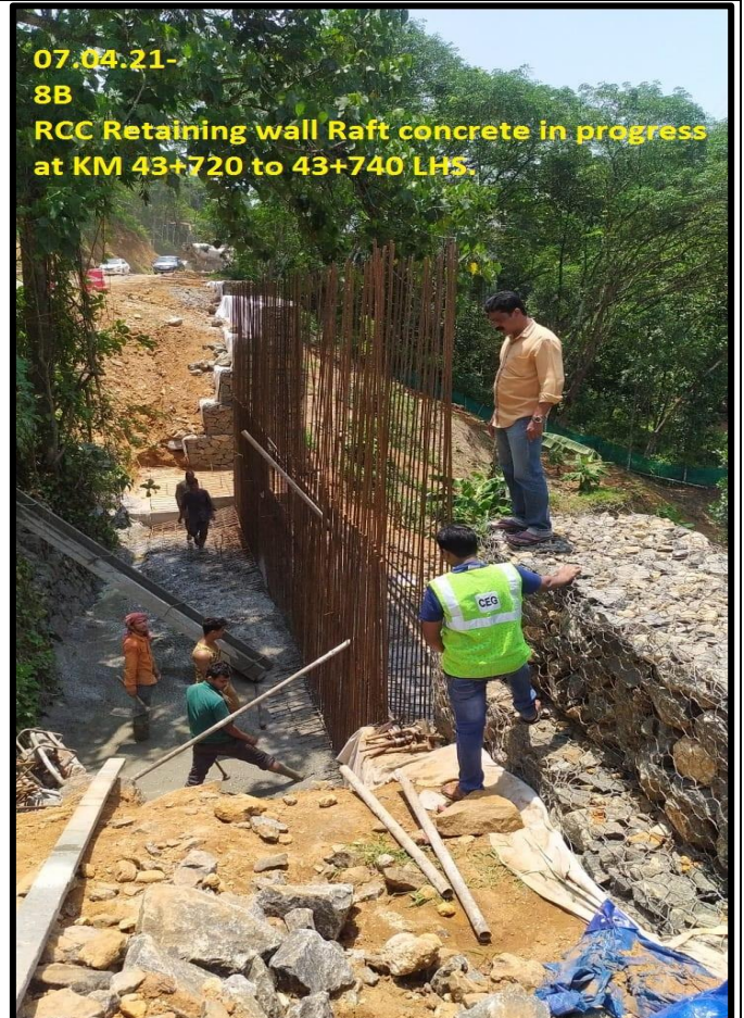
Retaining wall raft work in progress
