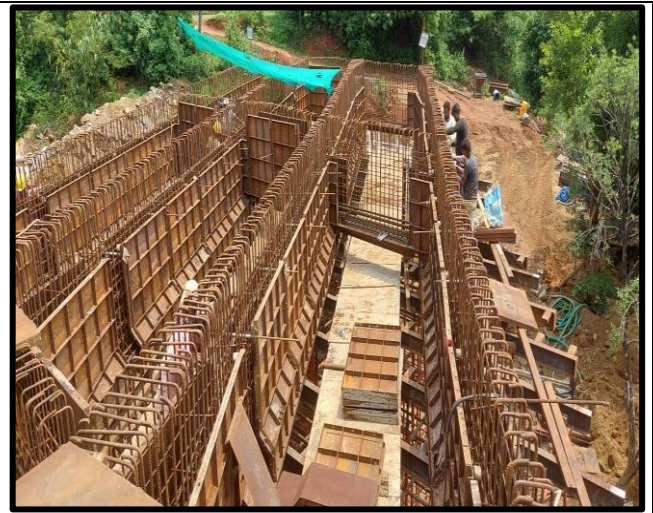
Kootupuzha Bridge Span P2-P3 shuttering works.
