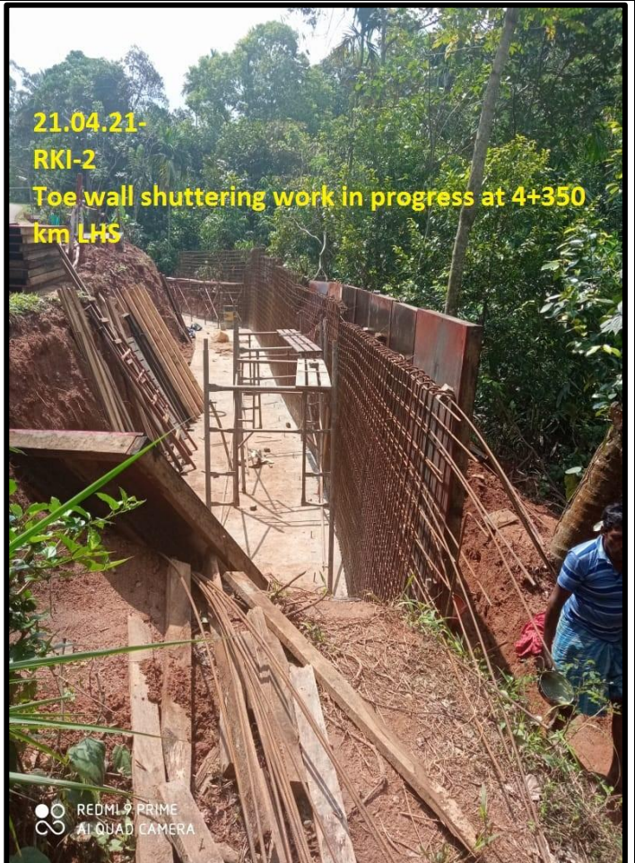
Toe wall work in progress
