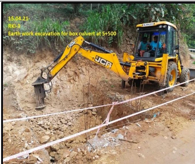
Box culvert excavation work in progress
