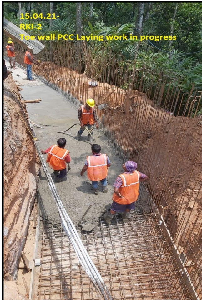
Toe wall PCC Laying work in progress
