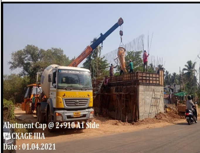
Abutment Cap @ 2+910 A1 Side
