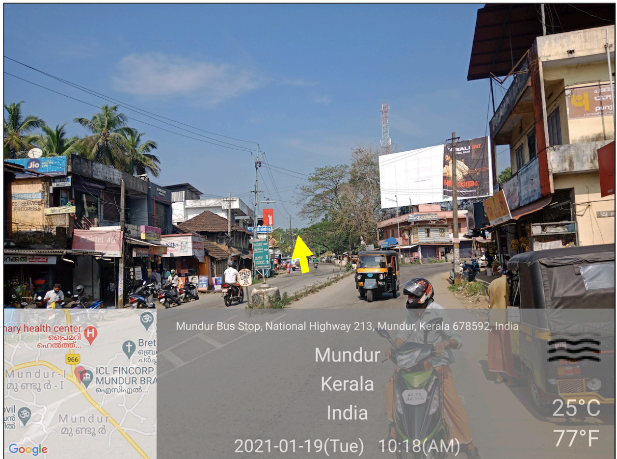
Start Chainage of Project Road at Mundur Junction (Arrow mark showing the direction of the road)
