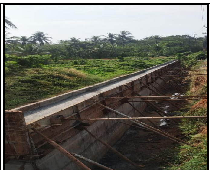
Retaining Wall 3 rd lift Completed @ Ch: 23+150 – 23+180 RHS
