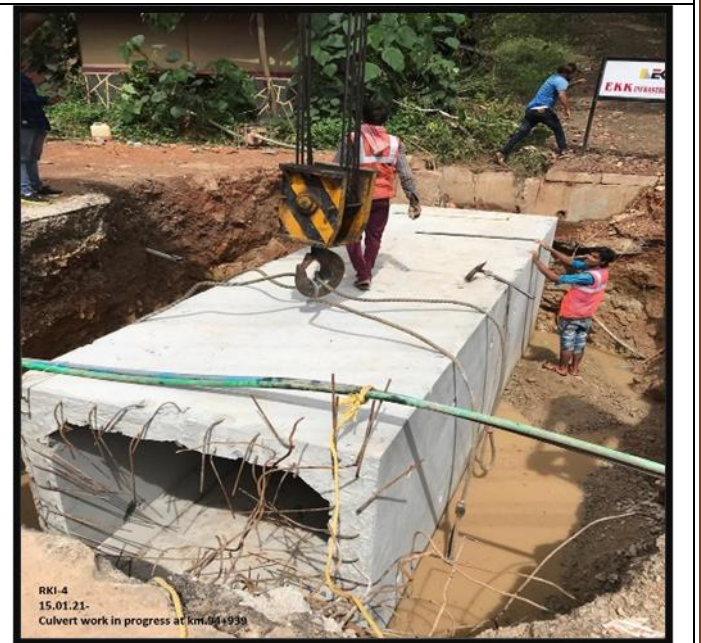
Box culvert work in progress
