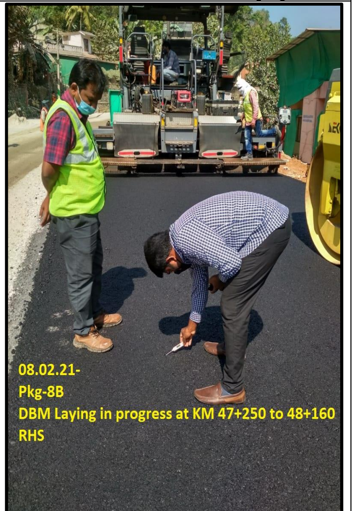
DBM Laying in progress at km.47+250 to 48+160
