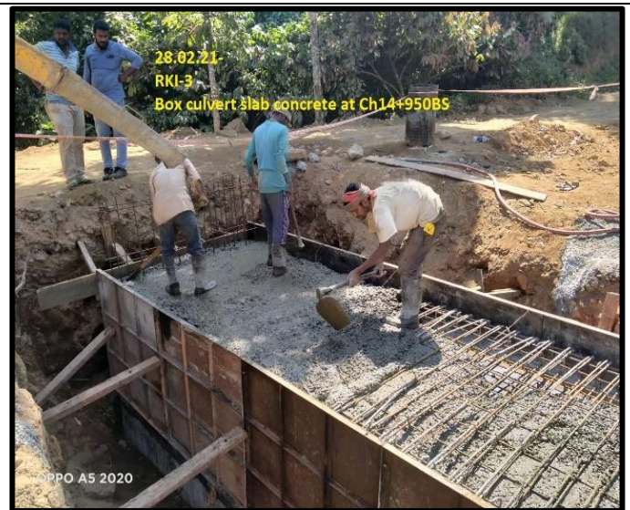
Box culverts slab concrete in progress
