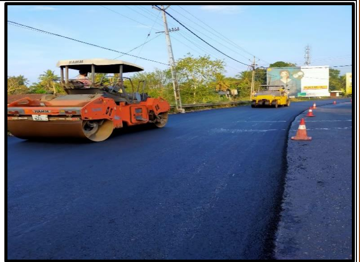
BC overlay work in progress
