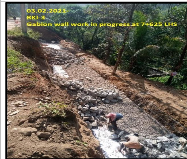
Gabion wall work in progress at km.7+625
