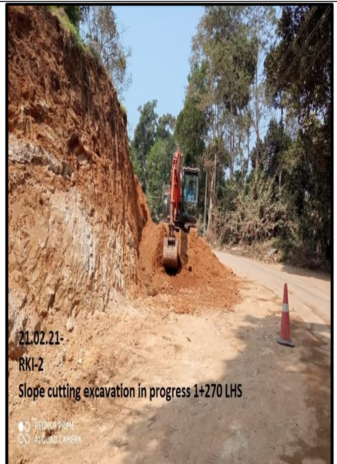
Slope cutting excavation in progress at km.1+270 LHS
