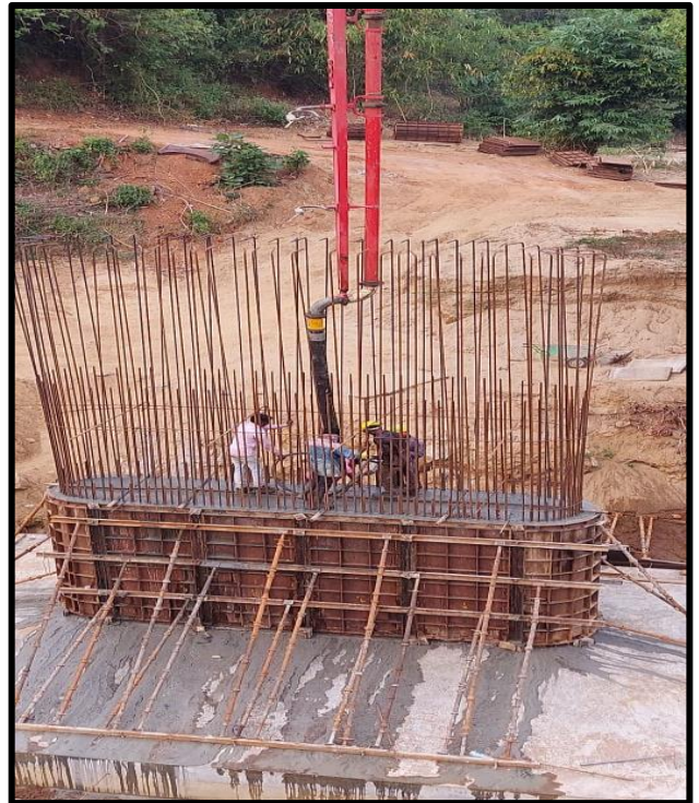
Kootupuzha Bridge Pier P3 01 st lift completed.
