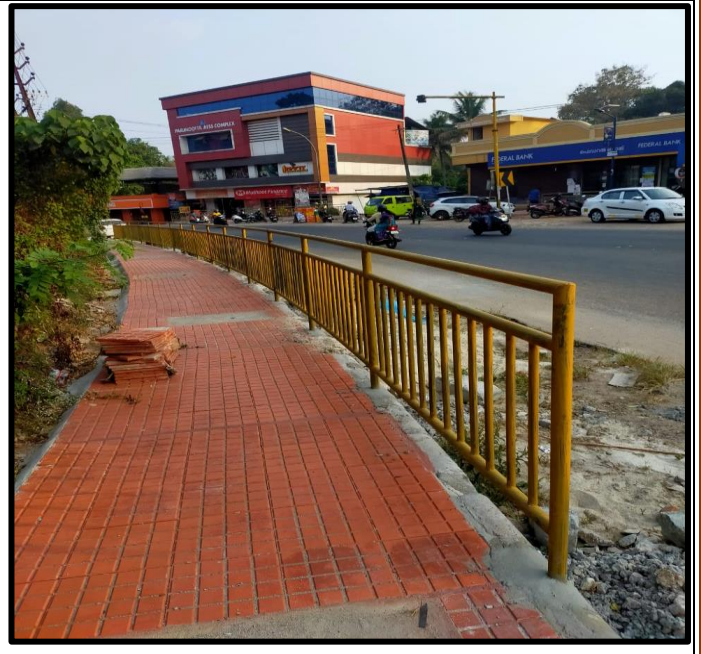
Foot Path laying work in progress
