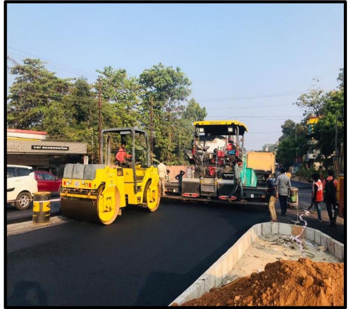
BC Laying work on 2+300. Ramanchira Junction
