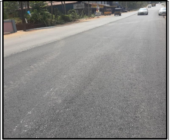
BC Laying @ Ch: 26+165 – 26+290 LHS
