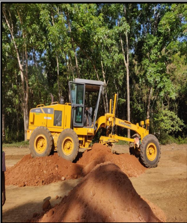
Embankment work in progress at km.15+00
