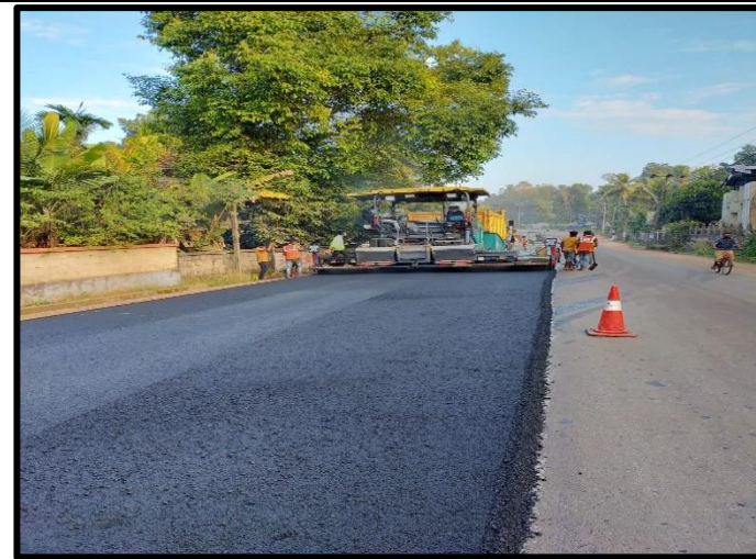
BC overlay work in progress
