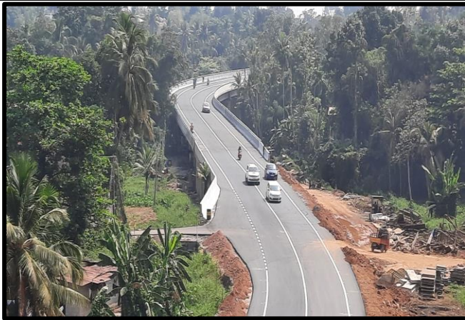
Road work completed for Thiruvalla Bypass
