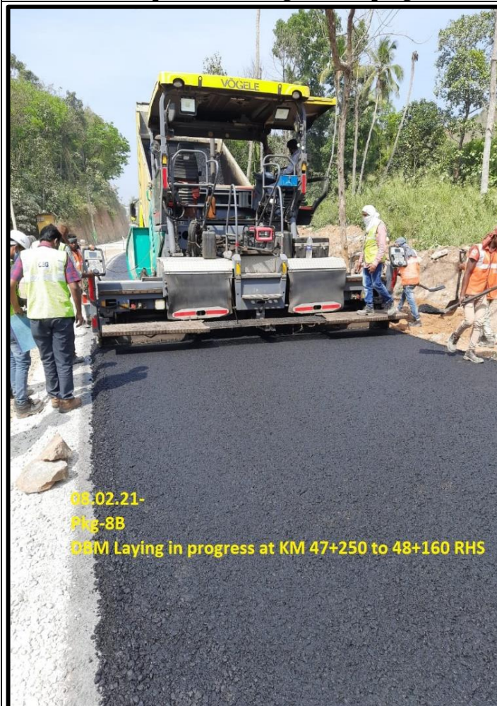
DBM Laying in progress at km.47+250 to 48+160
