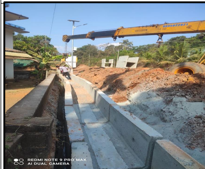
Drain Laying @ 28+817 – 28+837 LHS
