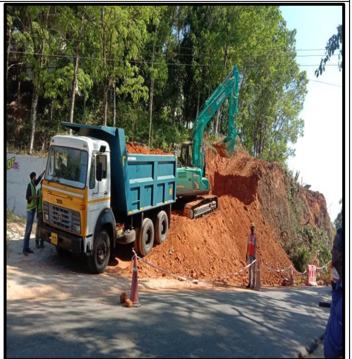
Excavation work in progress at km.2+450
