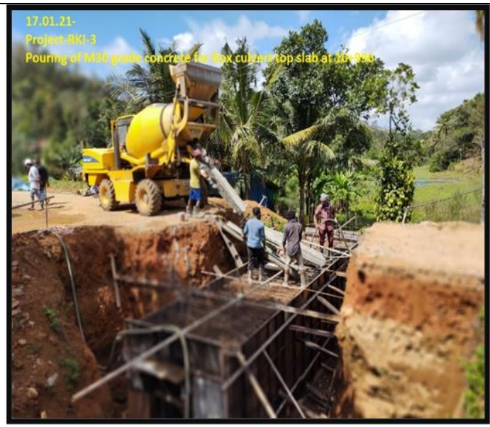
Box culvert concreting work in progress
