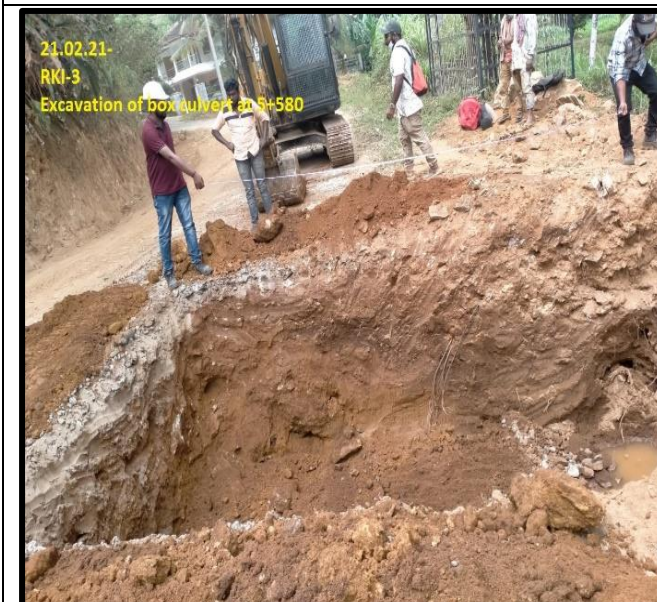
Box culvert Excavation work in progress
