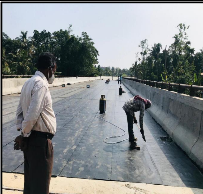
Poly propaline sheet fixing over deck slab of Viaduct
