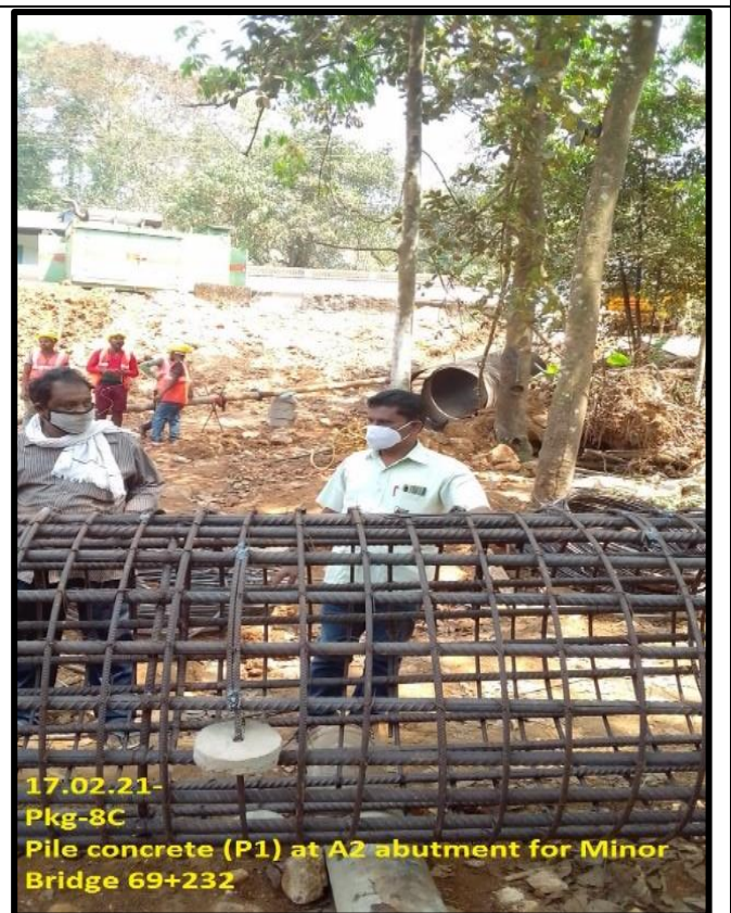
Pile reinforcement work in progress
