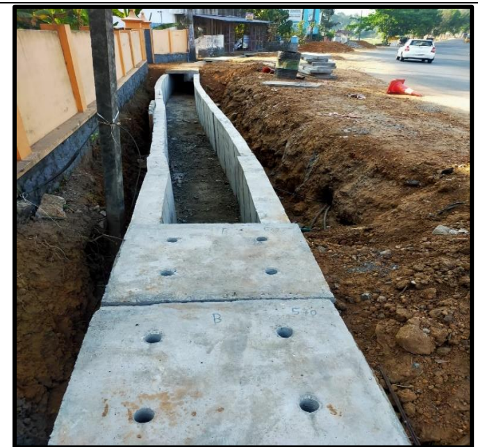
Drain Laying work in progress
