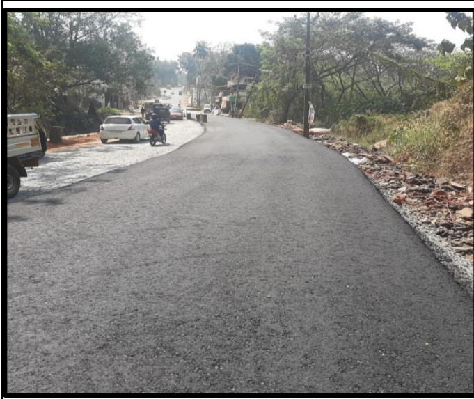
DBM Laying @ Ch: 26+260 – 26+370 LHS
