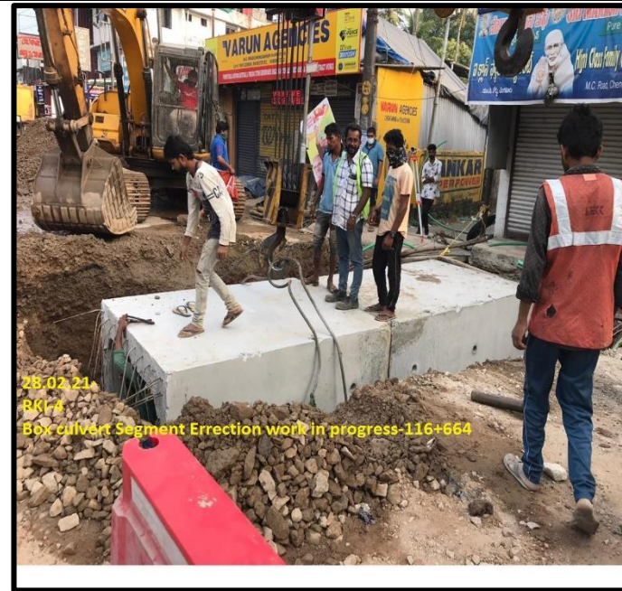
Precast box culvert work in progress
