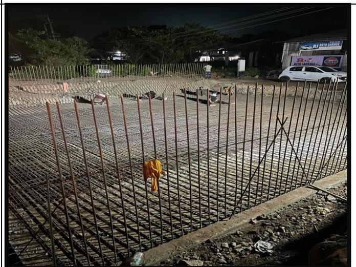
**REINFORCEMENT WORK IN PROGRESS FOR RAFT @ 3+000 VUP**
