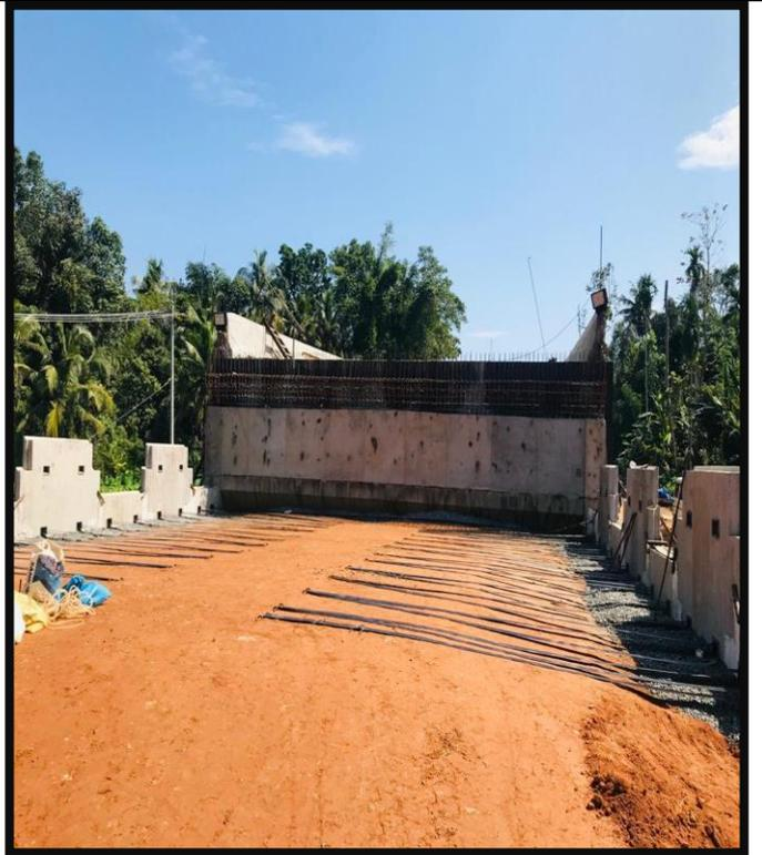
**Embankment filling work at A2 side approach of Viaduct.**
