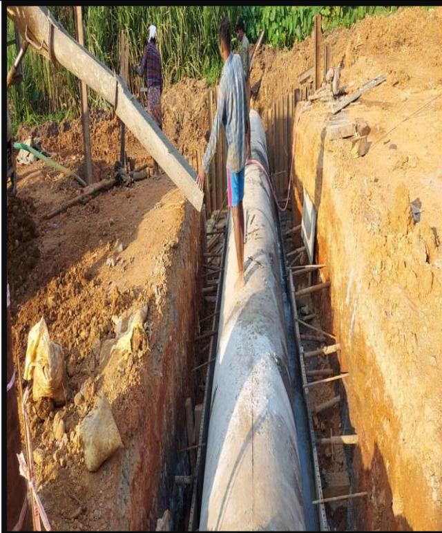
**Pipe culvert concreting works at 2+185**
