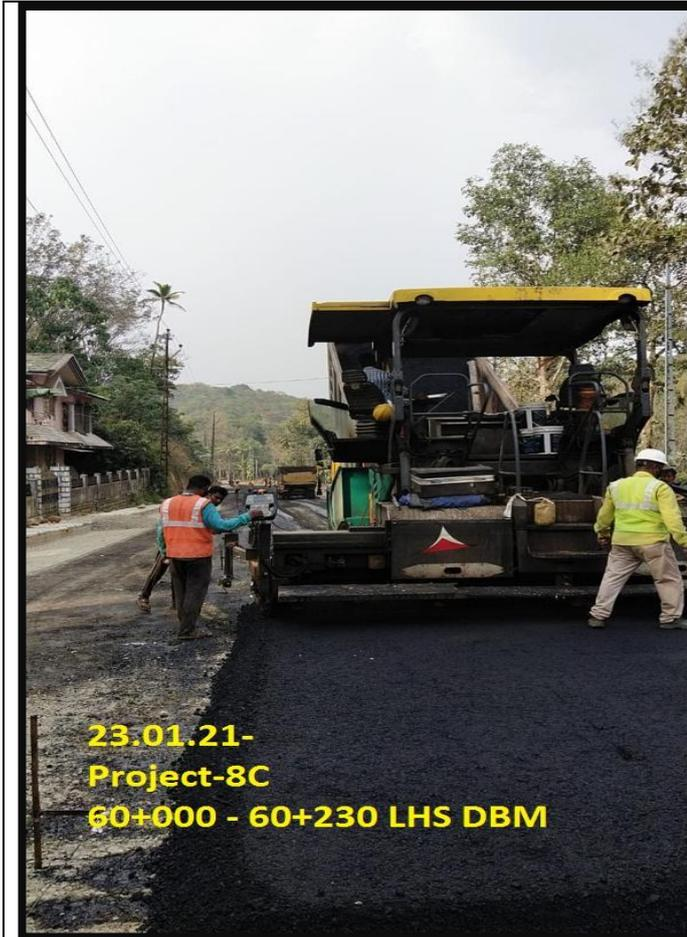
DBM Laying work in progress at km.60+00 to 60+230
