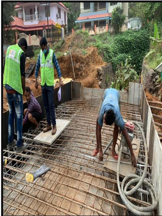
Box culvert slab reinforcement work in progress
