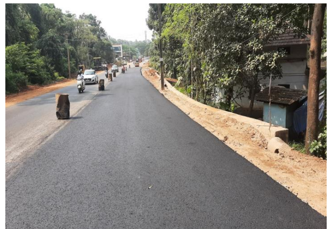
DBM LAYING @ 28+620-28+900 LHSDBM
