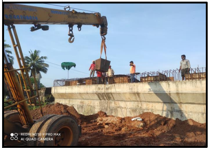
Pedestal @ Pier P1 – P2 Ch: 2+910
