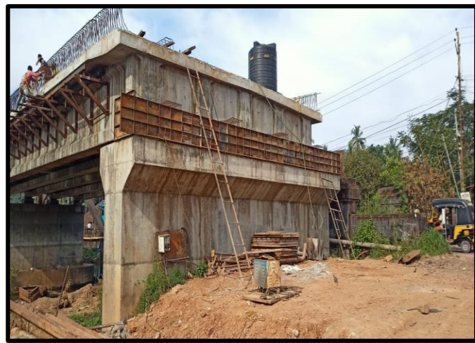
Abutment Cap @ A2 2+910
