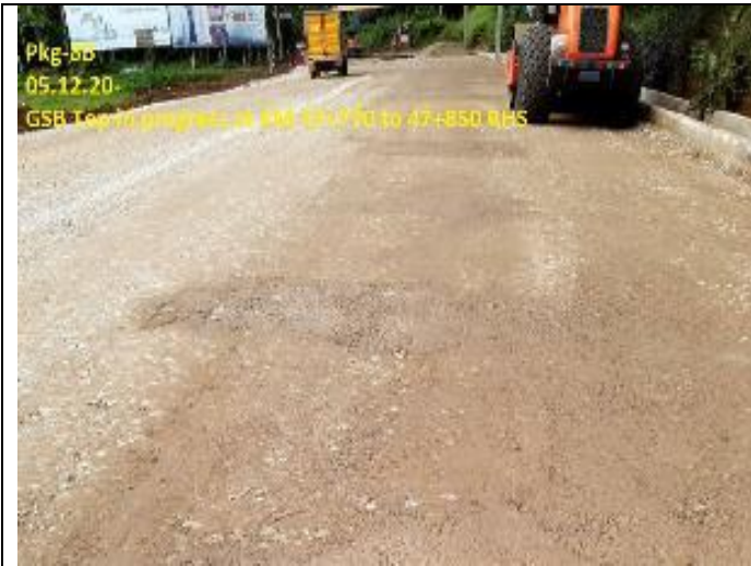
GSB laying work in progress at km.47+770 to 850
