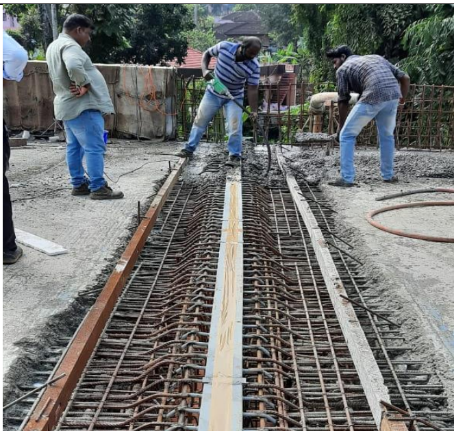
Expansion Joint fixed at P6
