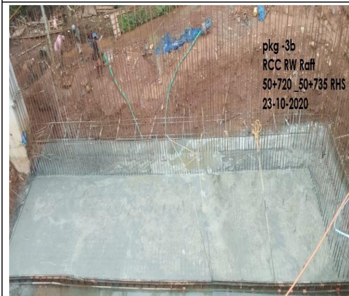
• RCC retaining wall Raft Km 50+720 to 50+735 RHS
