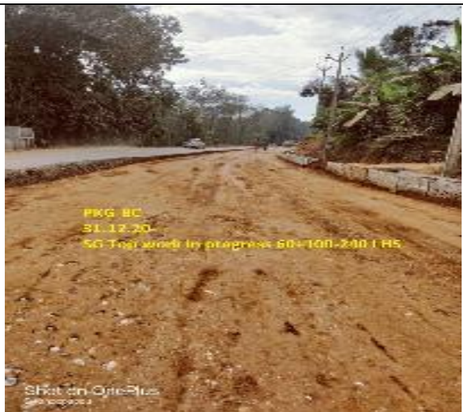
SG Top work in progress 60+100-240 LHS
