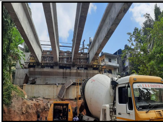
Cross Girder concrete at A1, Viaduct
