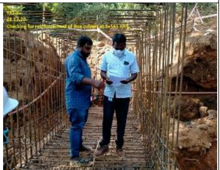
Checking for reinforcement of Box culvert at 3+565 RHS.
