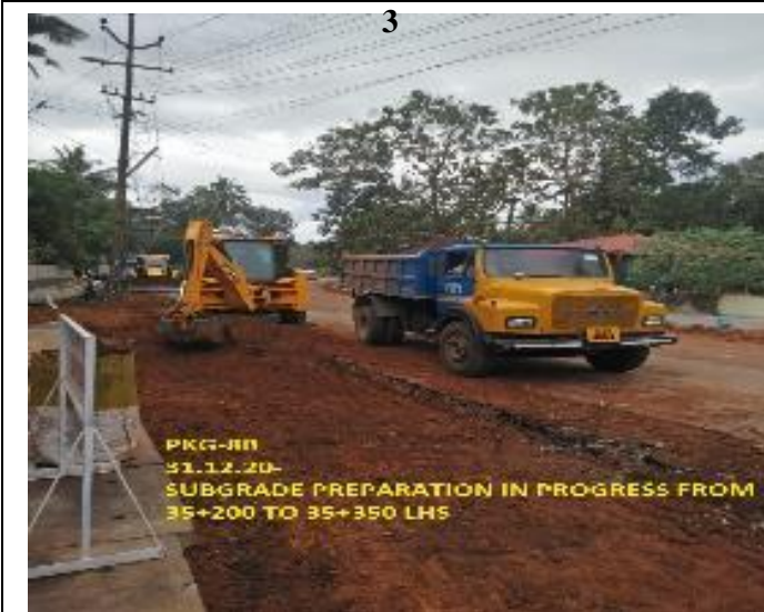
Subgrade work in progress at km.35+200 to 350
