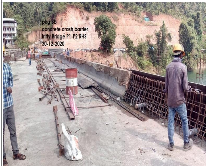
• Irritty Bridge at km 42+198 Crash Barrier P1-P2
