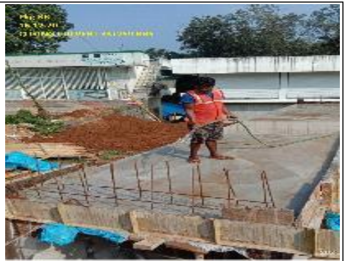
Curing work in progress
