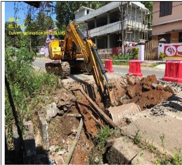
Culvert excavation work progress at km.99+236
