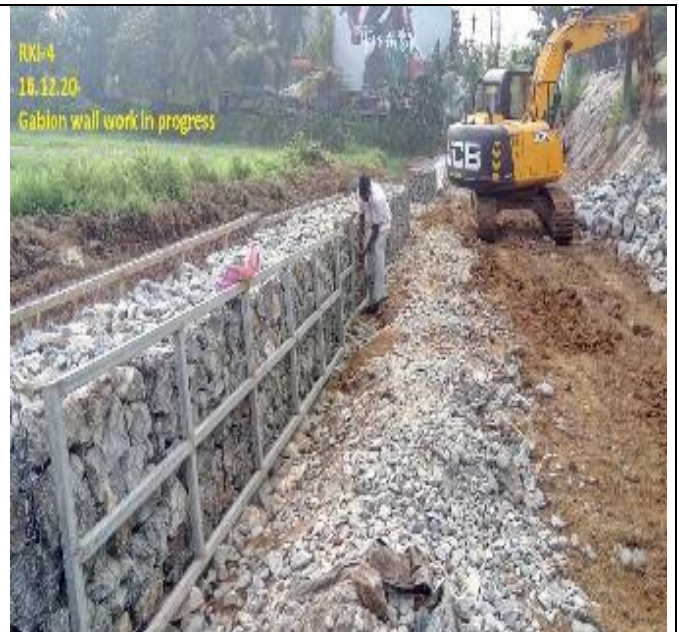
Gabion wall work in progress
