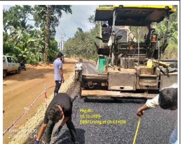
16.12.20-DBM Laying at CH62+960 RHS
