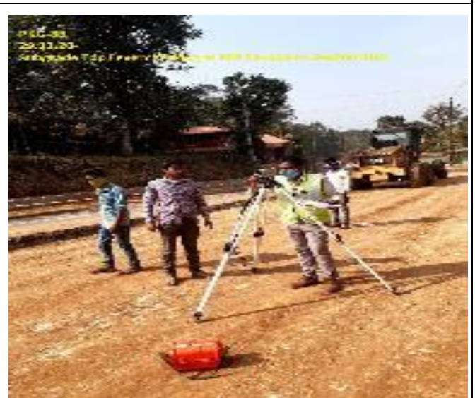
SG work in progress at km.59+600 to 59+700
