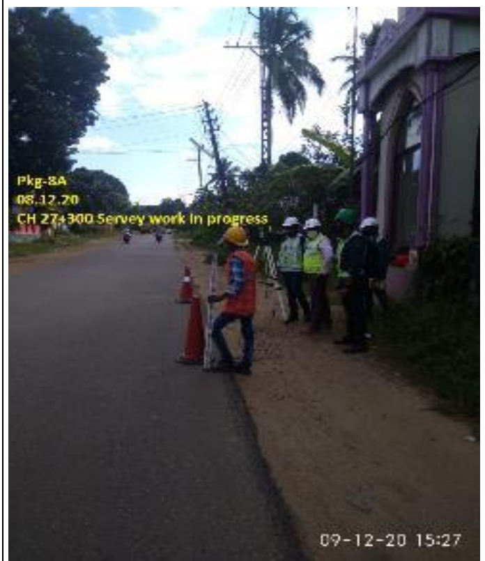
Survey work in progress
