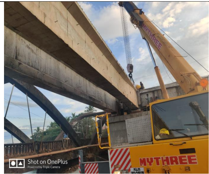
Girder Launching Completed B/w Pier P1-P2
