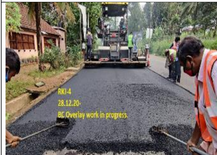
BC overlay work in progress
