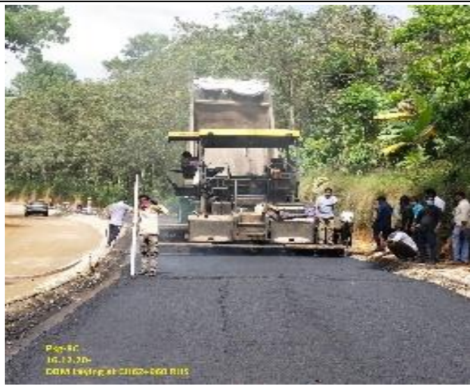
BM Laying at Ch63+030...
