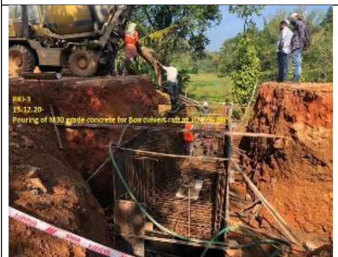
Pouring of M30 grade concrete for Box culvert raft at 10+996 BHS..
