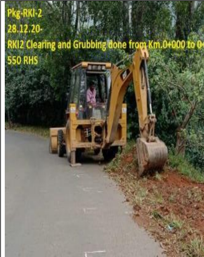
C&G work in progress
