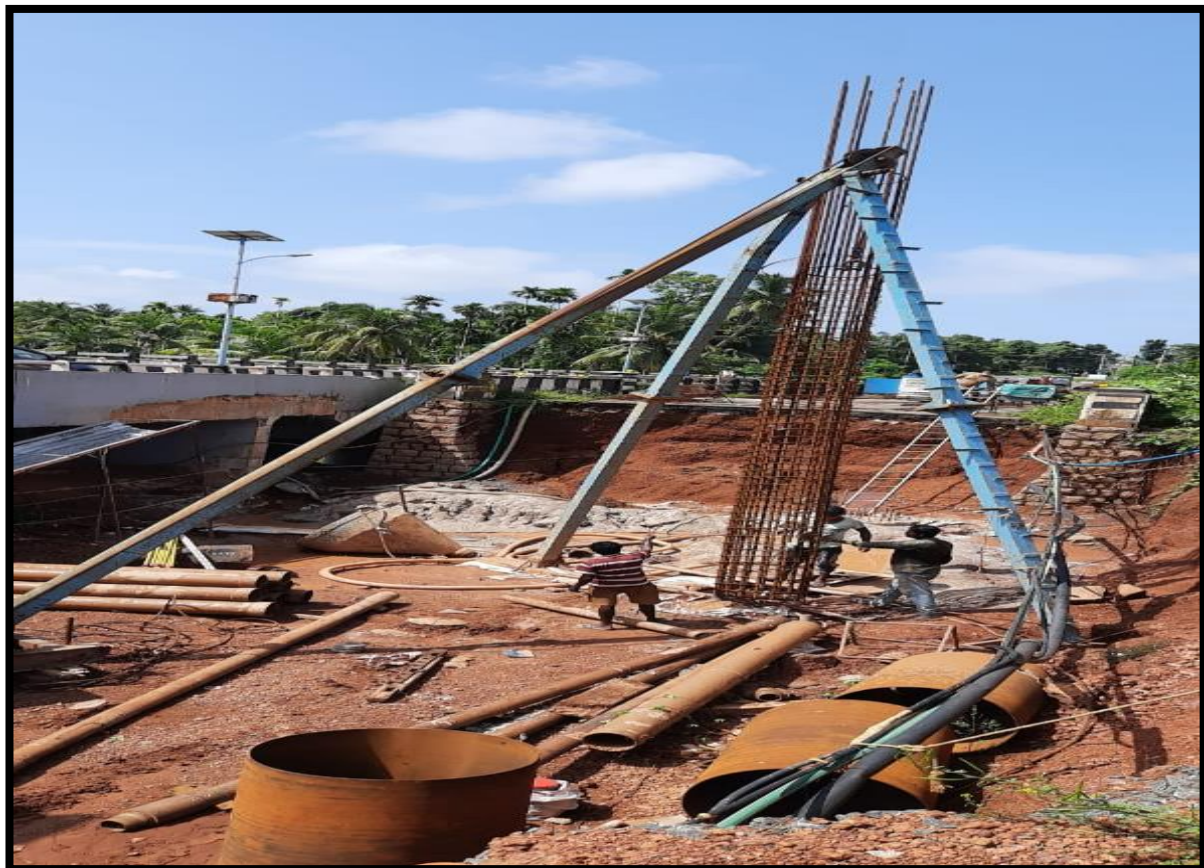
Ramapuram Existing bridge approach
