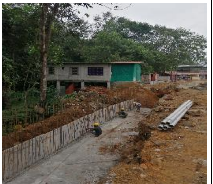
Toe wall work in progress
