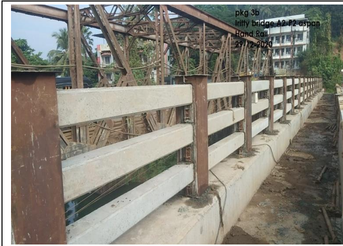
Irritty Bridge at km 42+198 Hand rail
