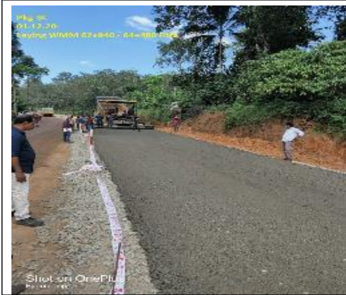
Laying WMM 62+940 - 64+400 RHS
