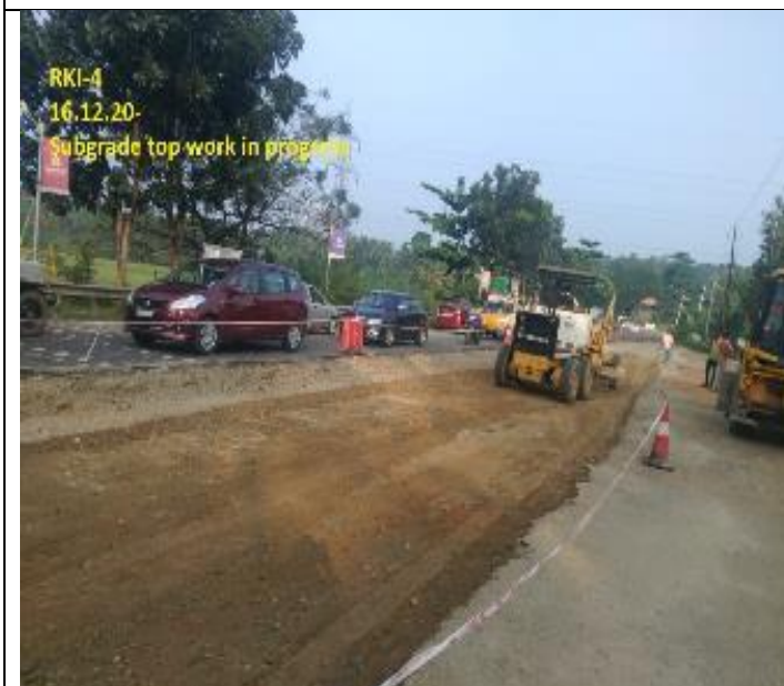
Subgrade top work in progress
