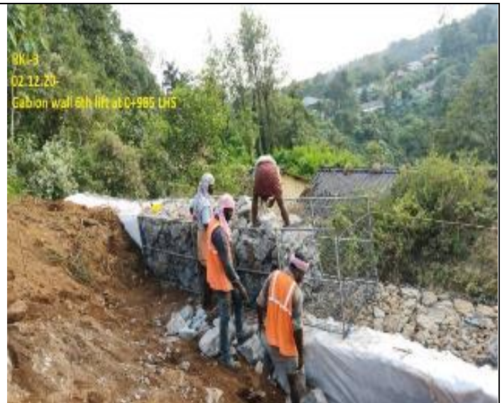
Gabion wall 6th lift at 0+985 LHS
