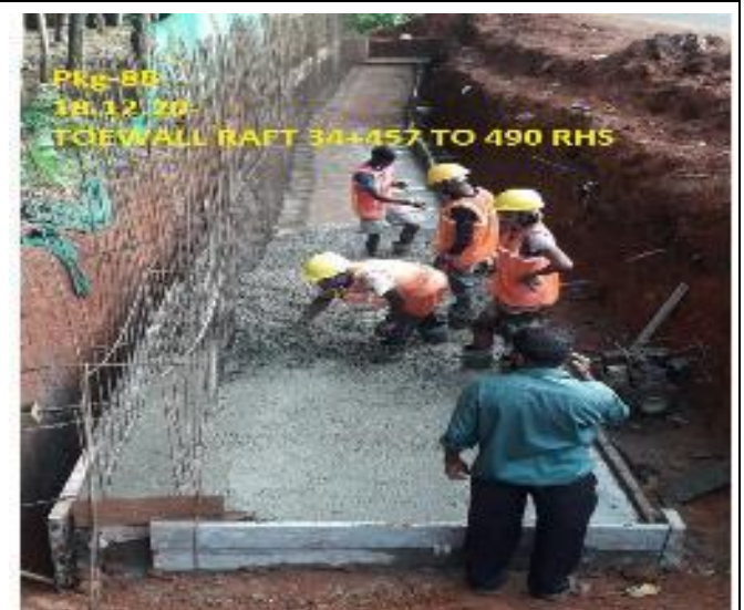
Toe wall Raft work in progress at km.34+457 to 34+490
