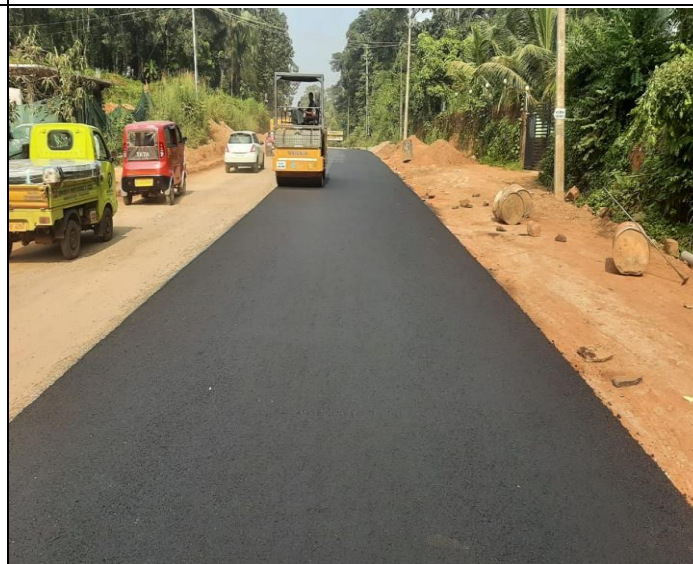
DBM LAYING @ 28+620-28+830 RH
