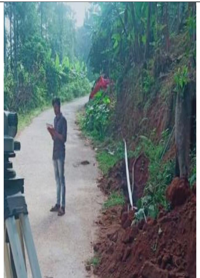
Culverts inventory levels checking work in progress
