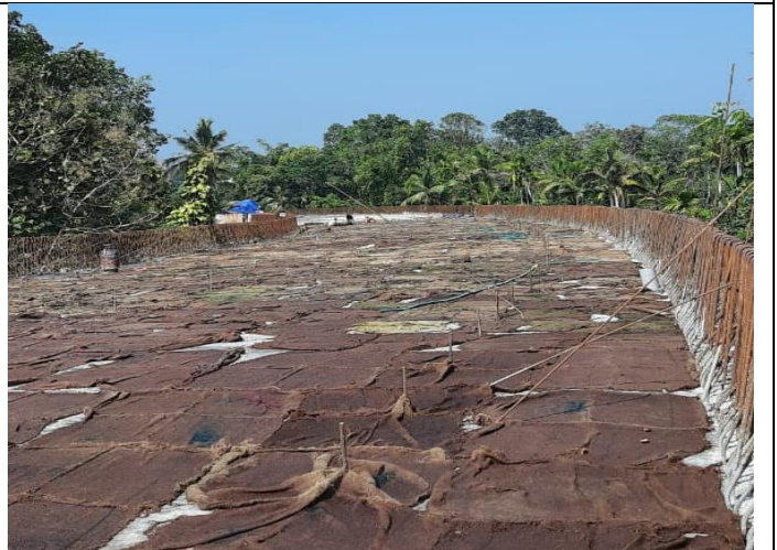
Deck slab concrete completed in all spans of viaduct
