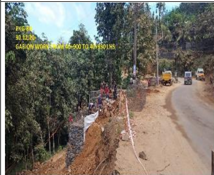
Gabion wall work in progress at km40+900
