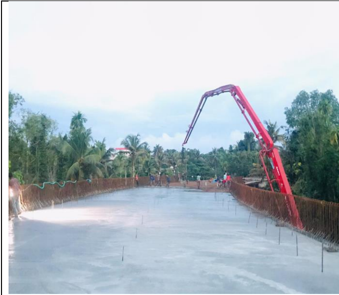
Deck slab concrete P3-P2, Viaduct
