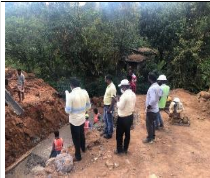
Laying of PCC at 11+821 Box culvert BH
