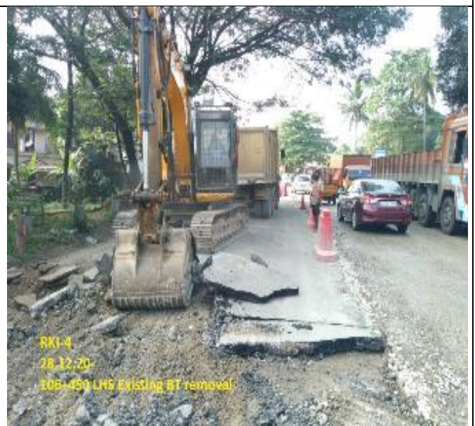
106+450 LHS Existing BT removal
