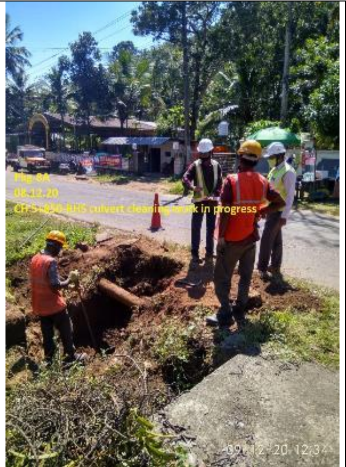
Culvert cleaning work in progress
