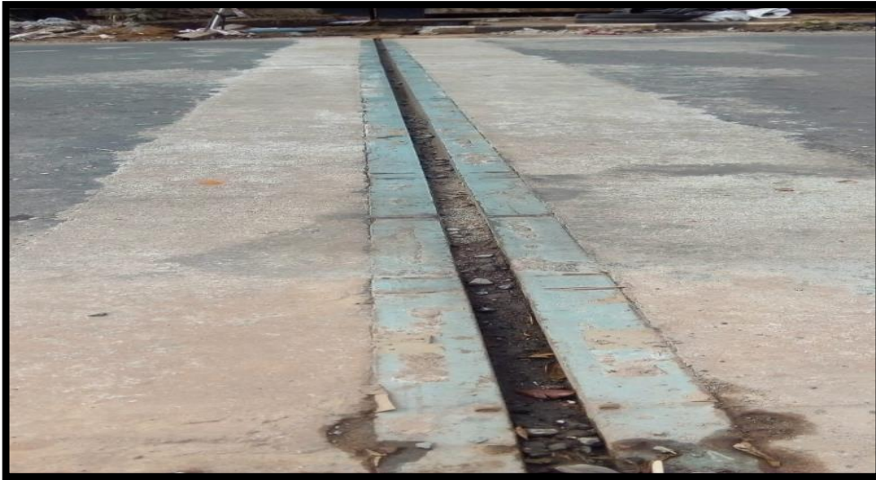
Chandrigiri Bridge Expnasion Joint
