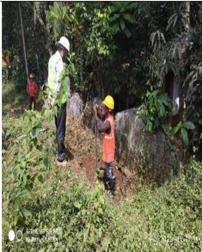
Culvert cleaning work in progress
