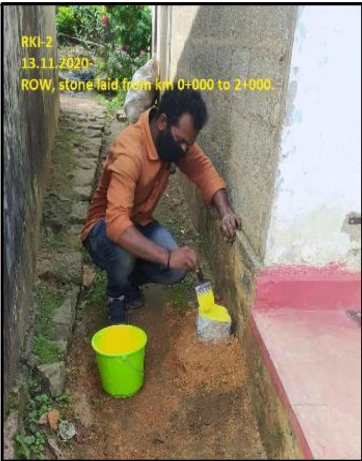
ROW Stone laying work in progress
