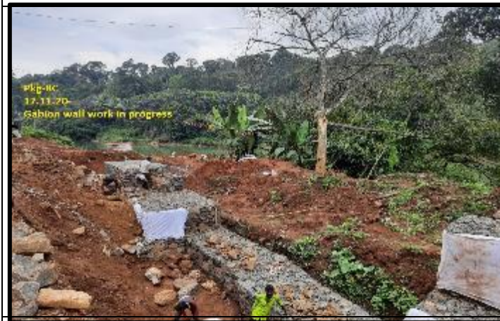
Gabion wall work in progress
