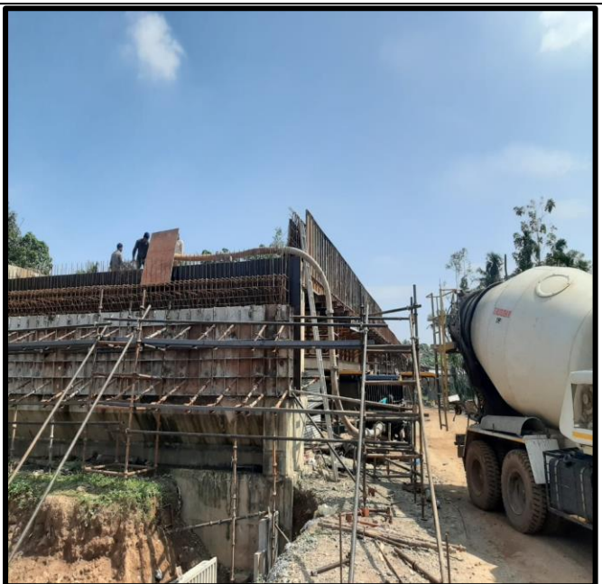
Cross Girder concrete at A1, Viaduct
