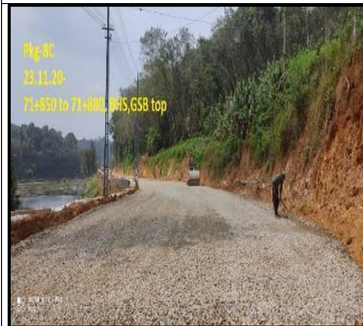
GSB Laying work in progress
