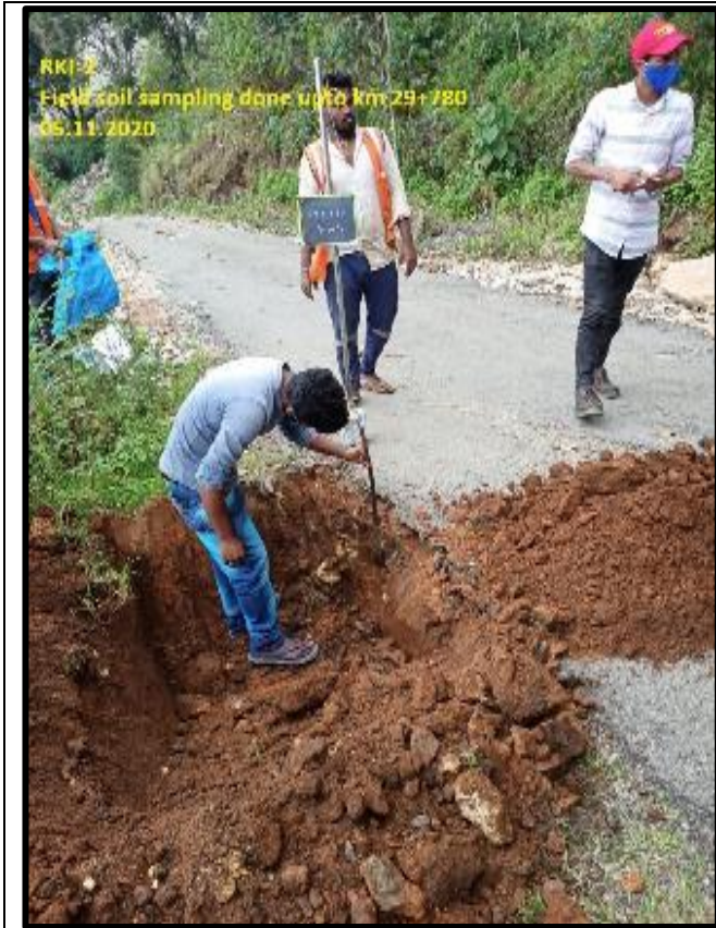
Soil sampling for sub soil investigation
