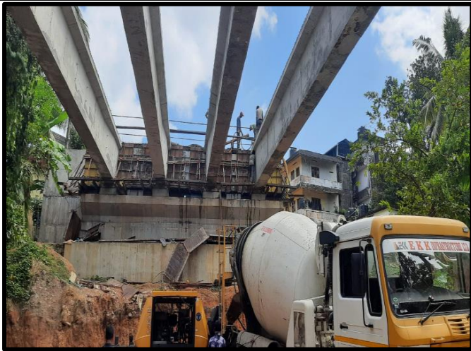
Cross Girder concrete at A1, Viaduct
