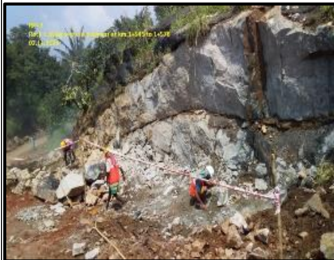
Rock cutting work in progress
