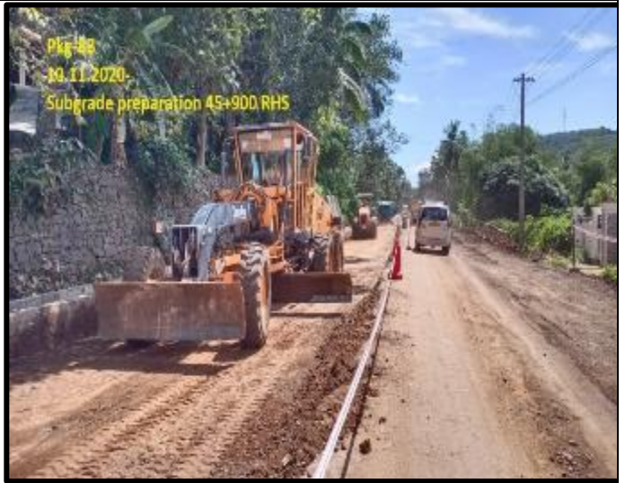
SG work in progress at km.45+900 RHS
