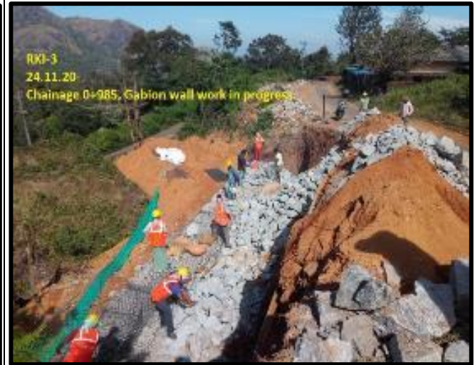
Gabion wall work in progress
