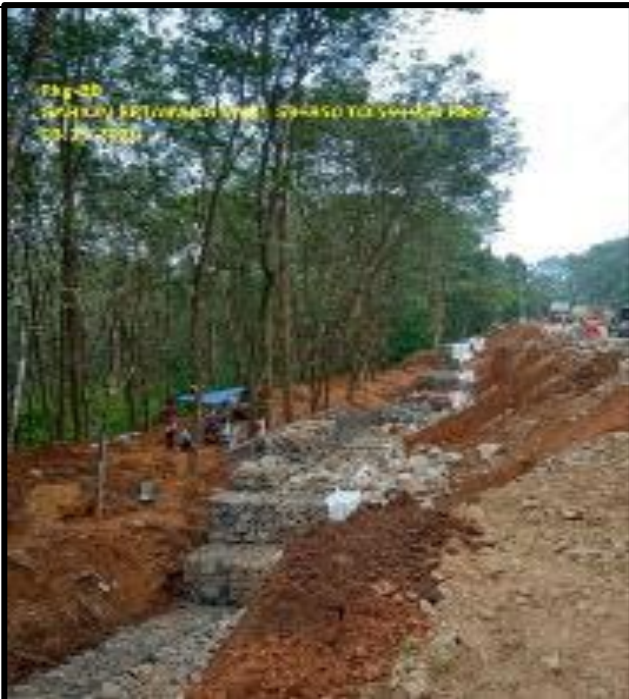
Gabion wall work in progress
