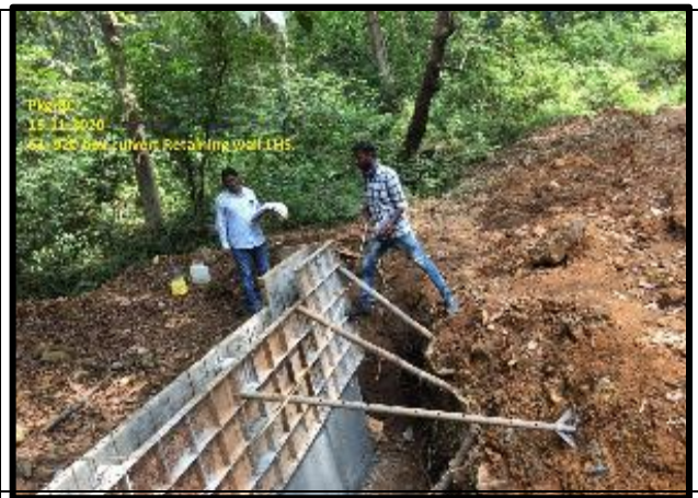
Concreting work in progress Box culvert return wall
