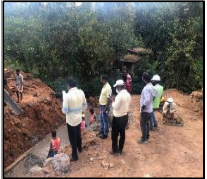
Culvert PCC work in progress
