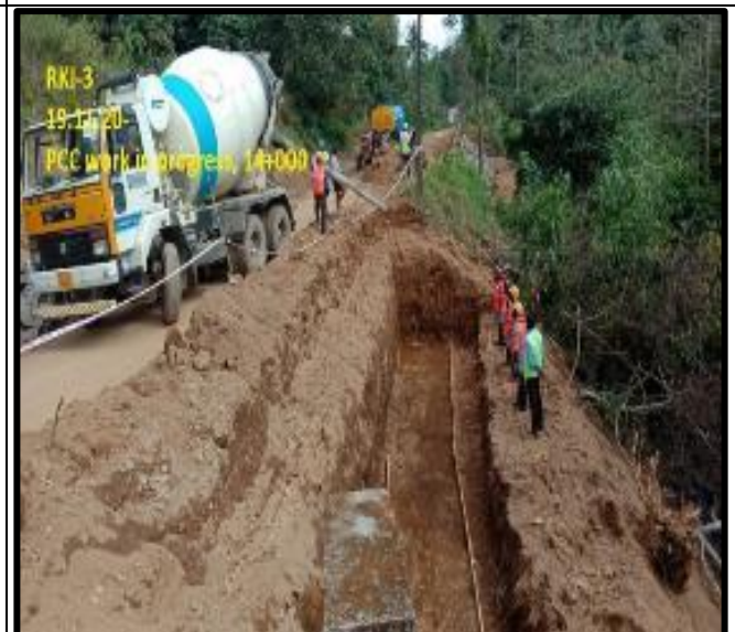
PCC work in progress at km.14+00
