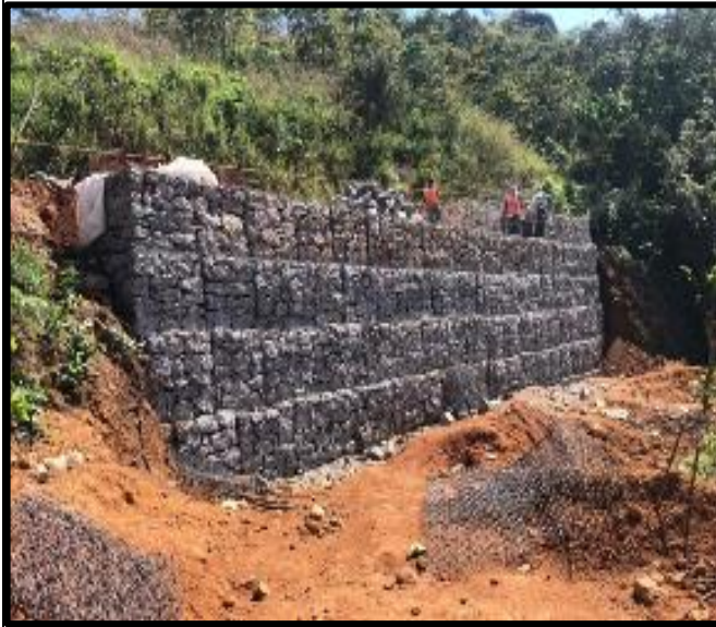
Gabion wall work in progress
