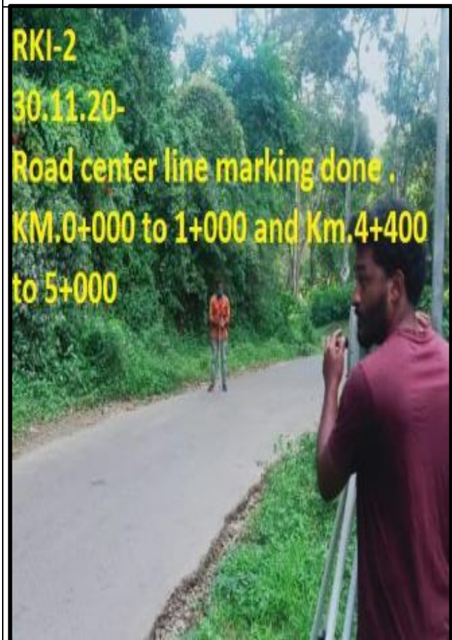
Centre line marking work progress
