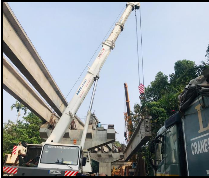
Girder erection work for P3-A1 completed
