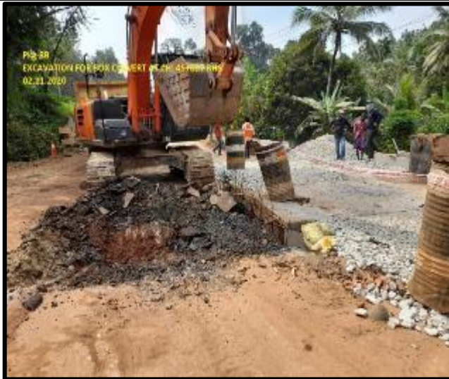
Excavation for culvert at km45+697
