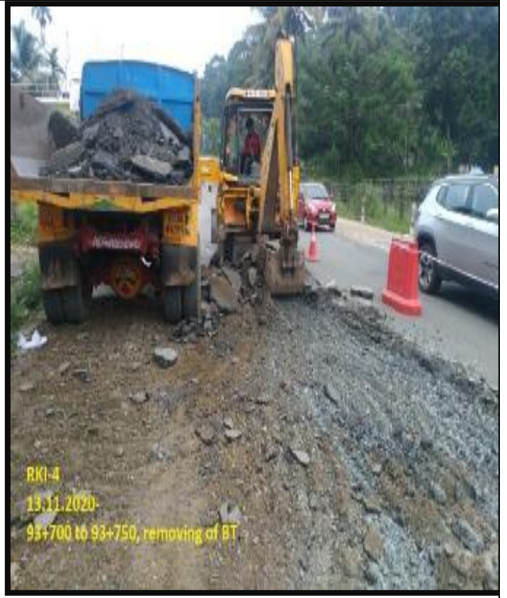
BT Scarification work in progress
