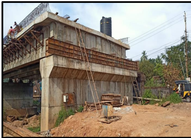
Abutment Cap @ A2 2+910
