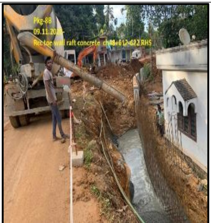
RCC Toe wall raft concrete -48+612 RHS
