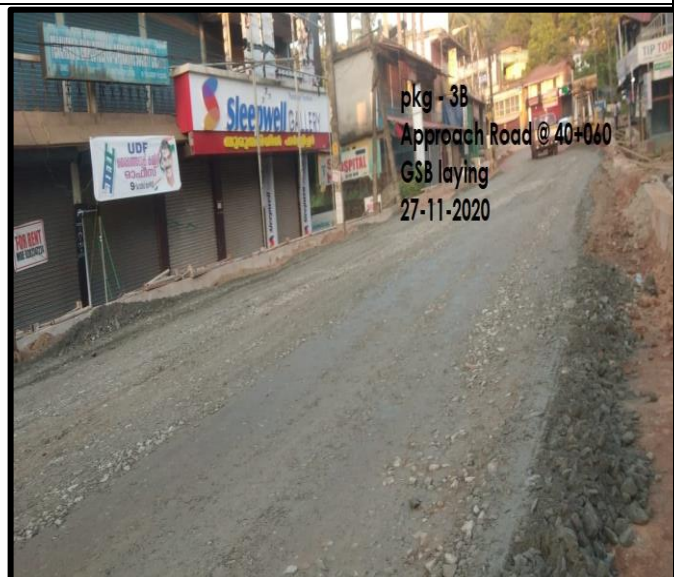
GSB laying for access road at Km 40+060 RHS
