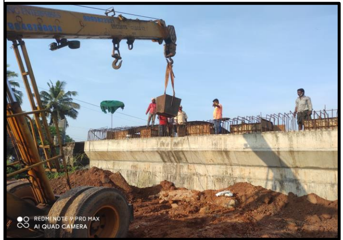
Pedestal @ Pier P1 – P2 Ch: 2+910
