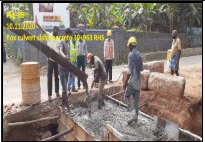
Box culvert work in progress
