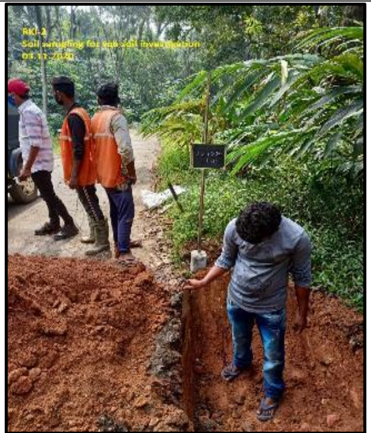
Soil sampling for sub soil investigation
