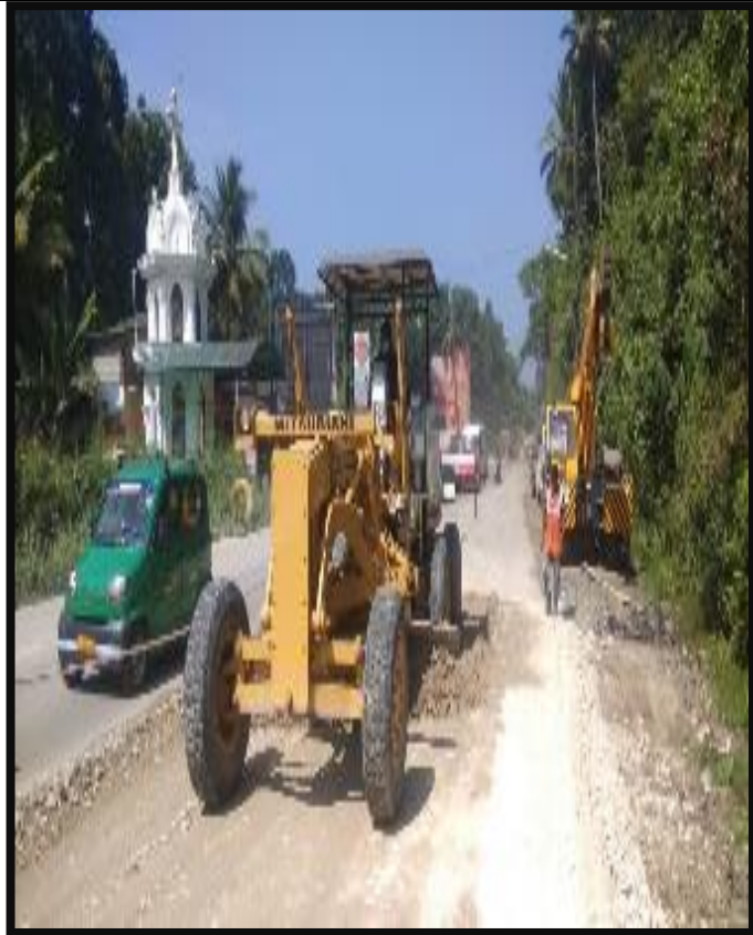
WMM Laying work in progress
