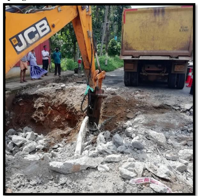
Dismantling of existing culvert work is in progress at Km 111/800,LHS
