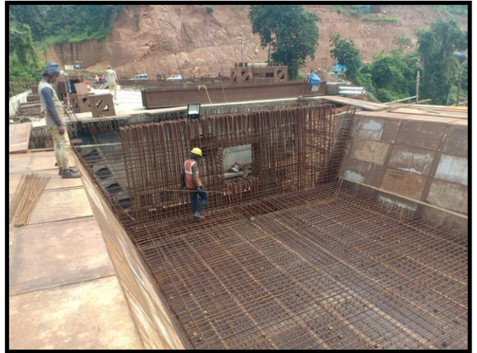
Iritty Bridge at km 42+198 SPAN P1-P2 reinforcement work in progress
