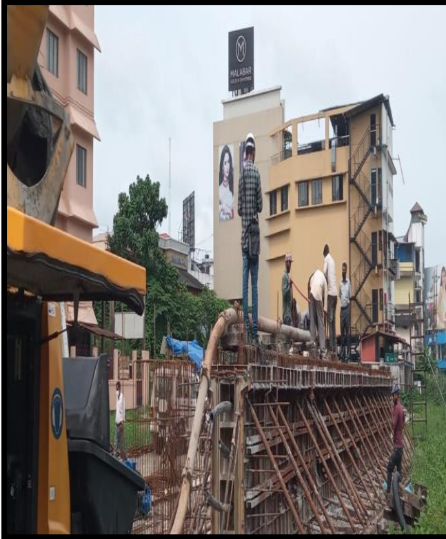
Girder concreting work at casting yard
