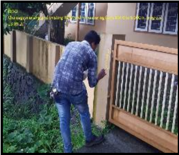
Chainage marking in progress
