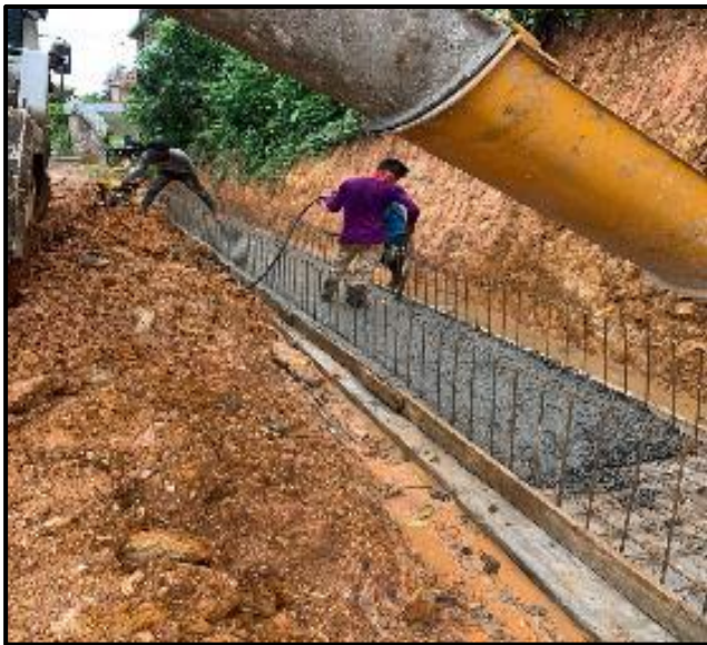
DRAIN RAFT COCRETE FROM 48+426 to 48+465 LHS
