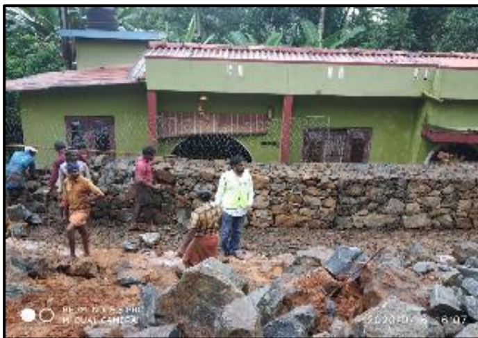
Gabion wall work in progress
