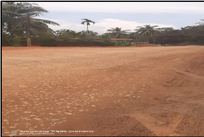
SG WORK 26+530 – 26+570 RHS
