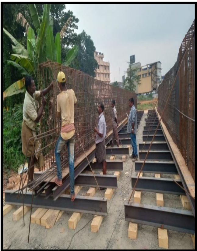
Girder reinforcement work, Viaduct
