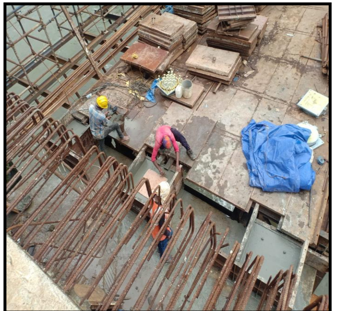
Iritty Bridge at km 42+198 pedestal concrete for P1 & P2
