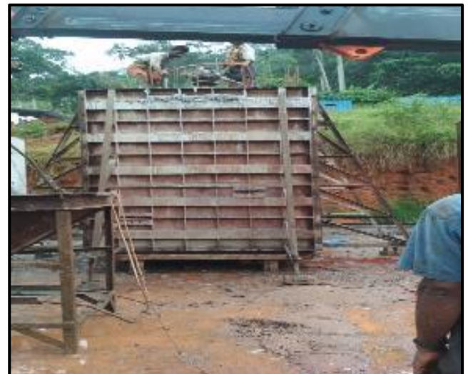
PRECAST BOX CULVERT PLACING 48+060 RHS
