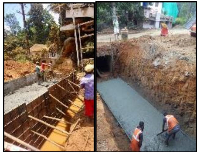
Culvert work in progress
