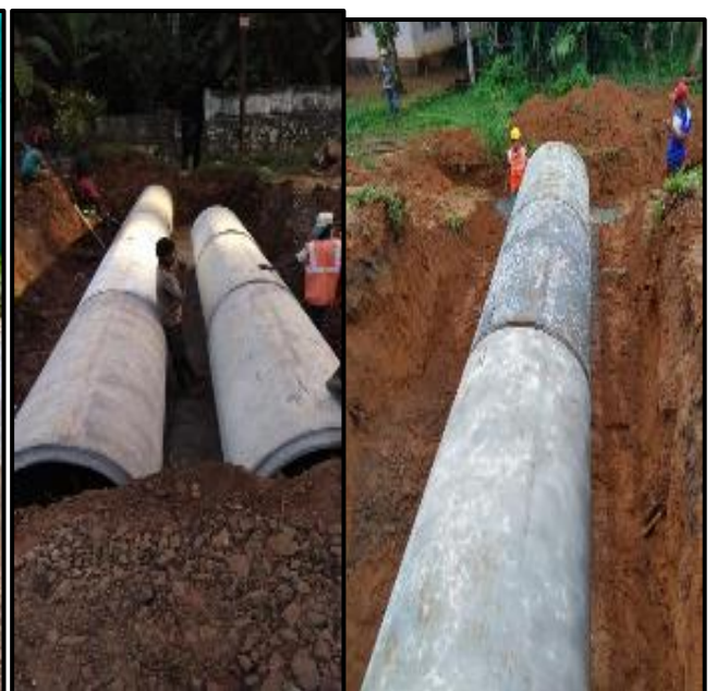
Pipe laying work in progress
