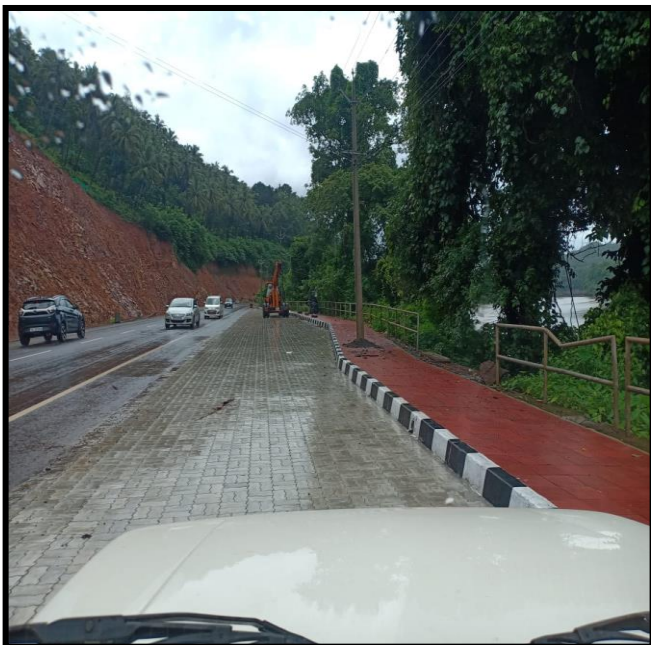
Paver block and footpath at km 42+320 .
