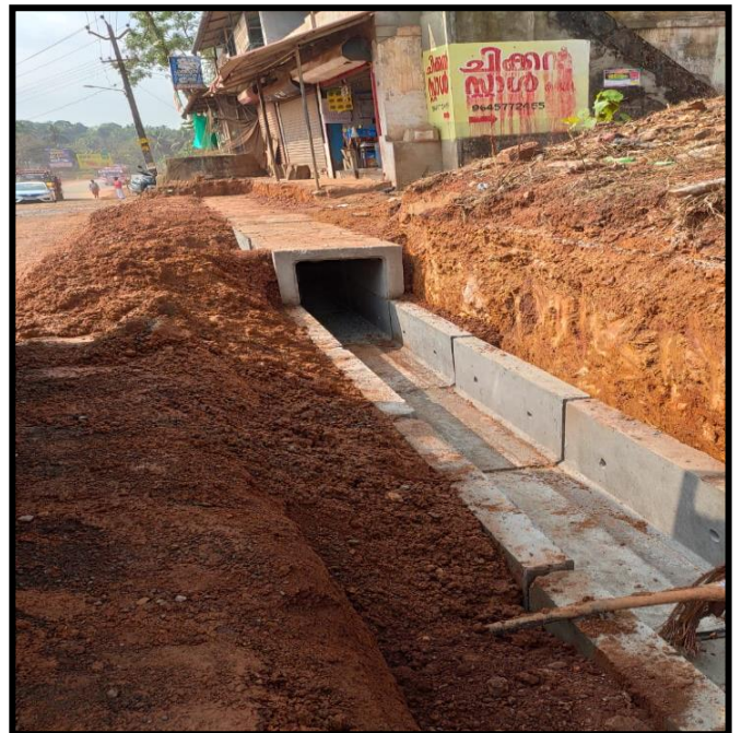
DRAIN LAYING @ 24+928-24+940 RHS
