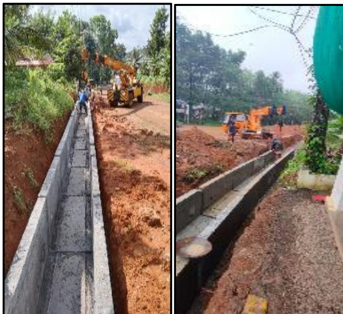
Drain work in progress
