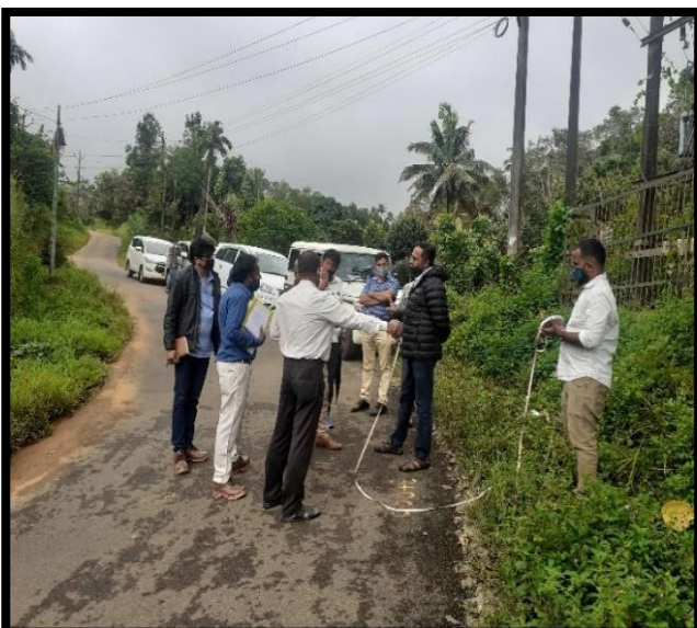
Authority Engineer Mr.Jwalendra kumar visited the site on 16.09.2020
