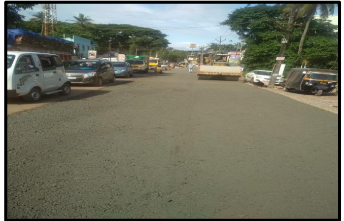
WMM 2 nd LAYER @ CH 27+270 – 27+440 RHS
