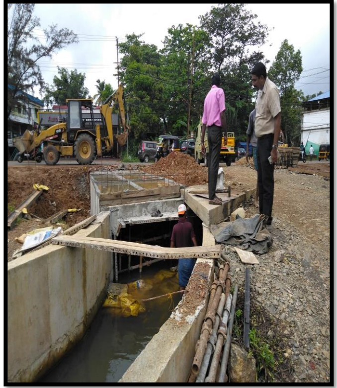
Culvert widening upto slab work completed at 2+300, RHS
