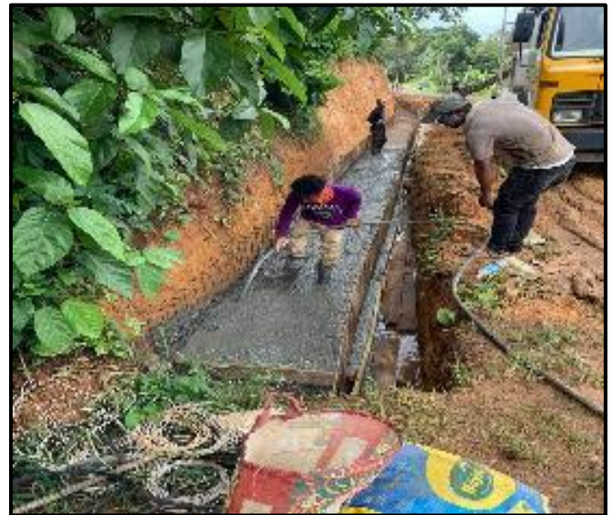
DRAIN RAFT COCRETE FROM 48+426 to 48+465 LHS
