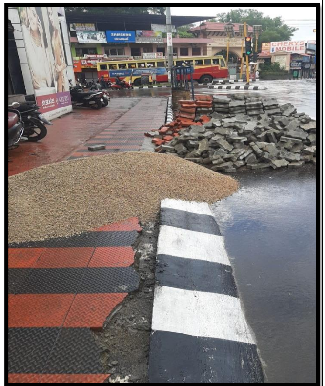
Footpath work in progress at 1+180
