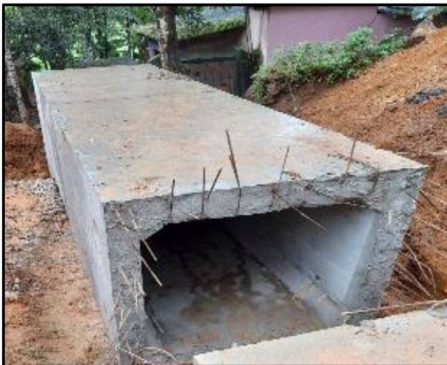
PRECAST BOX CULVERT PLACING 48+060 RHS
