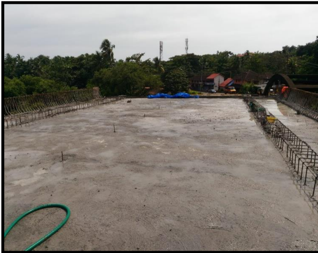
DECK SLAB P2-P3 @ 2+910 ERANHOLI BRIDGE
