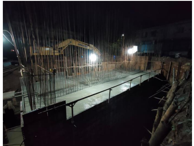
PILE CAP @ CH:2+910 ABUTMENT A2
