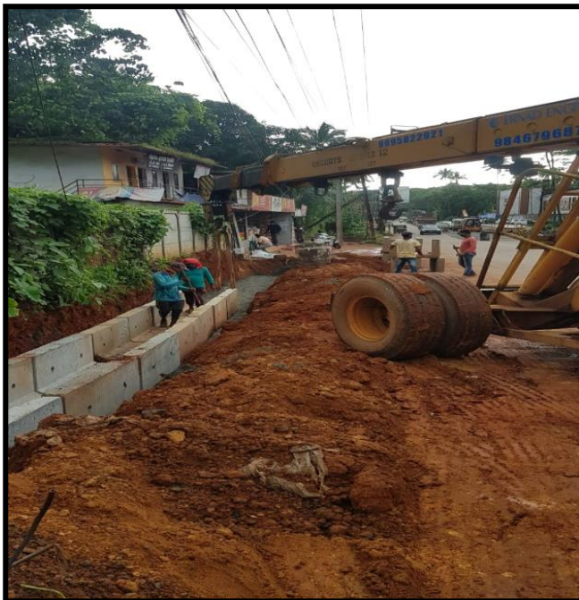
DRAIN LAYING @ 25+950-25+970 RHS
