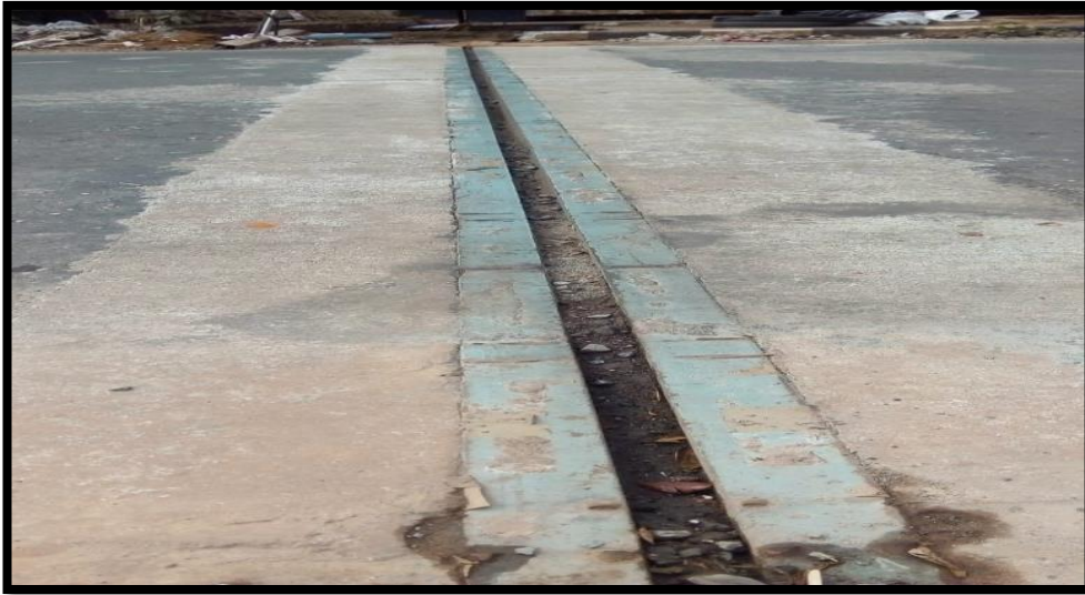
Chandrigiri Bridge Expansion Joint
