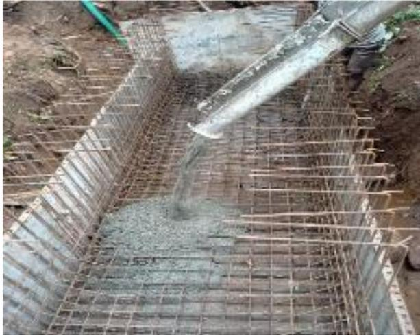
**Box culvert Raft work in progress**
