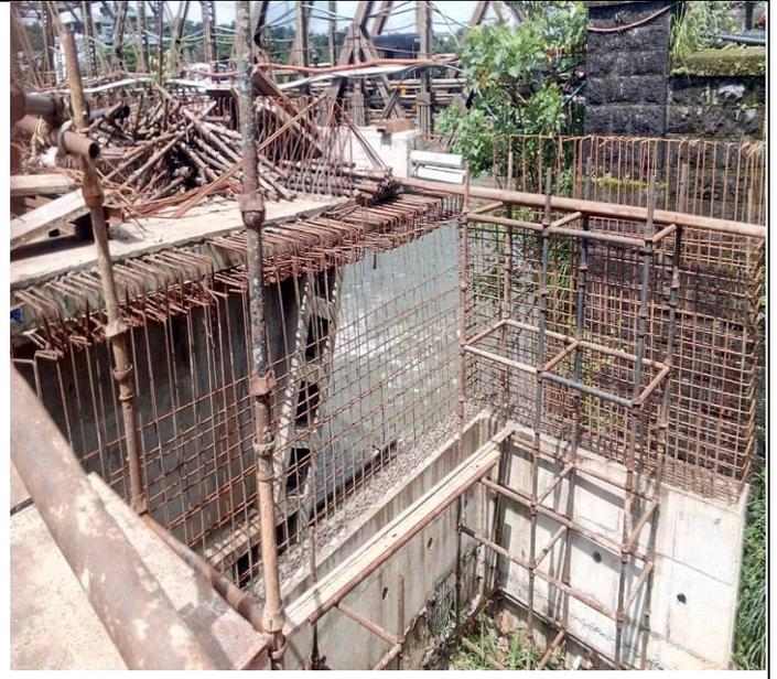
**Iritty Bridge at km 42+198 Dirt wall A2 side reinforcement work in progress**
