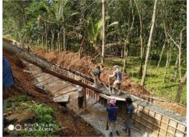
**Toe wall concreted work in progress**
