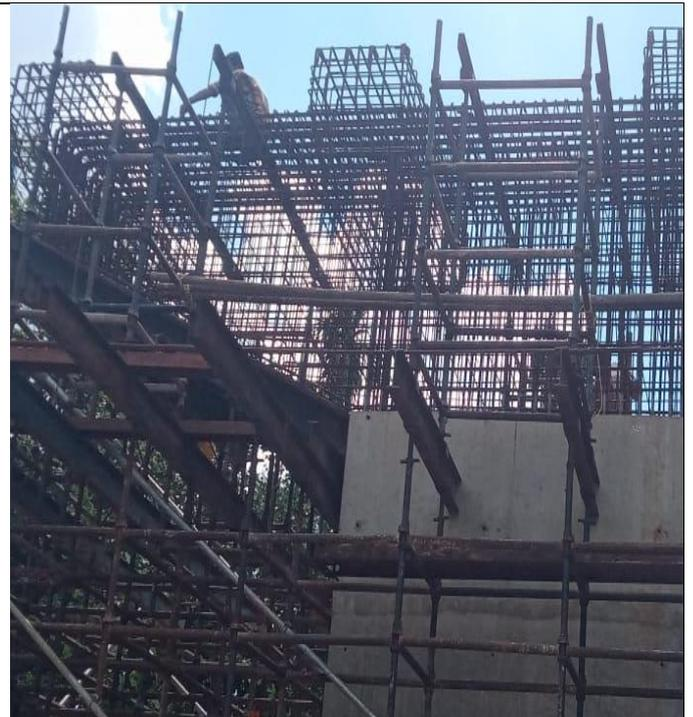
**Piercap Reinforcement work on P2, Viaduct**
