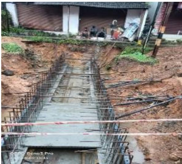
**Box culvert work in progress**
