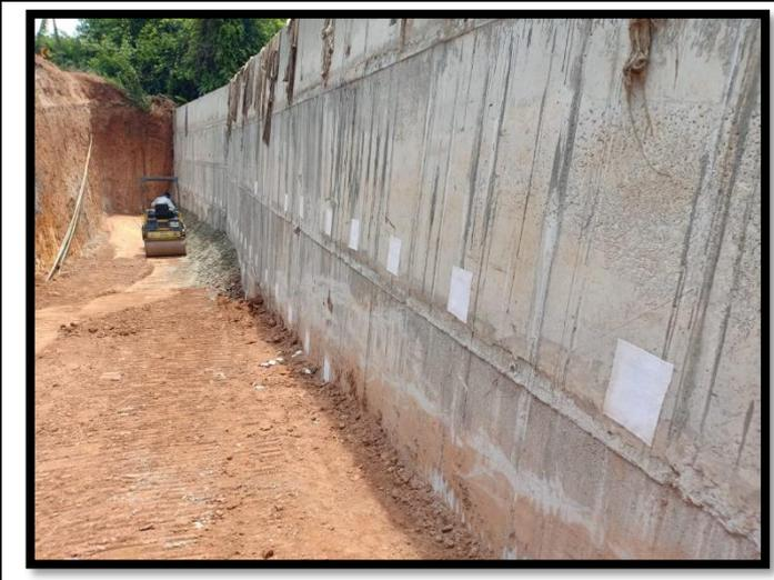
**Iritty Bridge at km 42+198 A1 side (RHS) approach filter media laying for stone pitching**
