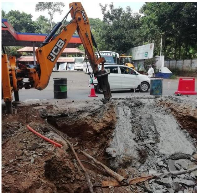
**Dismantling of existing road cross structure work is in progress at Km 111+800.**
