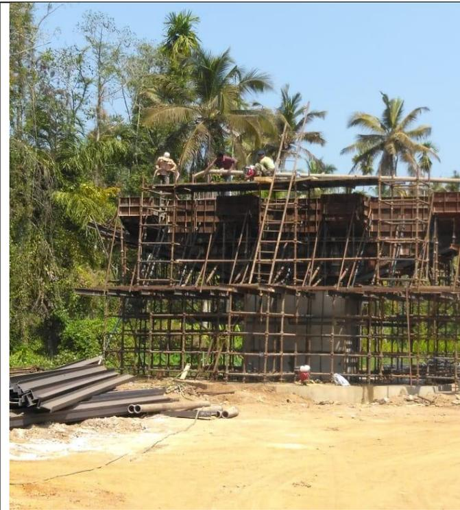
**Piercap concrete work on P3, Viaduct**
