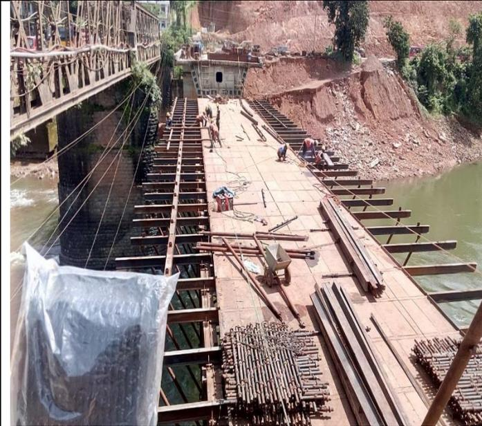
**Iritty Bridge at km 42+198 SPAN P1-P2 shuttering work in progress**
