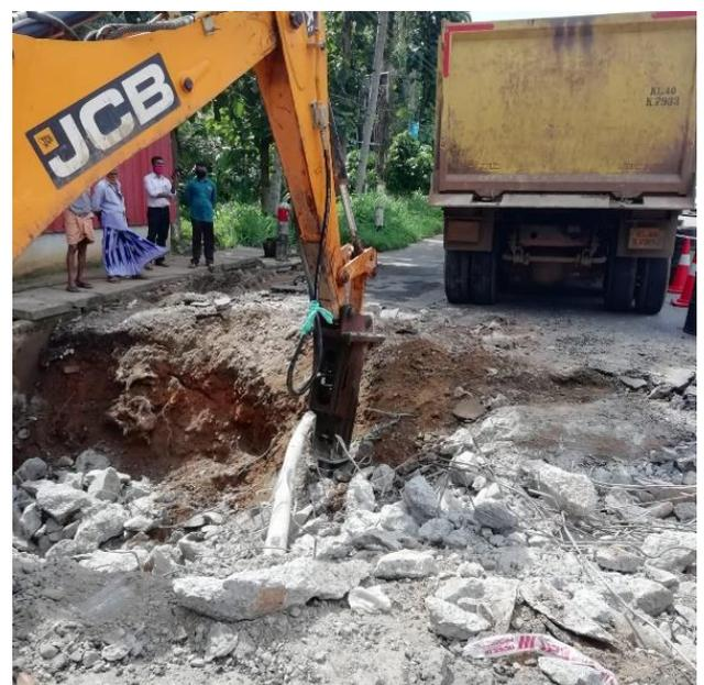
**Dismantling of existing culvert work is in progress at Km 111/800,LHS**
