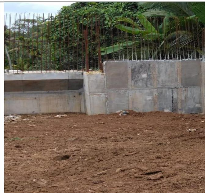
**L wall completed up to 2<sup>nd</sup> Lift**
