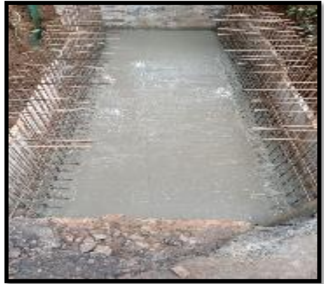
Box culvert work in Progress
