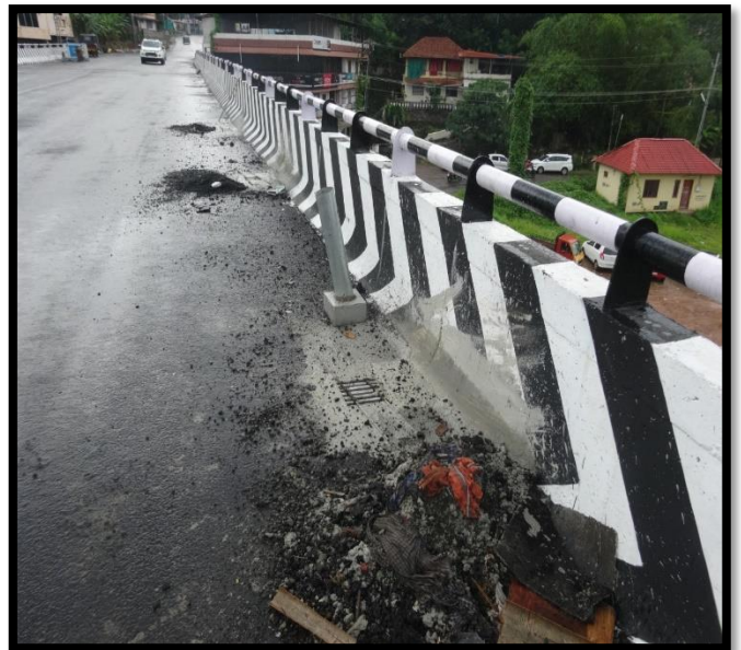
Drainage spout fixing work over Flyover
