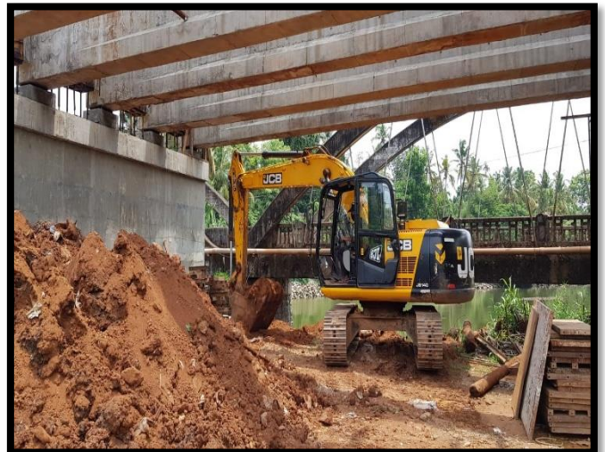
EARTHEN ISLAND REMOVAL WORK IN PROGRESS AT ERANHOLI BRIDGE
