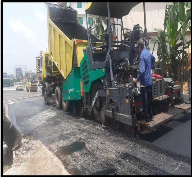
BC Laying work at Km:1+410
