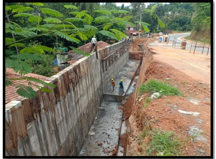
52+600 RHS retaining wall work in progress.
