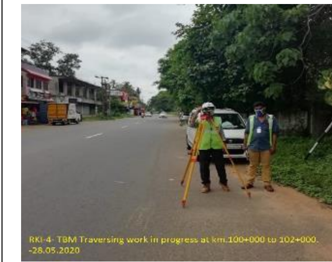
TBM Traversing work in progress
