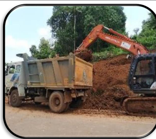
EXCAVATION IN PROGRESS CH: FROM 47+950 TO 48+170 LHS
