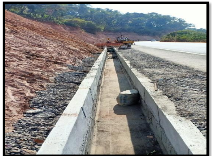
Drain work in progress.
