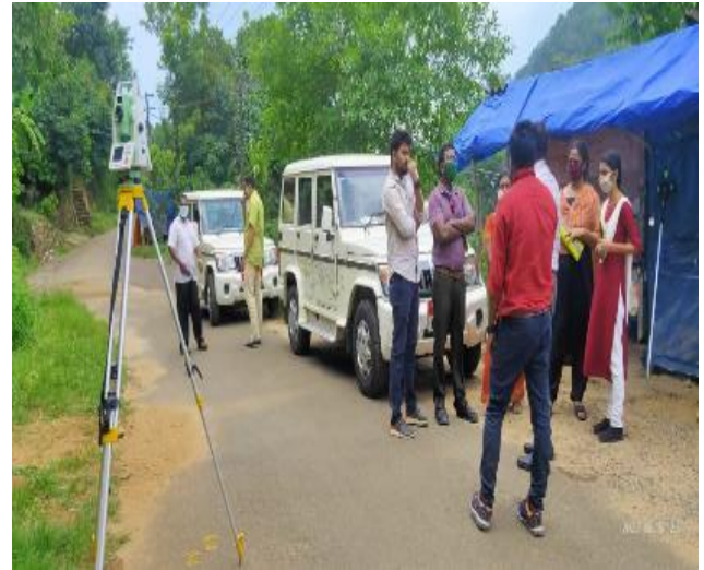
RKI 3 (Painavu to Ashokakavala) Road Executive Engineer, Muvattupuzha visited the site along with EPC Contractor
