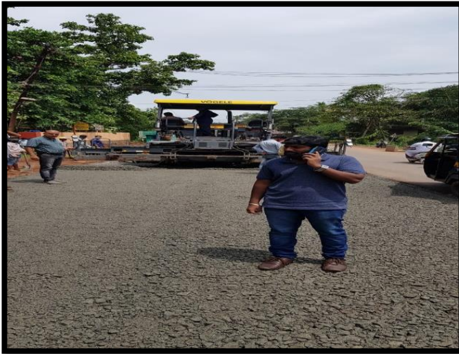
WMM 2 nd LAYER @ CH: 27+420- 28+100 RHS
