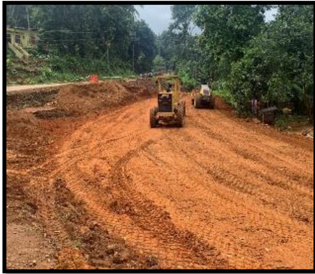
Embankment Filling work in Progress
