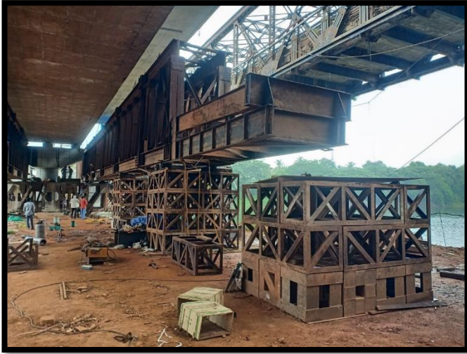
Iritty Bridge N- truss shifting for P1-P2 span
