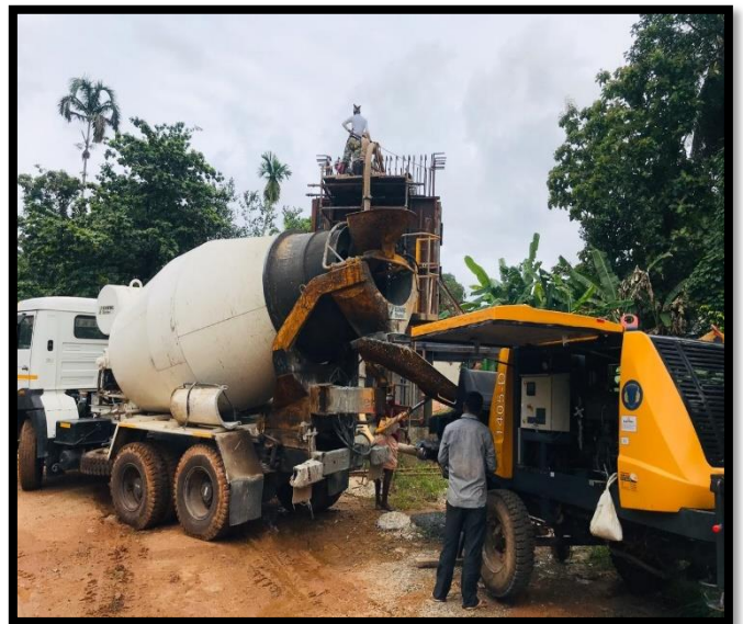
Pier P2 final lift Concreting
