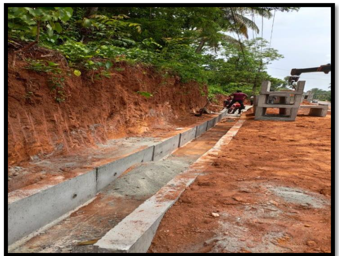
DRAIN LAYING @ 21+510 LHS
