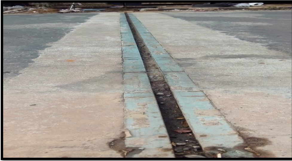
Chandrigiri Bridge Expansion Joint
