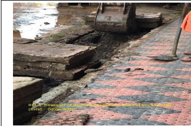
Culvert & Drain Cleaning Work in Progress
