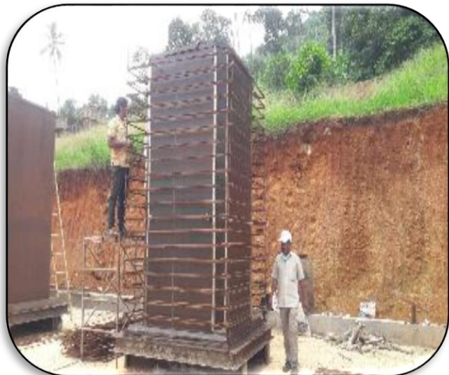
PRECAST BOX CULVERT REINFORCEMENT WORK IN-PROGRESS AT YARD
