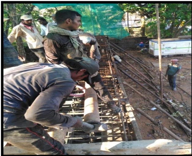
GIRDER CASTING @ CH 2+910
