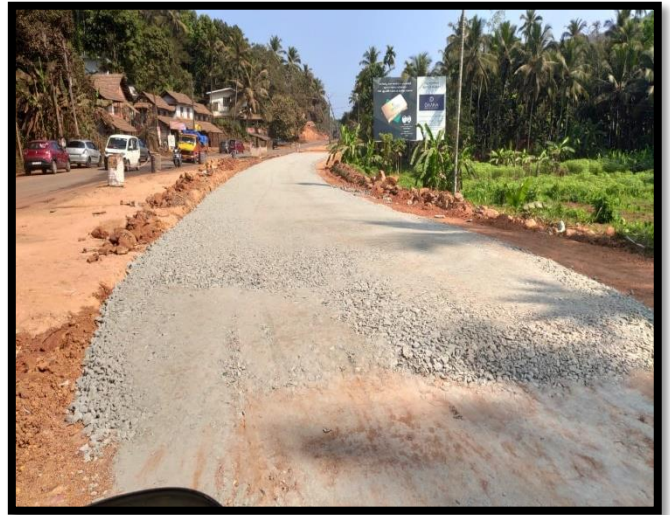
GSB IN PROGRESS AT 21+710 – 21+790 RHS
