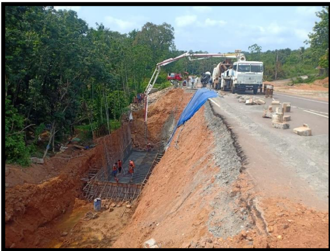
50+740 RHS retaining wall work in progress
