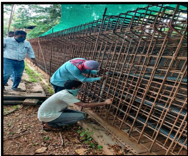
2 nd Girder Completd AT CH 21+135-21+180 RHS
