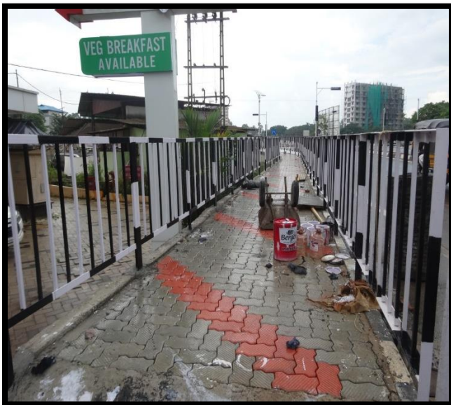
Handrail fixing work at 1+120, B1-B1 Junction
