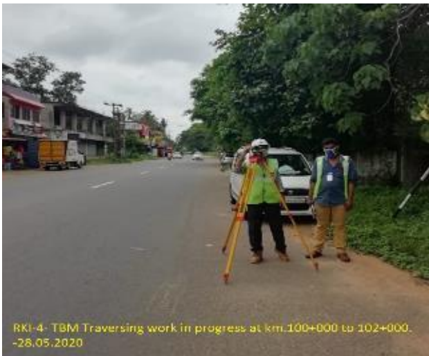
TBM Traversing work in progress
