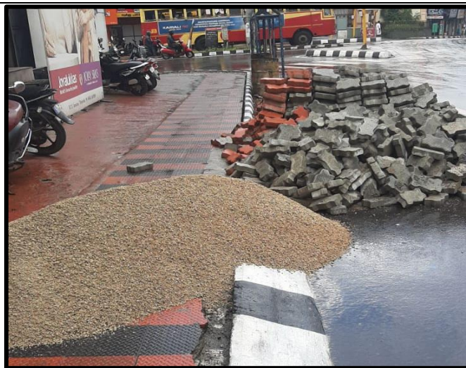
Footpath Laying work
