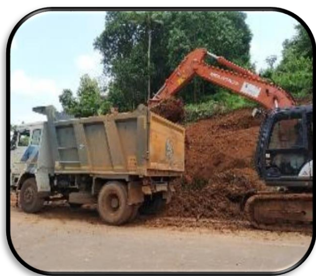
EXCAVATION IN PROGRESS CH: FROM 47+950 TO 48+170 LHS
