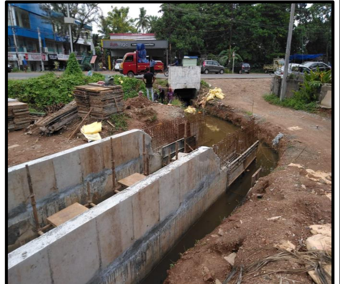
RCC Deep Drain work at 2+300,RHS
