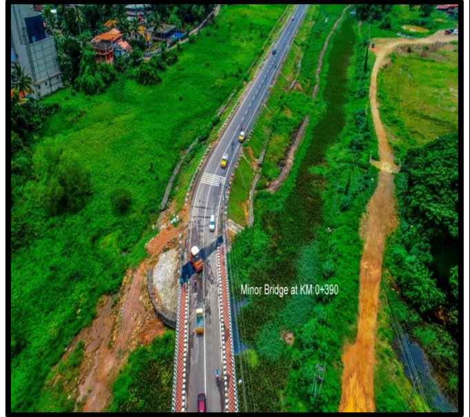
Minor Bridge, Thiruvalla Bypass
