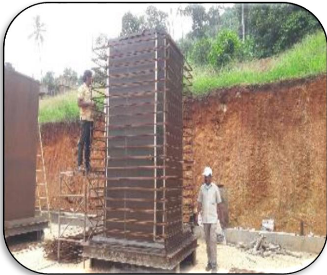
PRECAST BOX CULVERT REINFORCEMENT WORK IN-PROGRESS AT YARD
