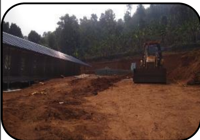
Staff quarters are in process
