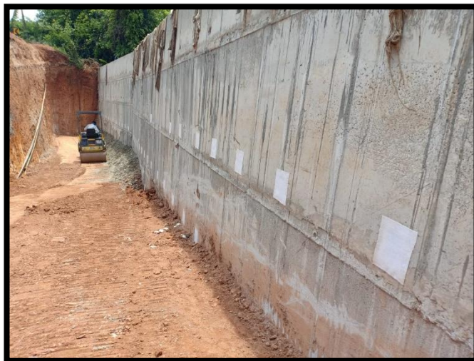
RHS retaining wall back filling work in progress
