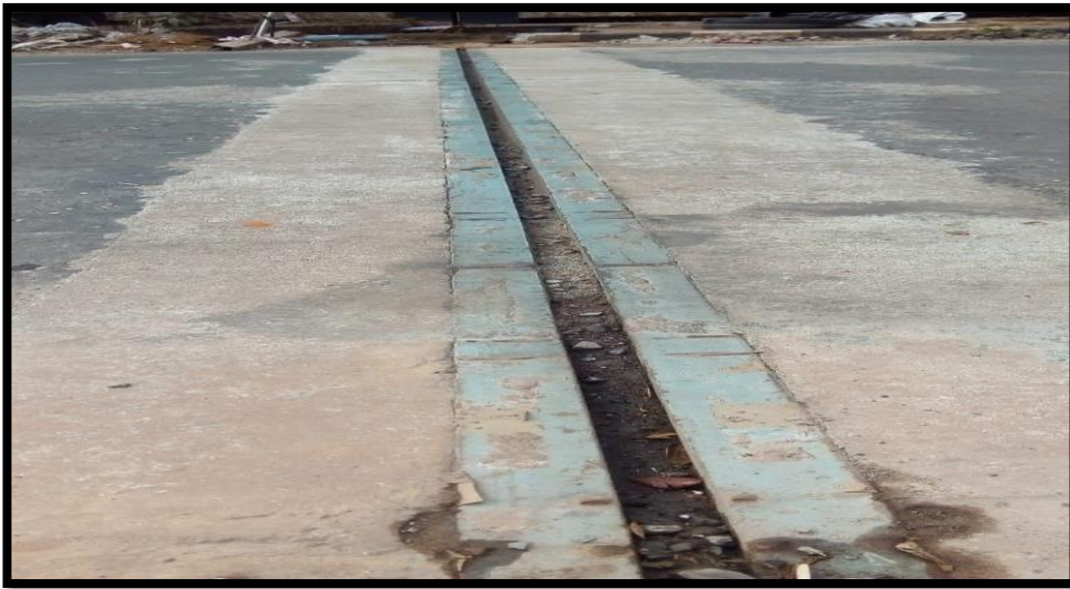
Chandrigiri Bridge Expansion Joint
