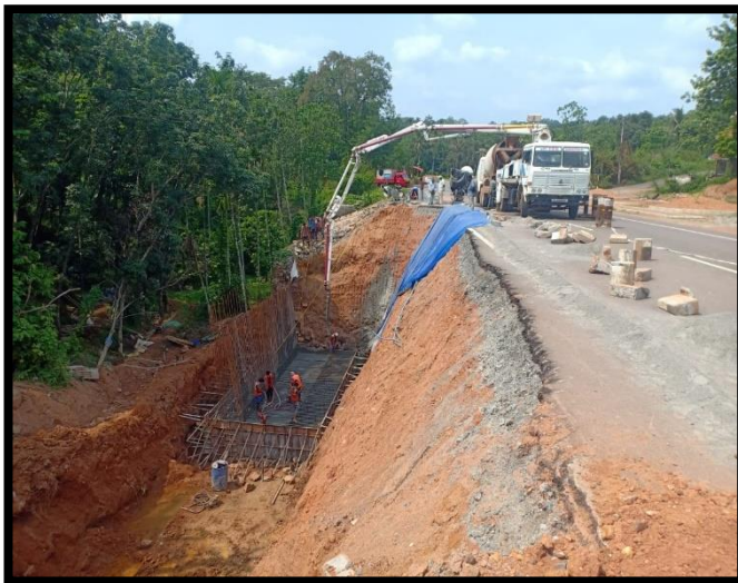
50+740 RHS retaining wall work in progress
