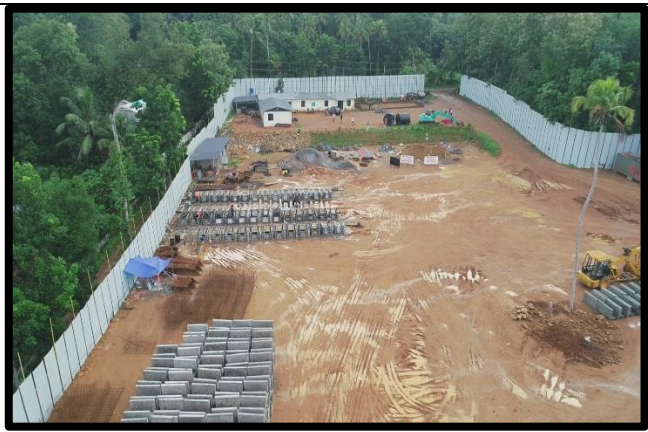
Drain Casting work in progress
