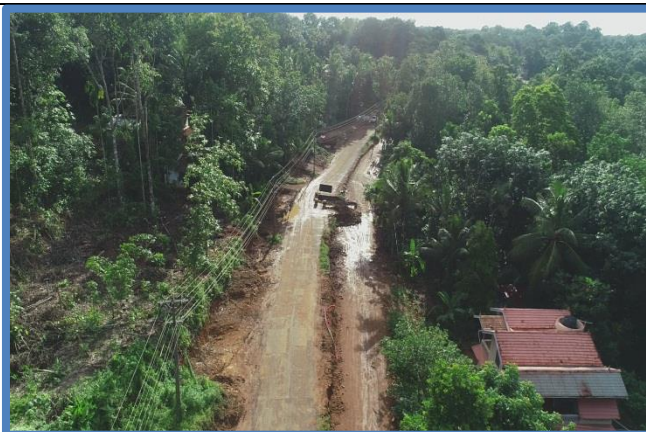
Culvert Excavation Work
