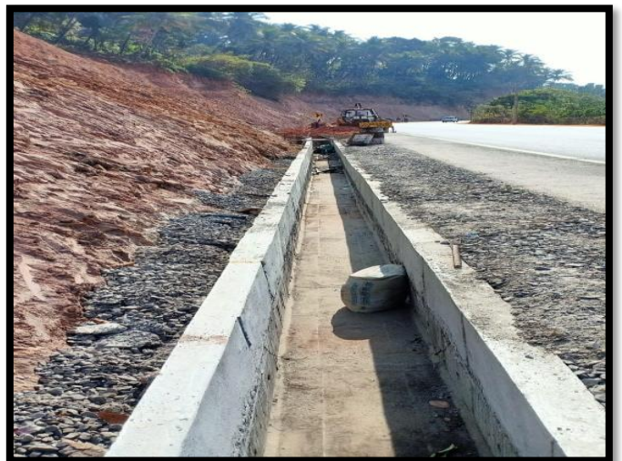
Drain work in progress.
