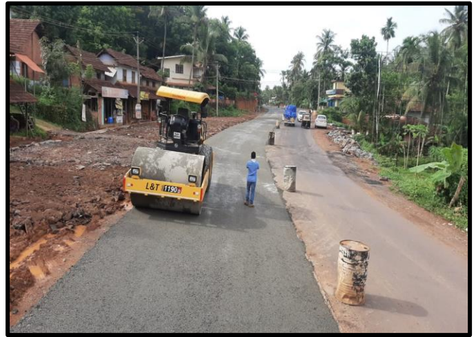
WMM 2 nd LAYER AT CH 21+700 - 21+900 LHS
