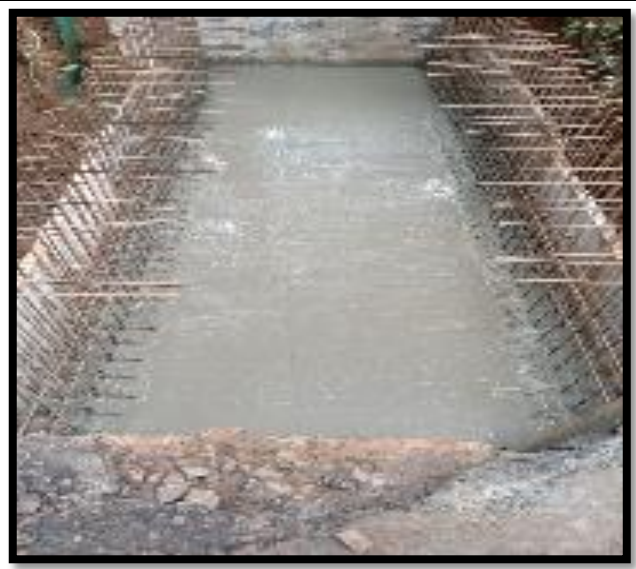
Box culvert work in Progress
