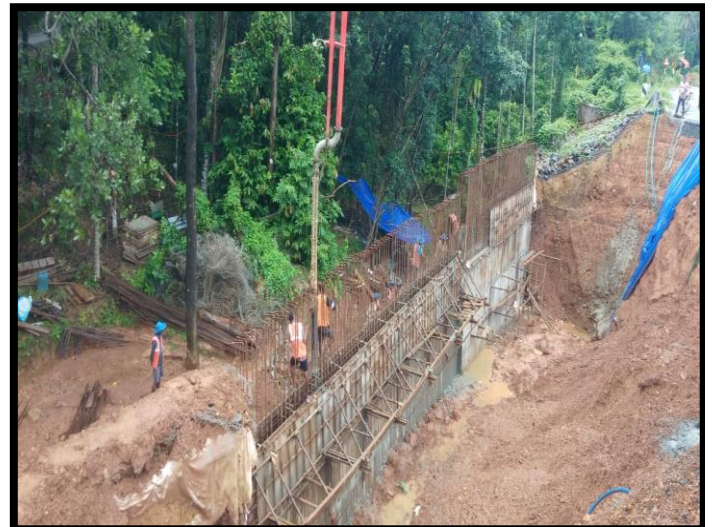
50+750 RHS retaining wall work in progress.
