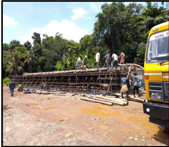
Girder Concreting, Viaduct
