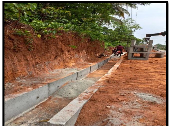
DRAIN LAYING @ 21+510LHS
