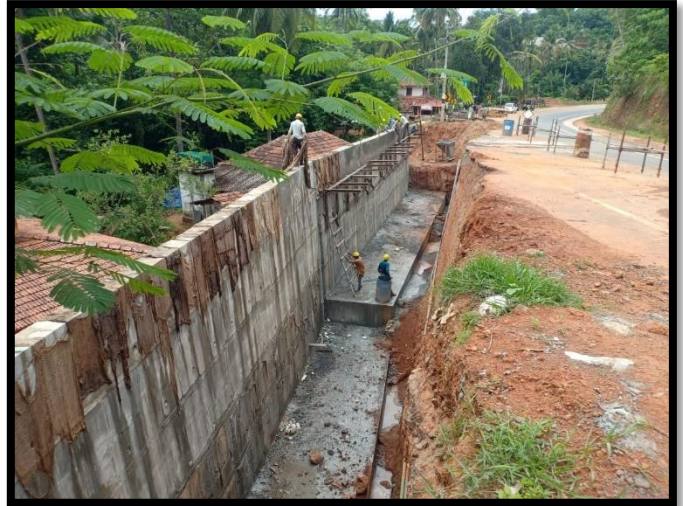
52+600 RHS retaining wall work in progress.
