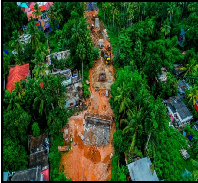
Viaduct Work, Thiruvalla Bypass
