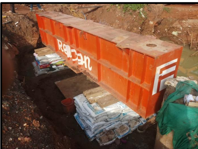
PILE LOAD TEST COMPLETED AT A2-P1 PILE KM 2+910
