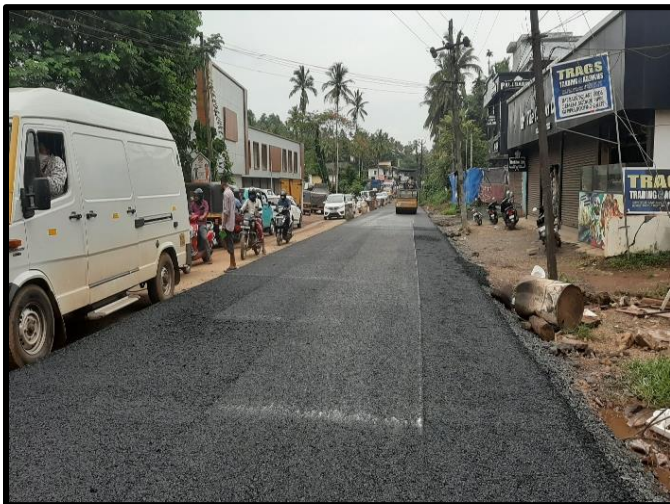
27+450 27+700 RHS DBM LAYING
