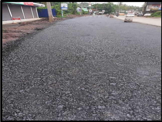
PRIME COAT AT 27+440-27+700 LHS
