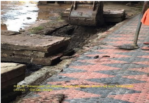
Culvert & Drain Cleaning Work in Progress
