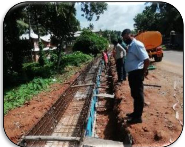
DRAIN WORK IN PROGRESS AT CH 45+350 LHS
