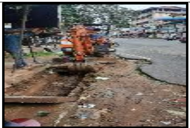
Drain Cleaning work in progress
