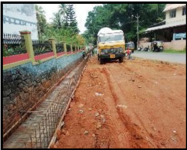
DRAIN WORK IN PROGRESS AT CH 40+100 RHS
