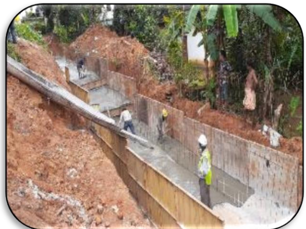
TOE WALL WORK IN PROGRESS AT CH 32+240 RHS
