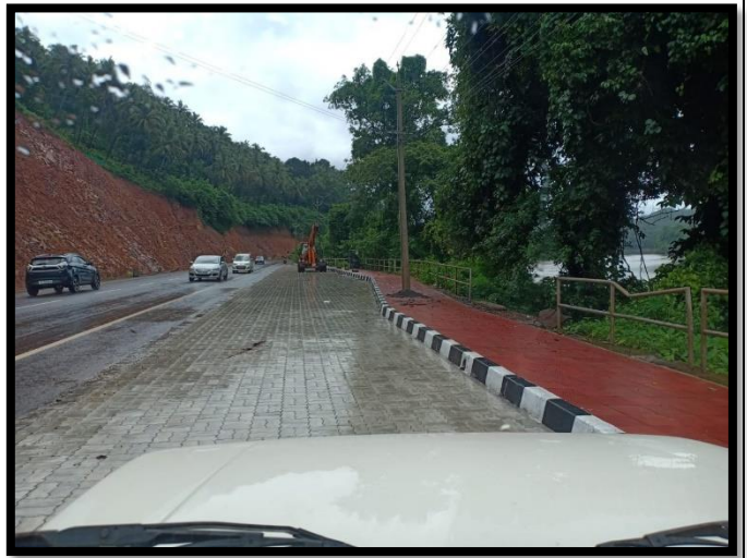
Paver block and footpath at km 42+320.
