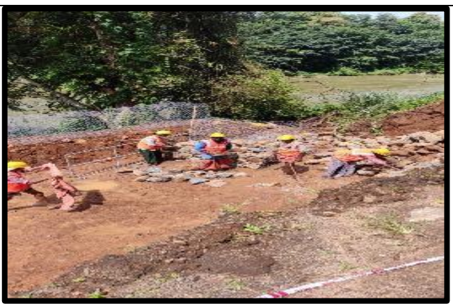
Gabion wall work in progress
