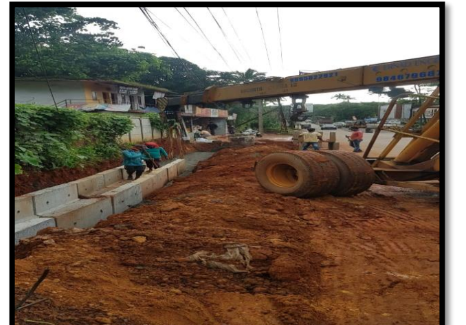
DRAIN LAYING @ 25+950-25+970 RHS
