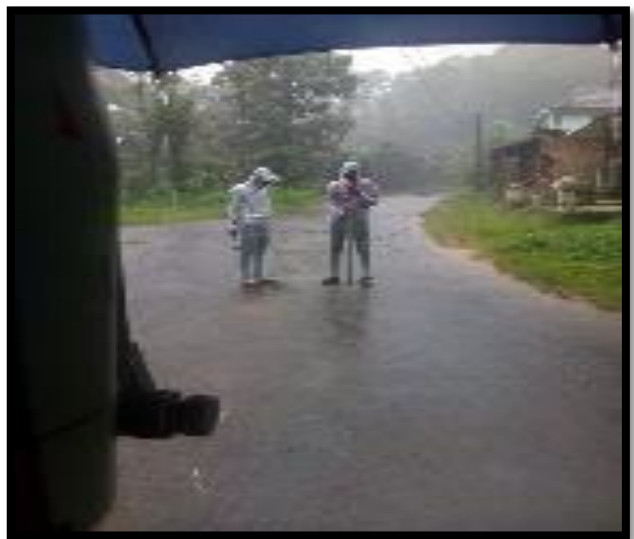
Survey work in progress
