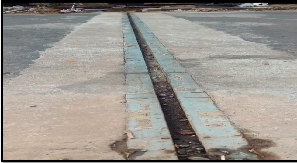
Chandrigiri Bridge Expansion Joint
