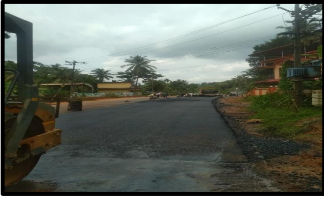
DBM LAYING @ CH 21+680-21+900 LHS
