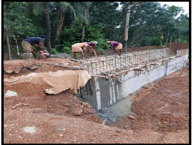
50+750 RHS RHS retaining wall work in progress.
