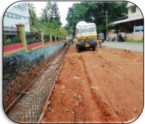
DRAIN WORK IN PROGRESS AT CH 40+100 RHS
