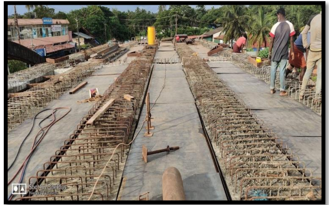
SHUTTERING WORK IN PROGRESS FOR 32m DECK SLAB @ CH 2+910 P2-P3
