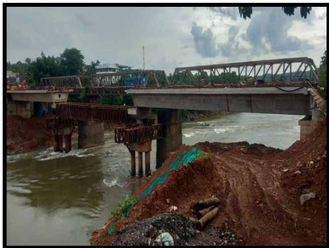
50+740 RHS retaining wall work in progress
