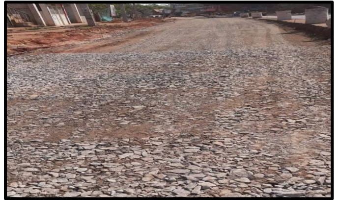
GSB LAYING @ CH 28+670 – 28+720 LHS
