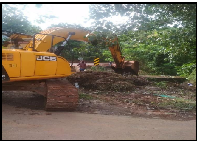
GABION WALL WORK IN PROGRESS @ CH 29+680-29+800 RHS
