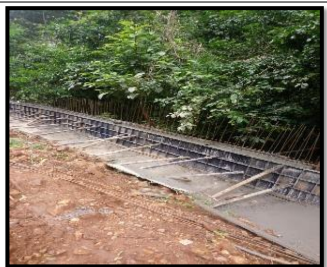
Toe wall Work in Progress
