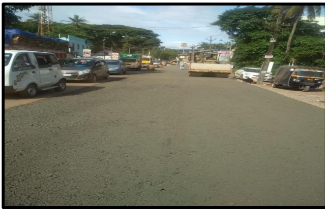
WMM 2 nd LAYER @ CH 27+270 – 27+440 RHS
