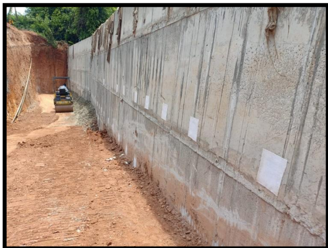
RHS retaining wall back filling work in progress
