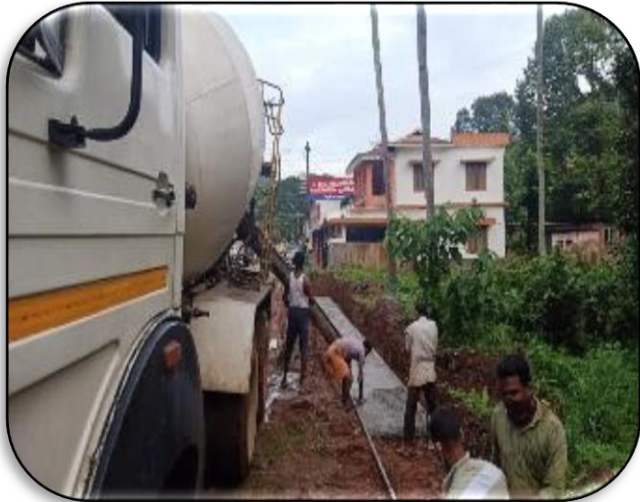
DRAIN WORK IN PROGRESS AT CH 45+350 LHS
