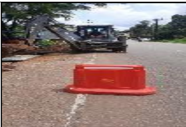
Drain Cleaning work in progress
