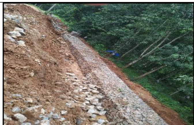
Gabion wall 1 st lift work in progress
