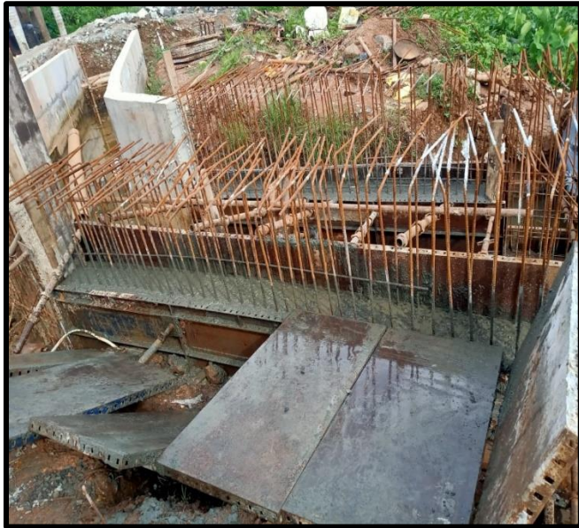
Wall concreting, Culvert widening at 2+300
