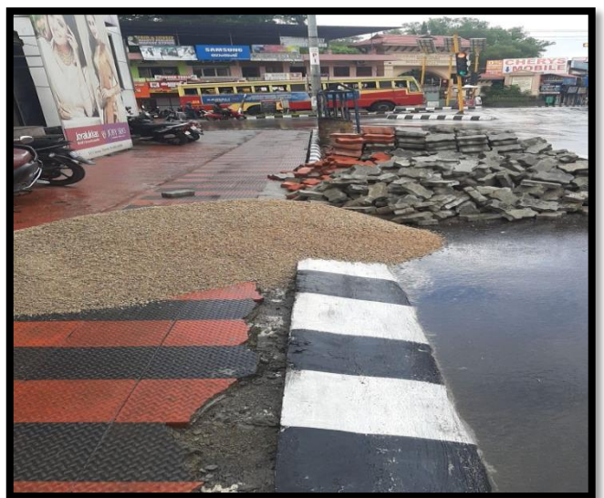
Footpath work in progress at 1+180
