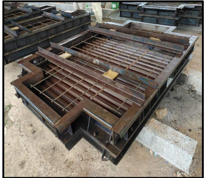
RE wall casting work at casting yard for Viaduct A2 side.
