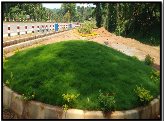
Oxbow land work in progress at km 46+850 LHS
