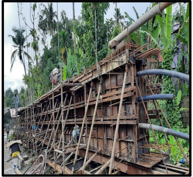
Girder concreting, Viaduct
