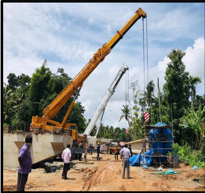
Precast Girder Erection at P8-P7, Viaduct
