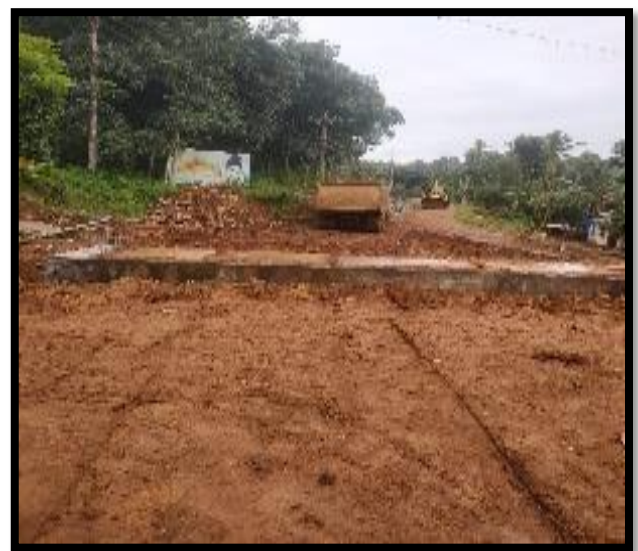
Back filling Work in progress
