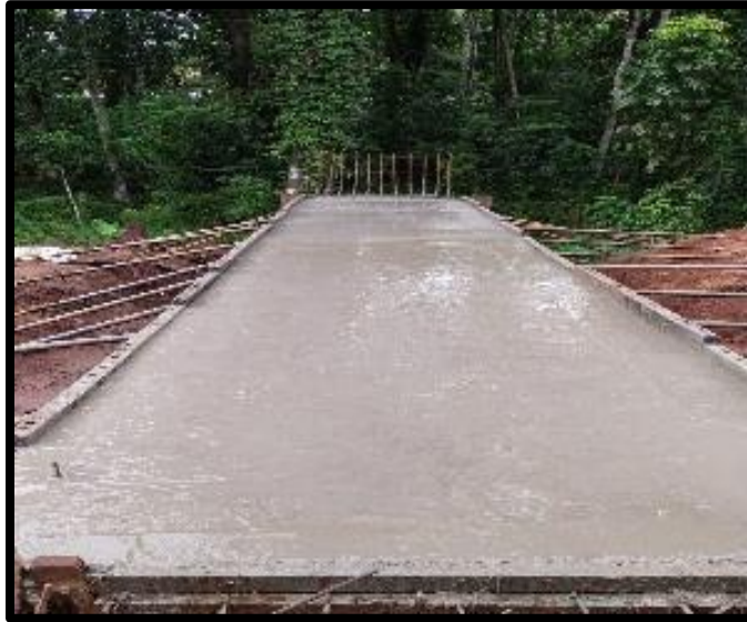
Box culvert Reinforcement work in progress
