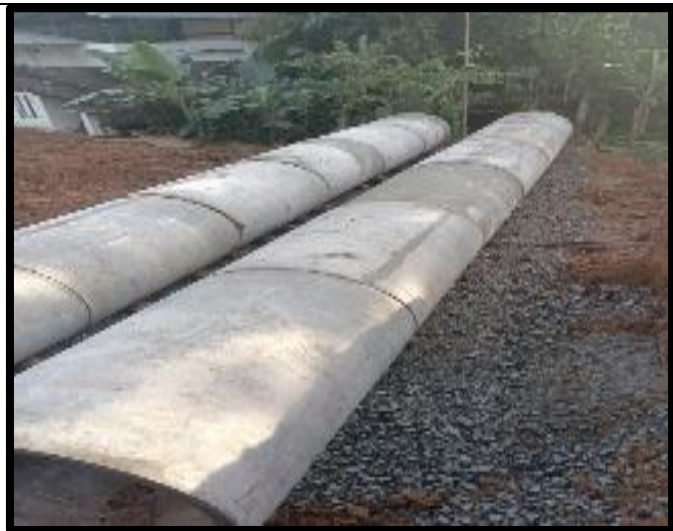
Pipe laying work
