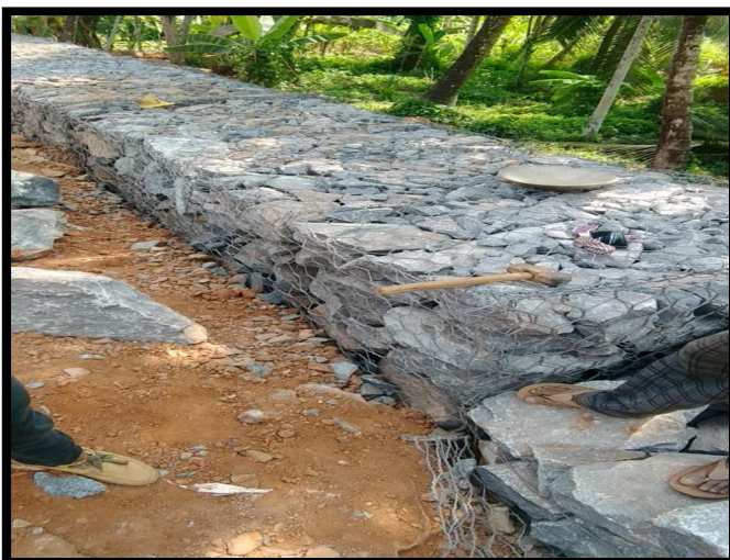
GABION IN PROGRESS AT CH 21+135-21+180 RHS
