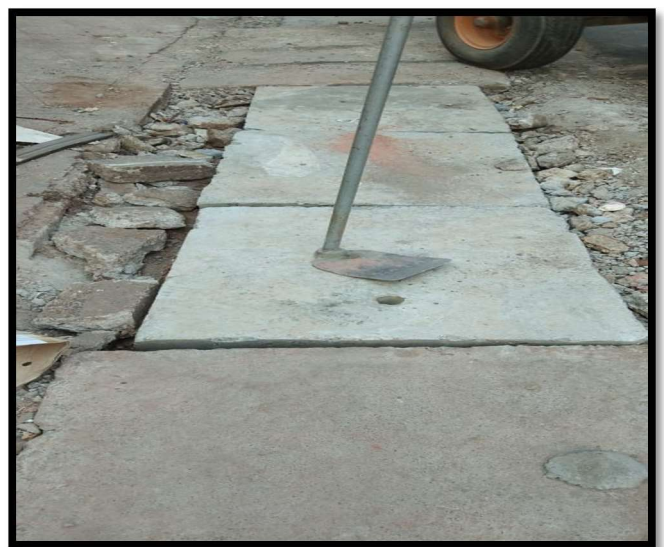
Coverslab fixing work
