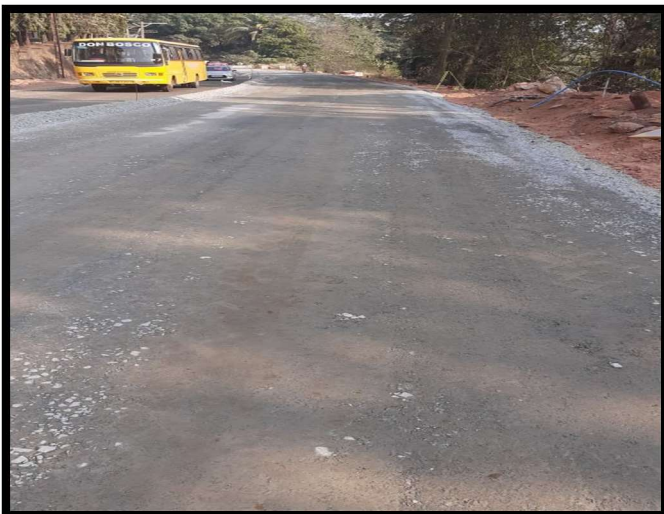
GSB in progress A2 side approach of Irritty Bridge
