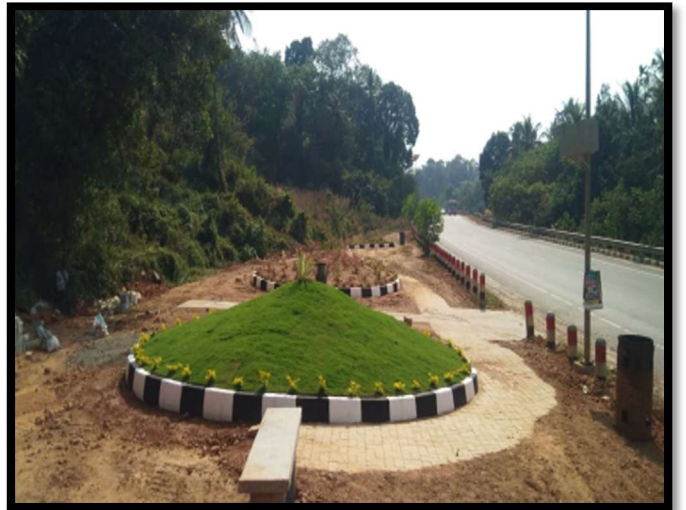
• Oxbow land at 39+350 RHS.
