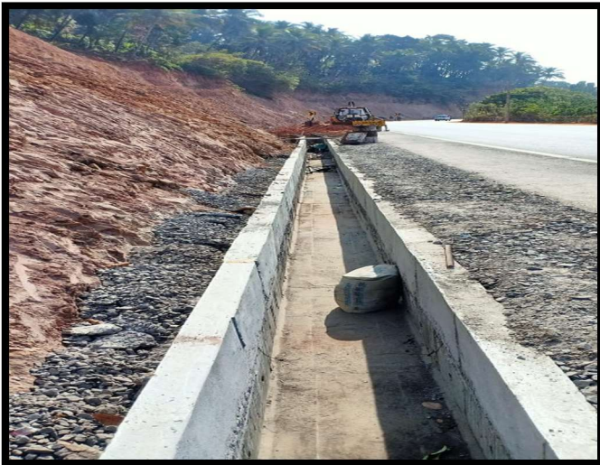
• Drain Work in progress 2 A2 side approach of Irritty bridge.
