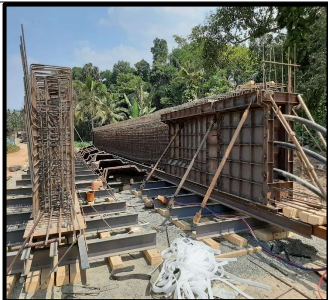
Girder shuttering work, Viaduct
