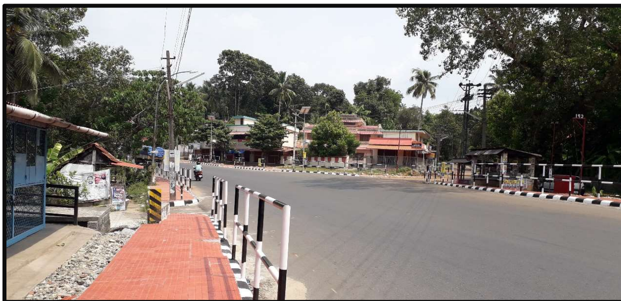
Railing at Footpath
