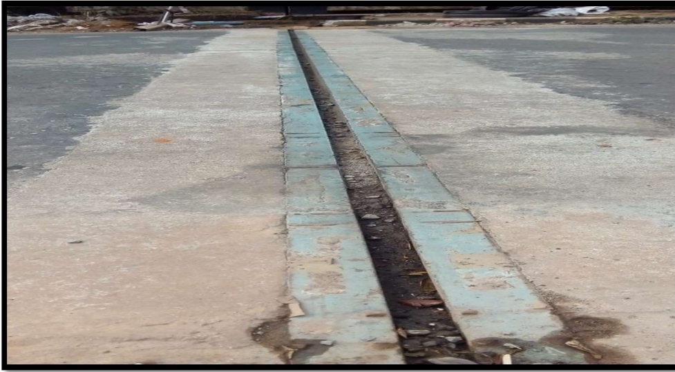
Chandrigiri Bridge Expnasion Joint
