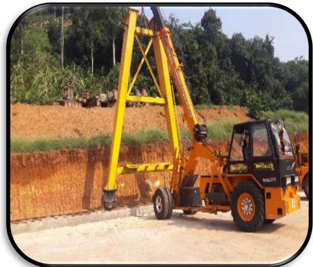
Casting yard preparation under progress
