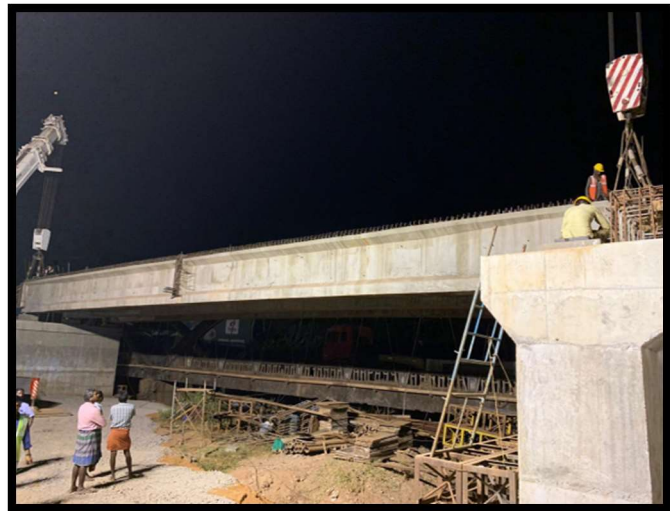
GIRDER LAUNCHING COMPLETED Between PIER P2-P3 @ Km 2+910
