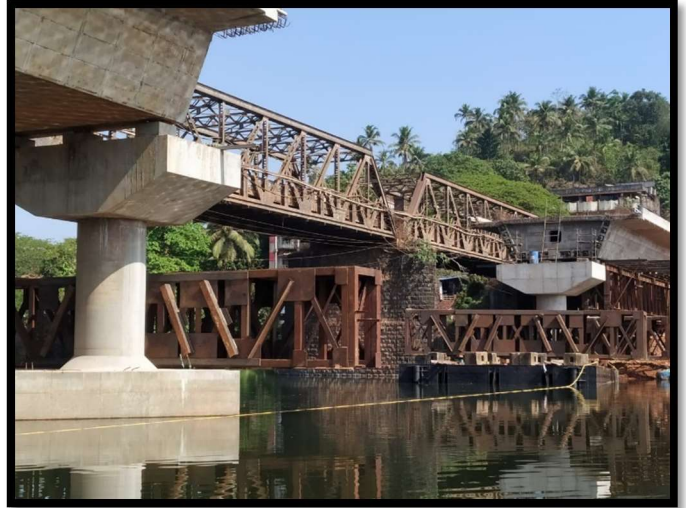
Irritty Bridge work is in progress
