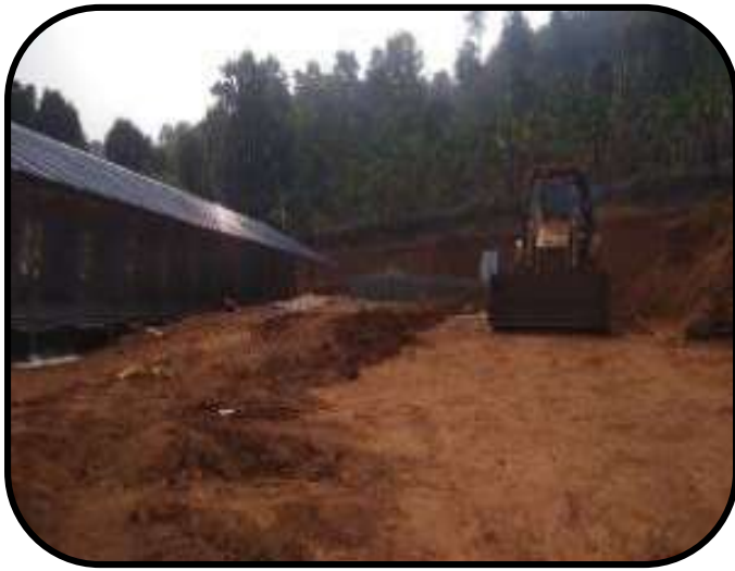
Staff quarters are in process
