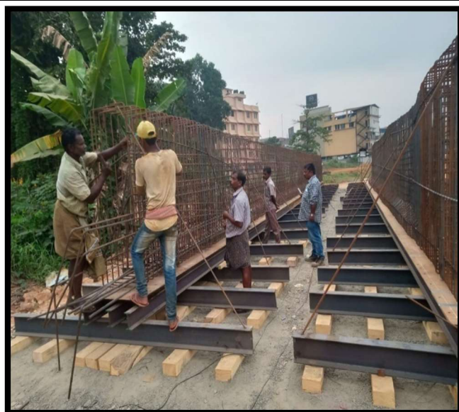
Girder reinforcement work, Viaduct
