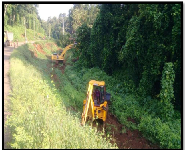
Embankment Filling work in Progress
