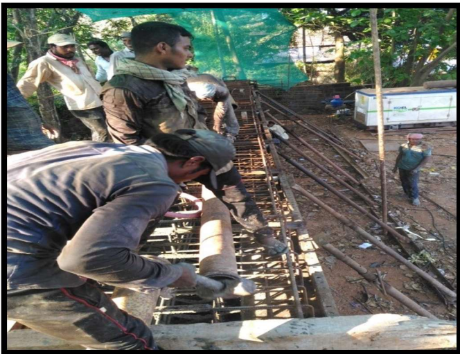
GIRDER CASTING @ CH 2+910
