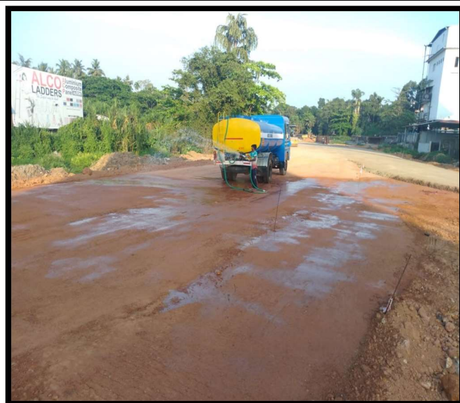
Subgrade work from Km:2+150 to km:2+200
