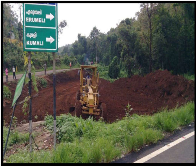
Embankment Filling work in Progress @ CH: 60+400 – 60+450
