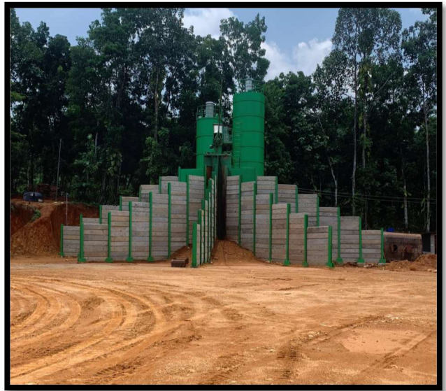
RMC Plant erection work Completed
