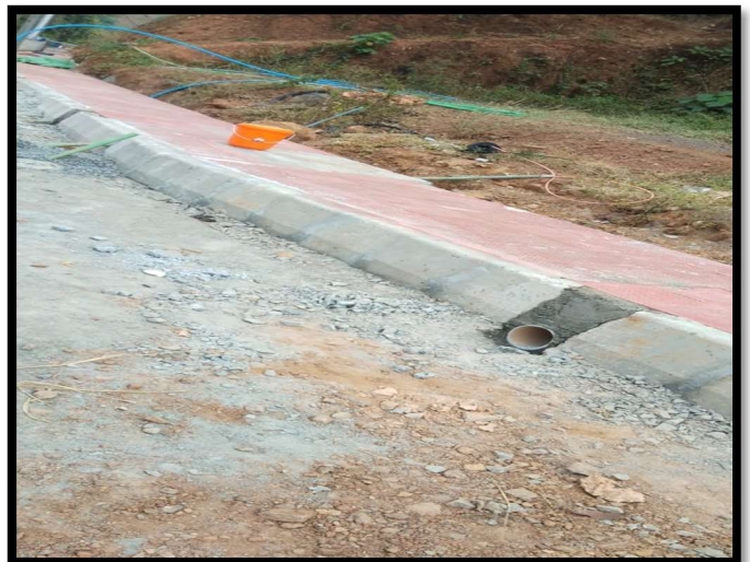
• Footpath work in progress.
