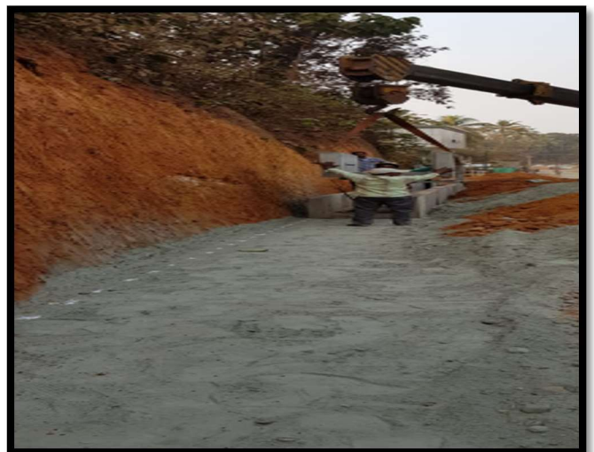
DRAIN LAYING @ 21+430LHS
