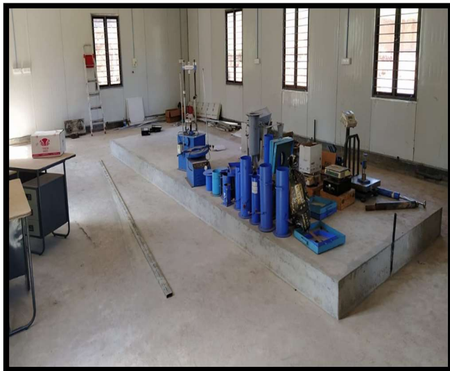
Laboratory construction completed and equipment fixing in progress
