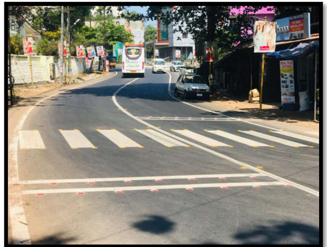
Road Marking works completed at BC completed areas
