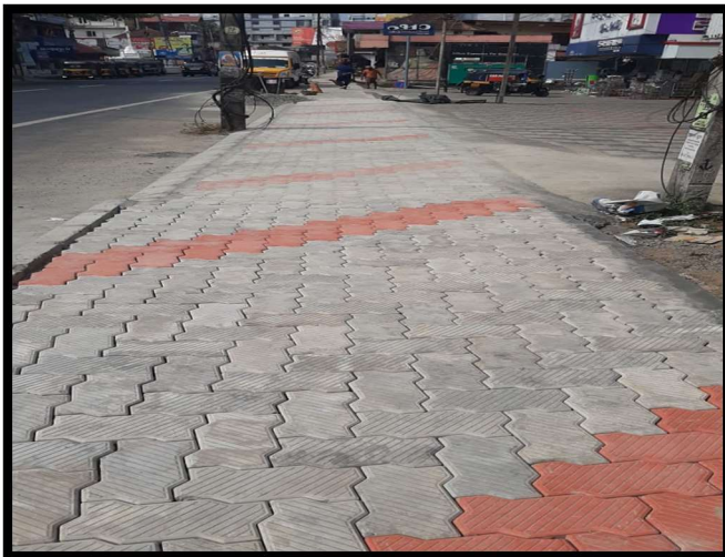
Footpath Laying work
