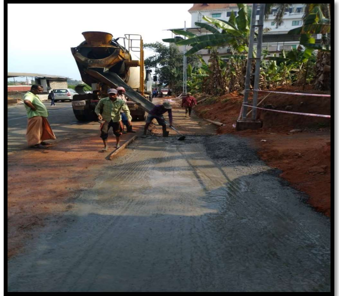
V drain concreting work at 1+450 LHS
