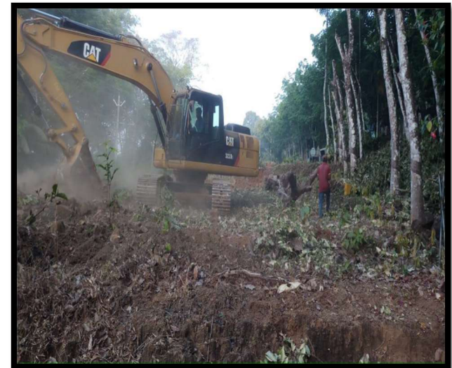
C & G Work in Progress
