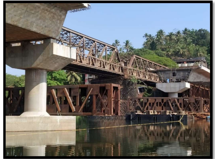
Iritty Bridge work is in progress
