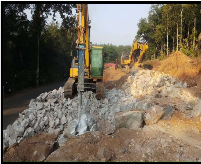
Rock breaking work in progress
