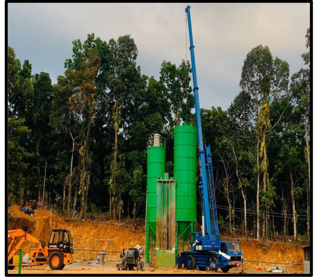
RMC Plant erection work in progress
