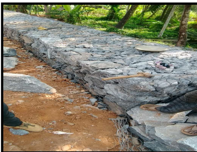
GABION IN PROGRESS AT CH 21+135-21+180 RHS
