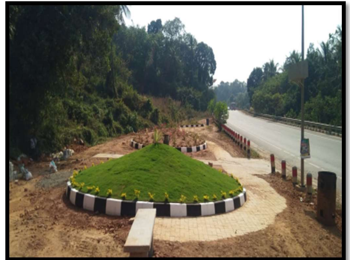
• Oxbow land at 39+350 RHS.
