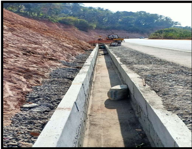
• Drain Work in progress 2 A2 side approach of Iritty bridge.
