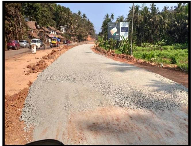
GSB IN PROGRESS AT 21+710 – 21+790 RHS
