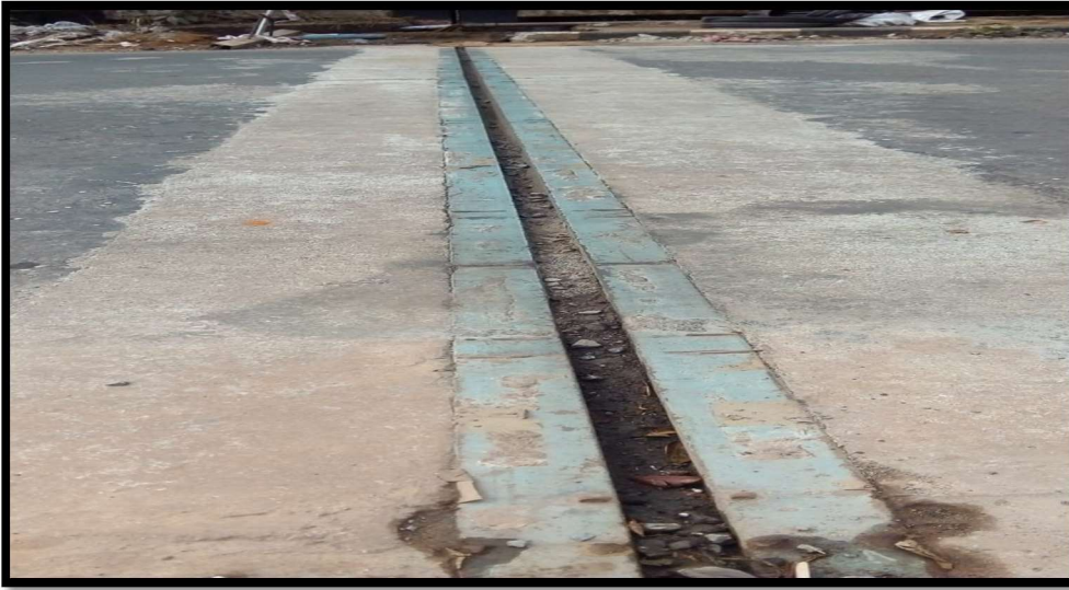
Chandrigiri Bridge Expnsion Joint
