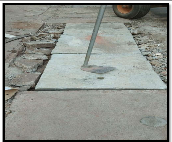
Coverslab fixing work
