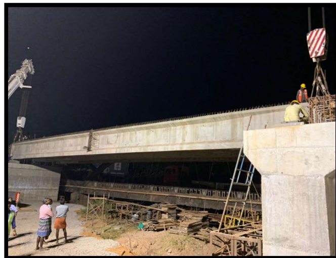
GIRDER LAUNCHING COMPLETED Between PIER P2-P3 @ Km 2+910
