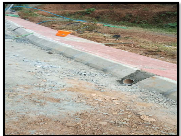
• Footpath work in progress.
