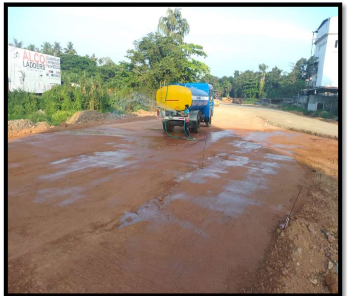
Subgrade work from Km:2+150 to km:2+200
