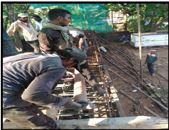
GIRDER CASTING @ CH 2+910
