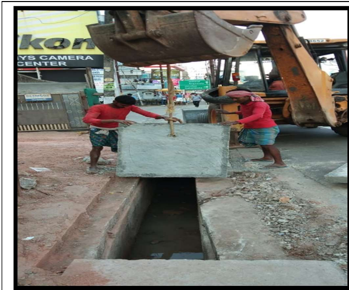
Coverslab fixing work
