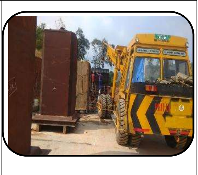
Culvert moulds preparing in progress
