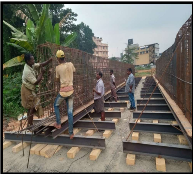
Girder reinforcement work, Viaduct
