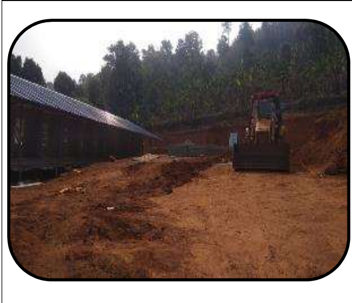
Staff quarters are in process
