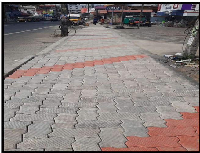
Footpath Laying work
