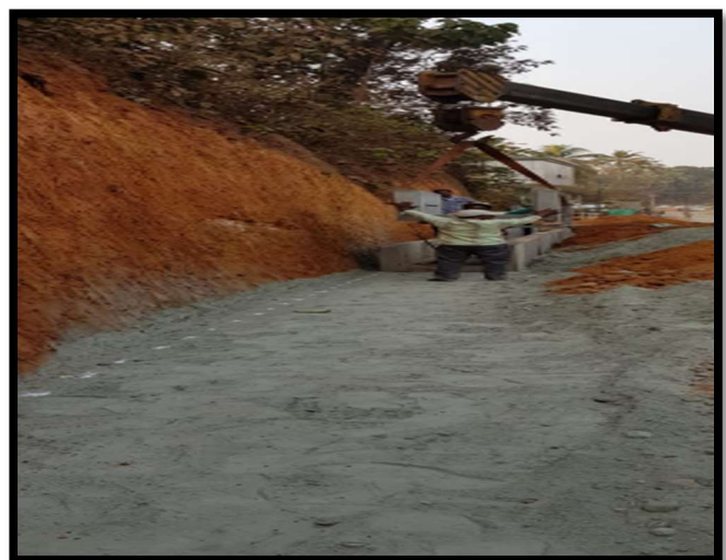
DRAIN LAYING @ 21+430LHS
