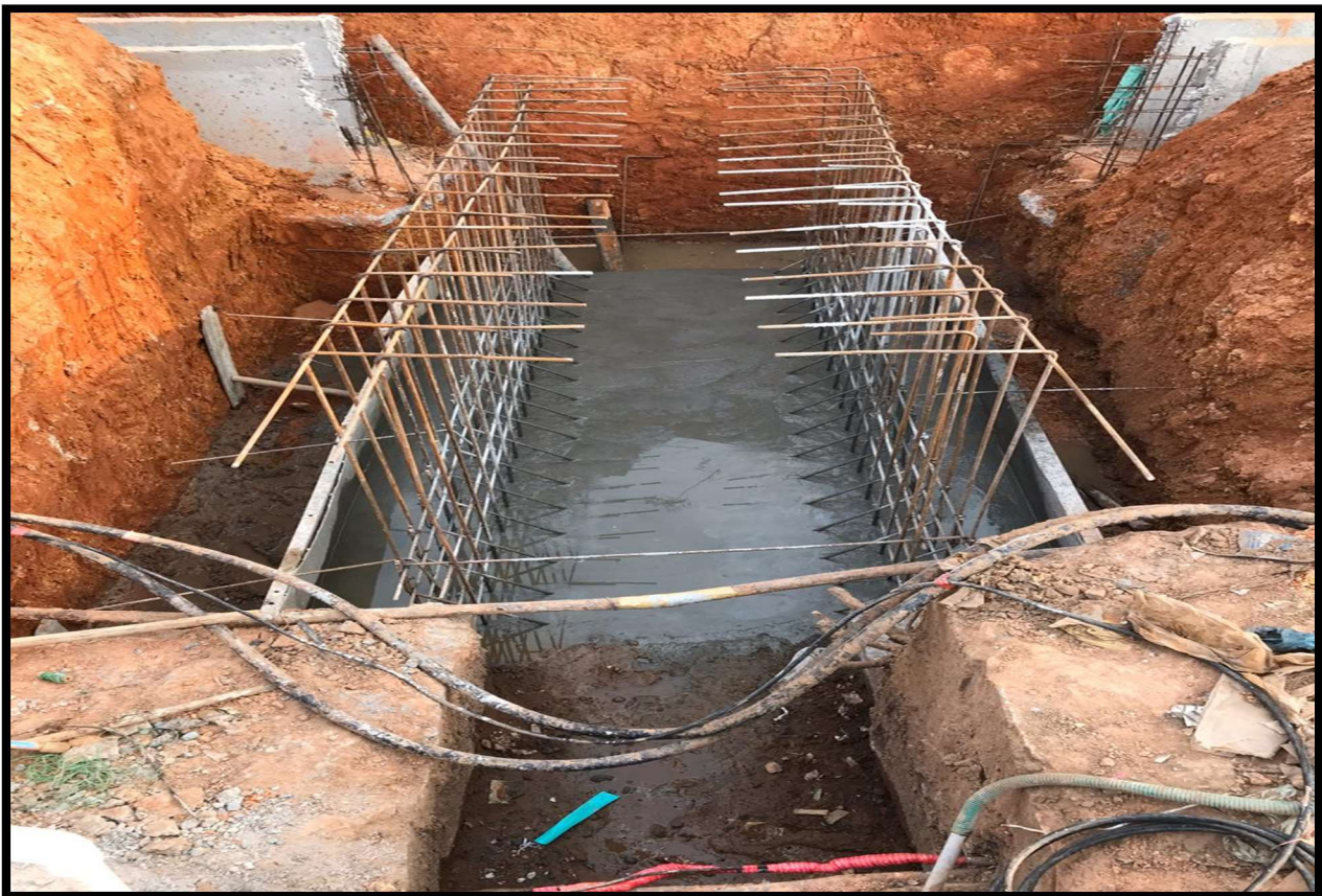
Culvert extension @ Adoor
