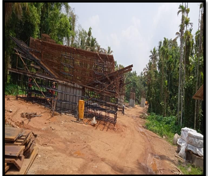
Reinforcement work for Viaduct.
