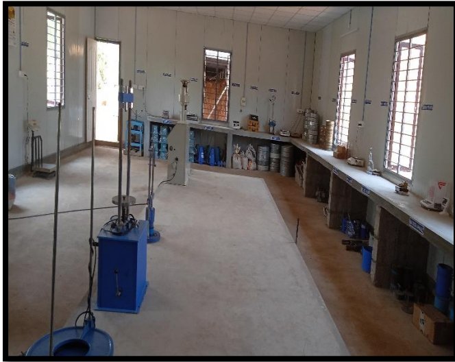
Site Laboratory construction work is in progress
