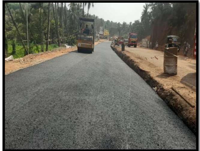
DBM @ CH: 21+230 to 21+350 RHS
