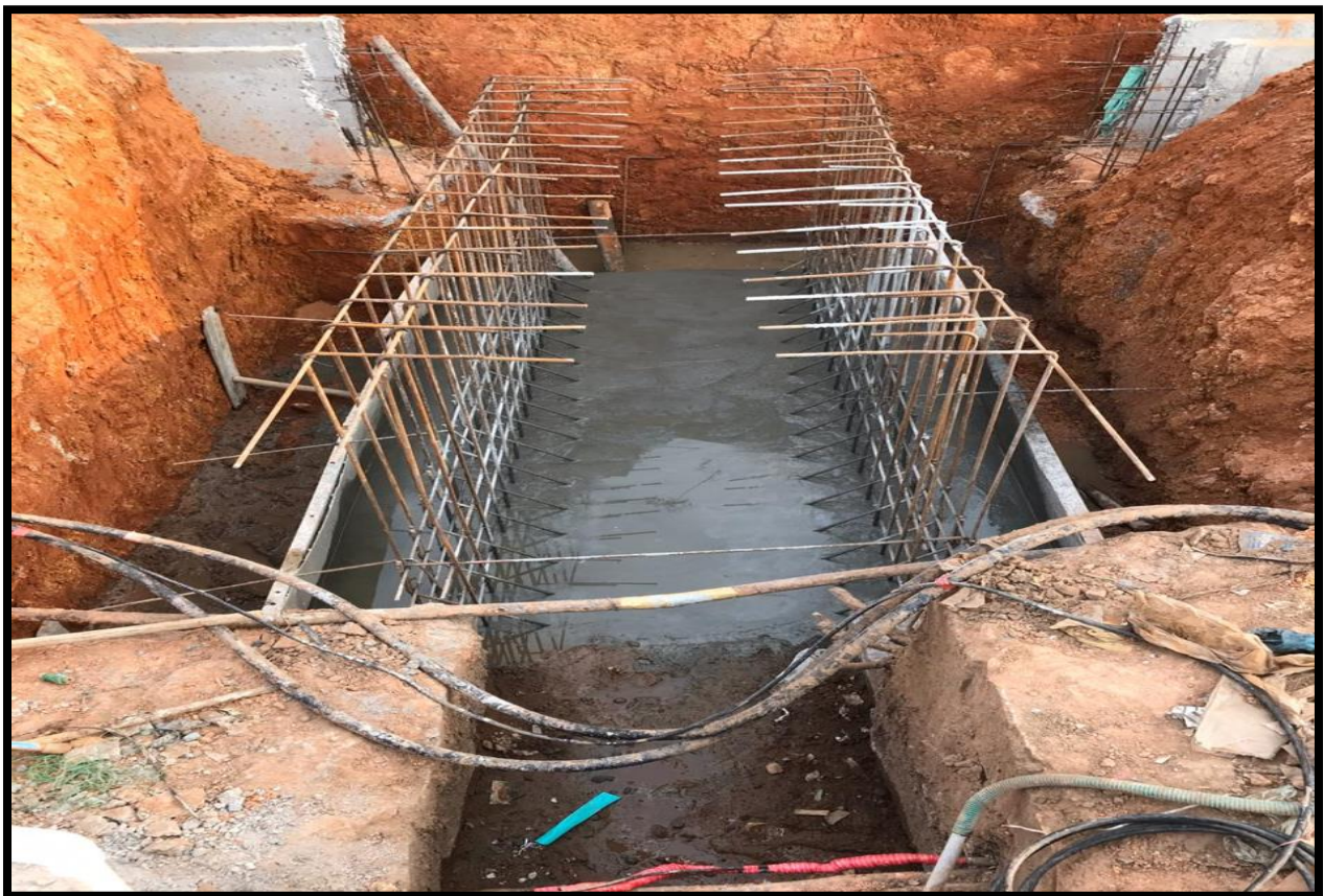
Culvert extension @ Adoor
