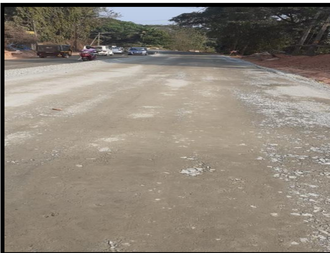
GSB in progress A2 side approach of Iritty Bridge
