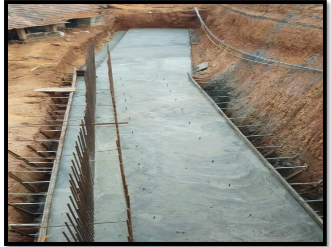
Footpath & Hand rail work is in progress
