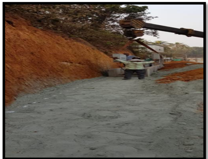
DRAIN LAYING @ 21+430 LHS
