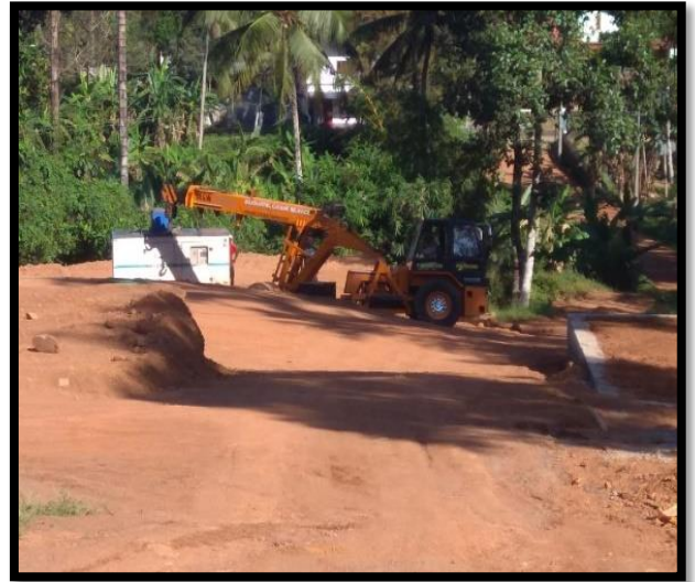
Base camp construction is in progress
