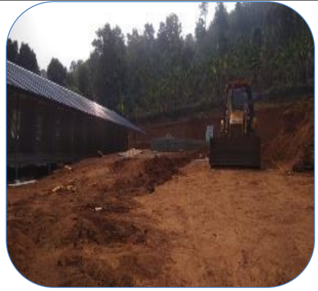
Staff Quarter in progress
