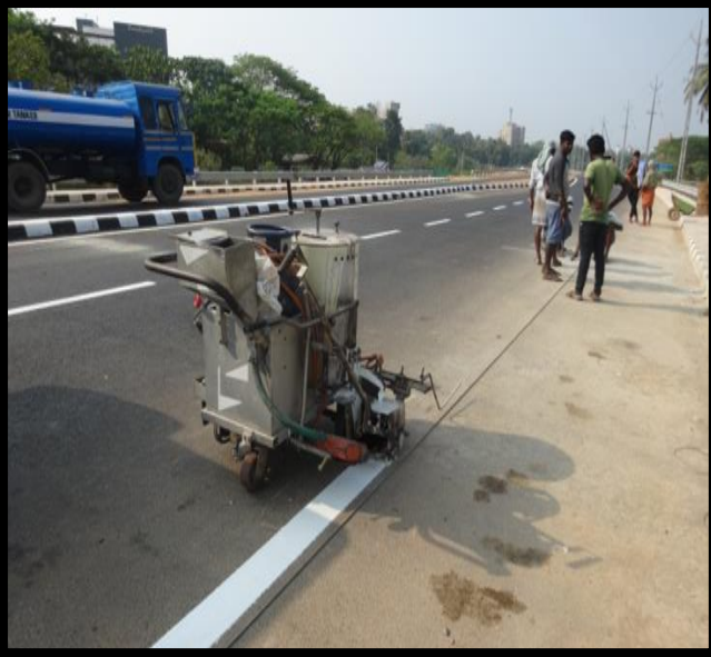
Road Marking work in progress.
