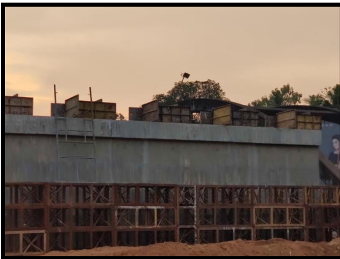
PEDESTAL CONCRETING @ CH: 2+910
