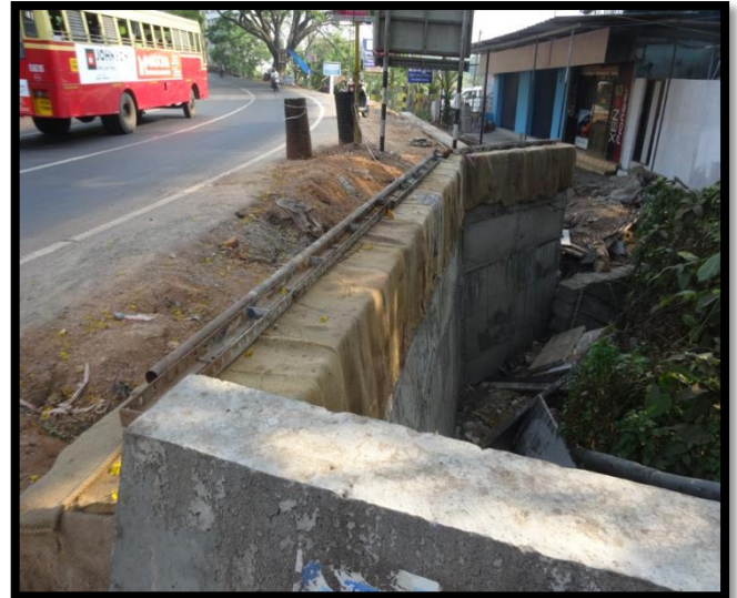
Culvert extension work in progress at Rejinamundi culvert.
