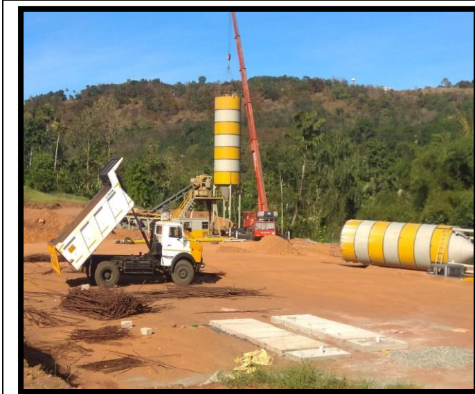
Plant Erection in progress
