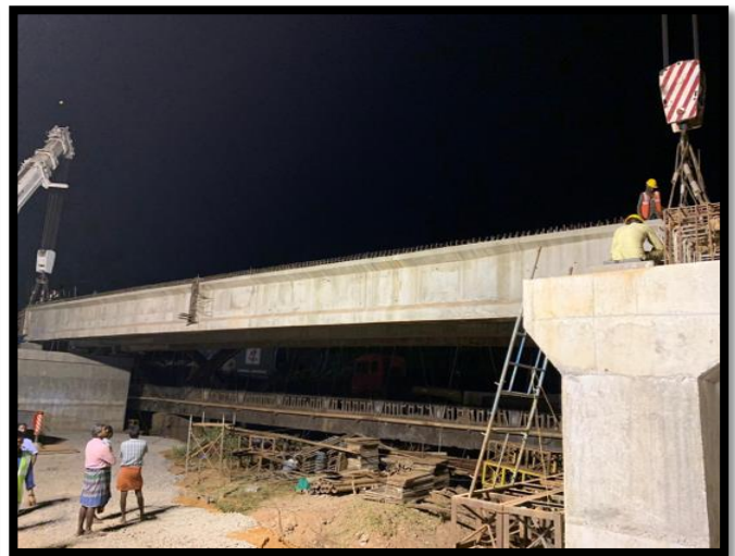
GIRDER LAUNCHING COMPLETED Between PIER P2-P3 @ Km 2+910
