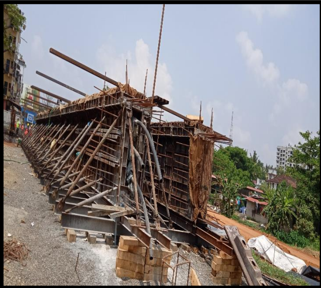
Casting of PSC Girder at Viaduct work
