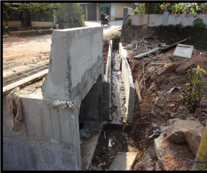
Crash barrier and drain work at 7+640, Rejinamundi Culvert
