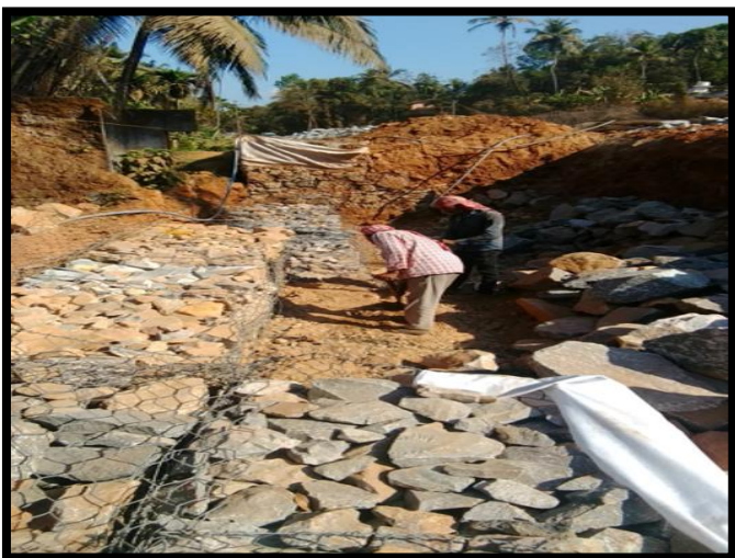
GABION WORK IN PROGRESS AT CH: 21+370 RHS
