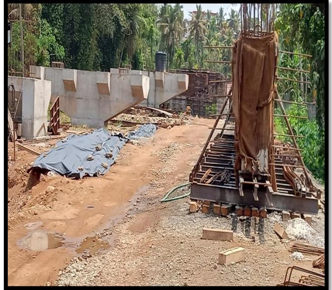
Pier Concrete work
